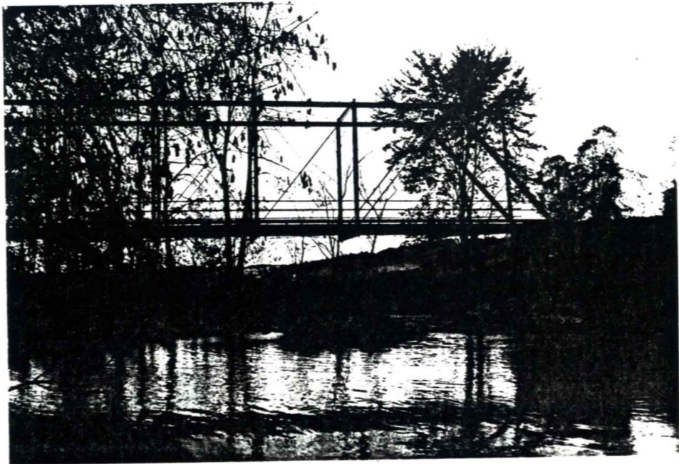
3.50 Pearl Creek, N.Y., Crossman Road, Catka Creek, Pratt through truss, 1879, potential NR, elevation.
