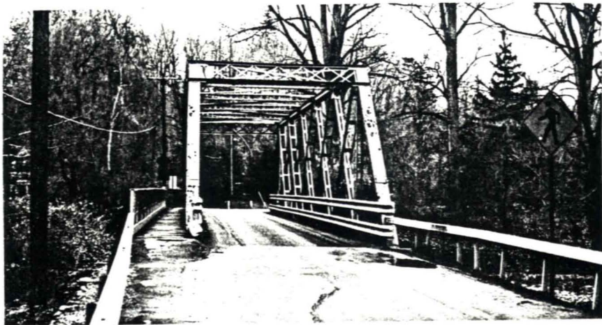
3.33 Ithaca, N.Y., Forest Home Drive, Fall Creek, Warren Double Intersection through truss, 1909, portal.
