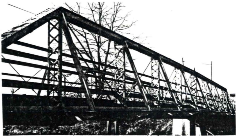
3.8 Dryden, N.Y., Red Mill Road, Fall Creek, 2 span Pratt pony truss, 1887, outriggers.
