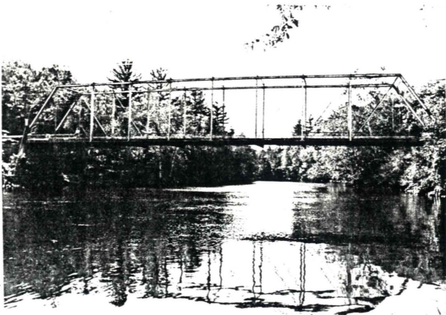
3.59 Schuyler Falls, N.Y., Goddeau Road, Saranac River, Pratt through truss, 1900, elevation.
