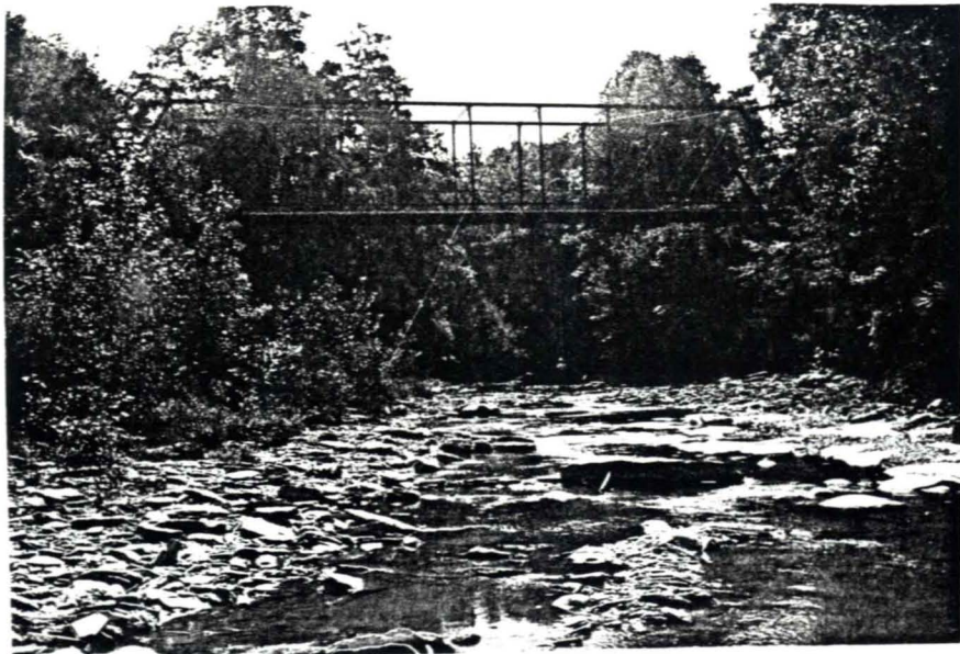
3.54 Westfield, N.Y., South Water Street, Chatauqua Creek, Pratt through truss, n.d., elevation.
