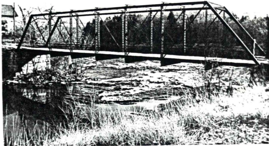
3.68 Gouverneur, N.Y., Lockie Road, Oswegatchie River, Pratt through truss, 1885, elevation.
