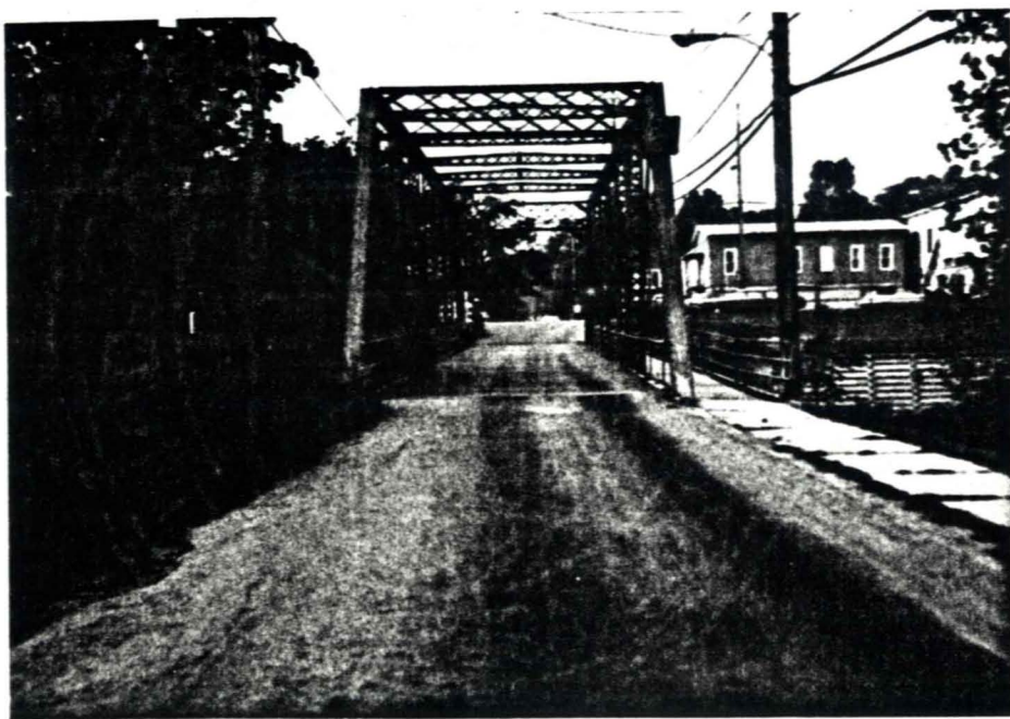
3.46 Landers Corners, N.Y., Otselic River, Pratt through truss, 1890, portal.
