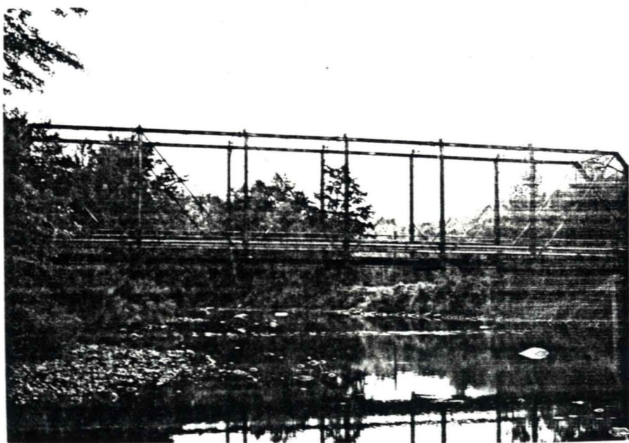
3.40 Keene, N.Y., South Lacy Road, East Branch Ausable River, Pratt through truss, 1895, longitudinal view.
