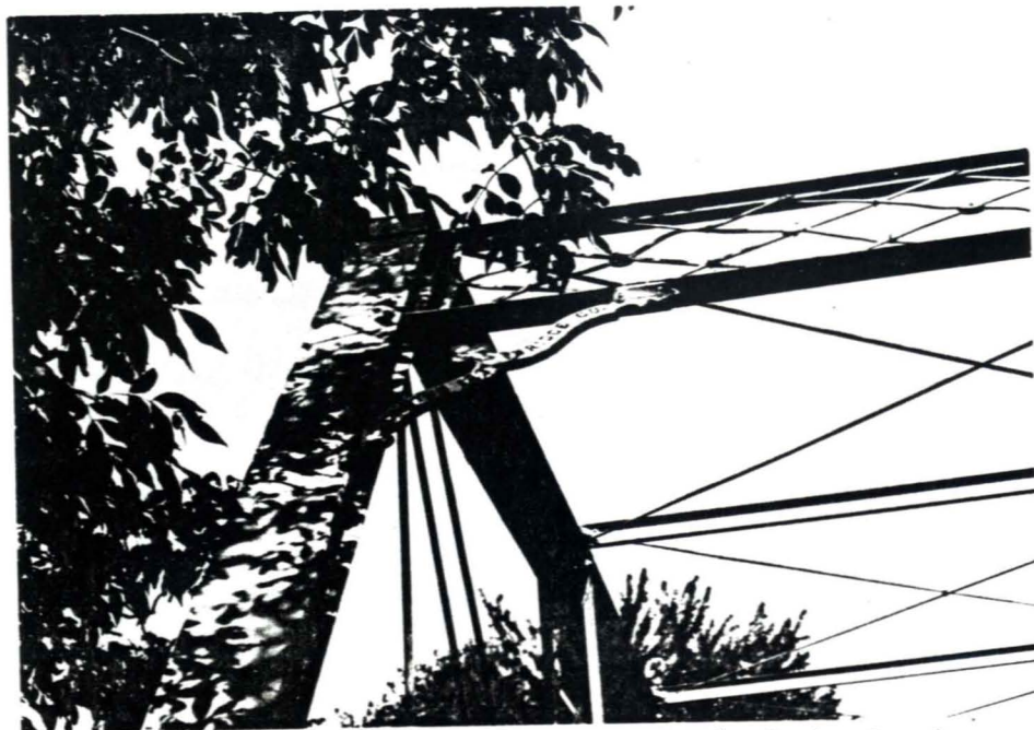
3.52 Pearl Creek, N.Y., Crossman Road, Catka Creek, Pratt through truss, 1879, potential NR, knee bracing.
