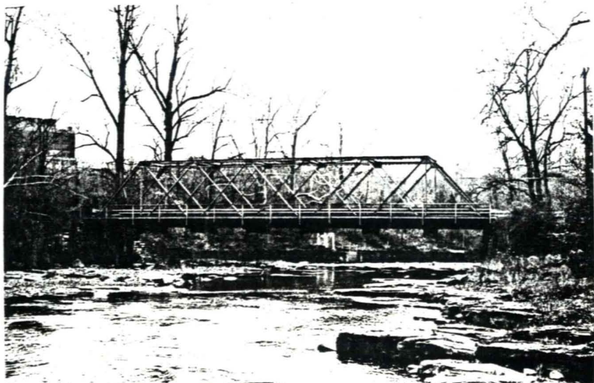
3.32 Ithaca, N.Y., Forest Home Drive, Fall Creek, Warren Double Intersection through truss, 1909, elevation.
