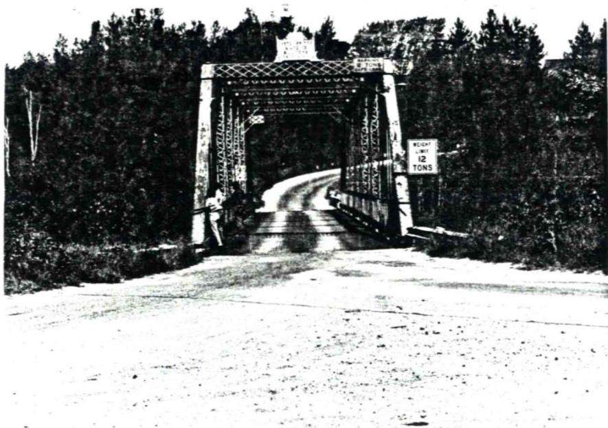
3.63 Saranac, N.Y., Ore Bed Road, Saranac River, Pratt through truss, 1898, approach.
