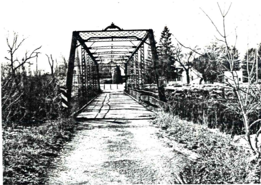
3.69 Gouverneur N.Y., Lockie Road, Oswegatchie River, Pratt through truss, 1885, portal.
