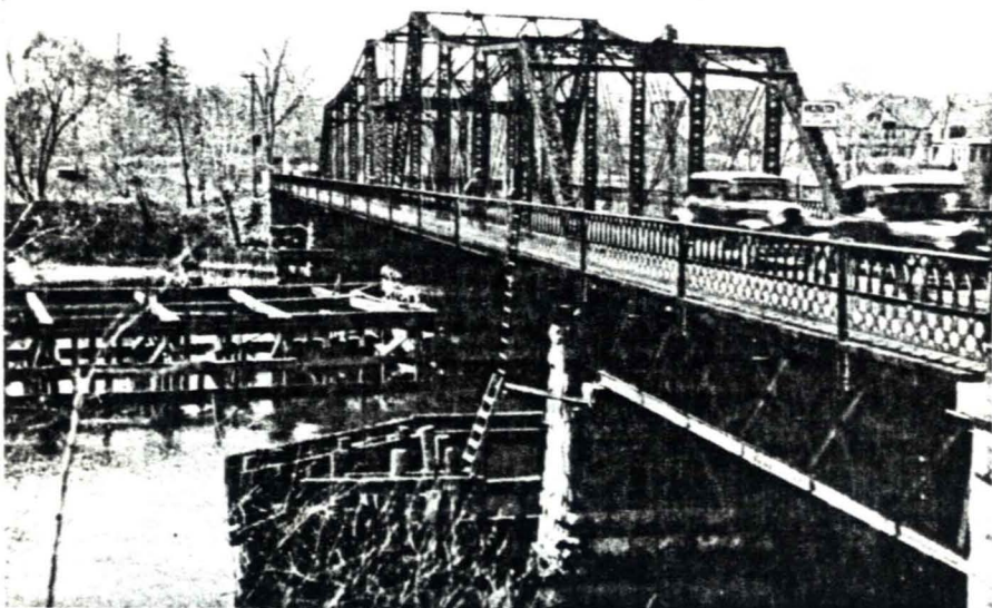
3.29 Rutherford, N.J., Union Avenue, Passaic River, swing bridge, 1896, historic longitudinal view.
