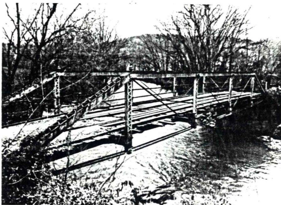
3.28 New Middleton, Tenn., Bradford Hill Road, Mulhervin Creek, 1901, demolished.
