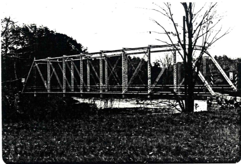
3.70 Wegatchie, N.Y., Kearney Road, Oswegatchie River, Pratt through truss, 1886, potential NR, elevation.
