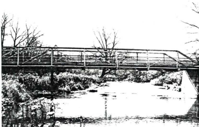
3.7 Dryden, N.Y., Red Mill Road, Fall Creek, 2 span Pratt pony truss, 1887, longitudinal view showing pier.
