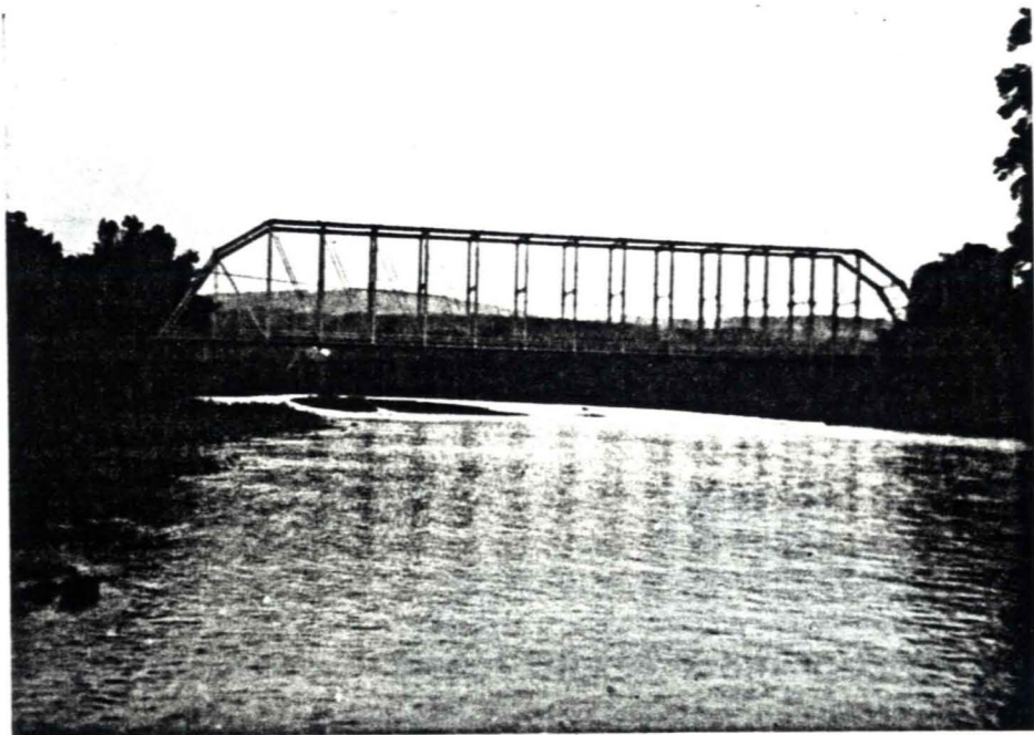
3.58 Caneadea, N.Y., East Hill Road, Genesee River, Camelback truss, 1903, elevation.
