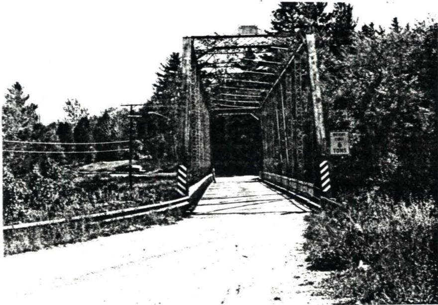
3.60 Schuyler Falls, N.Y., Goddeau Road, Saranac River, Pratt through truss, 1900, approach.
