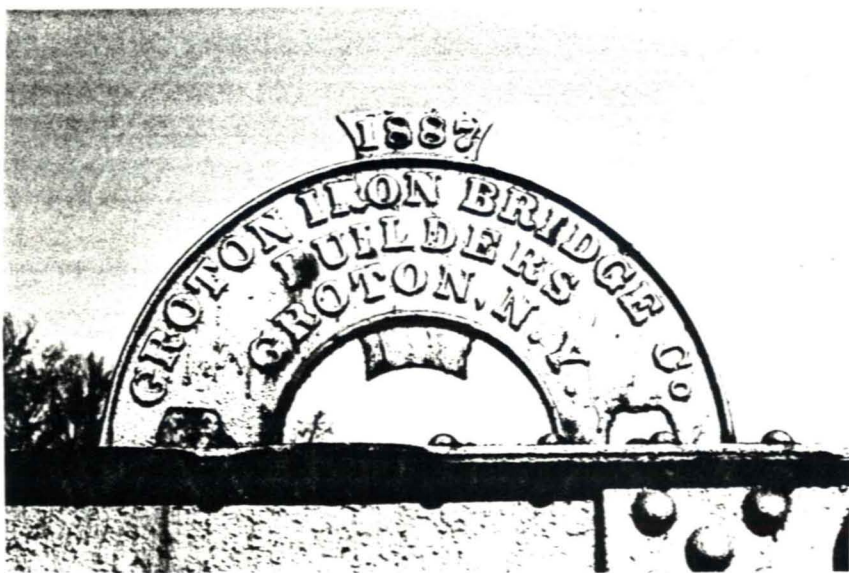
3.10 Dryden, N.Y., Red Mill Road, Fall Creek, 2 span Pratt pony truss, 1887, bridgeplate.
