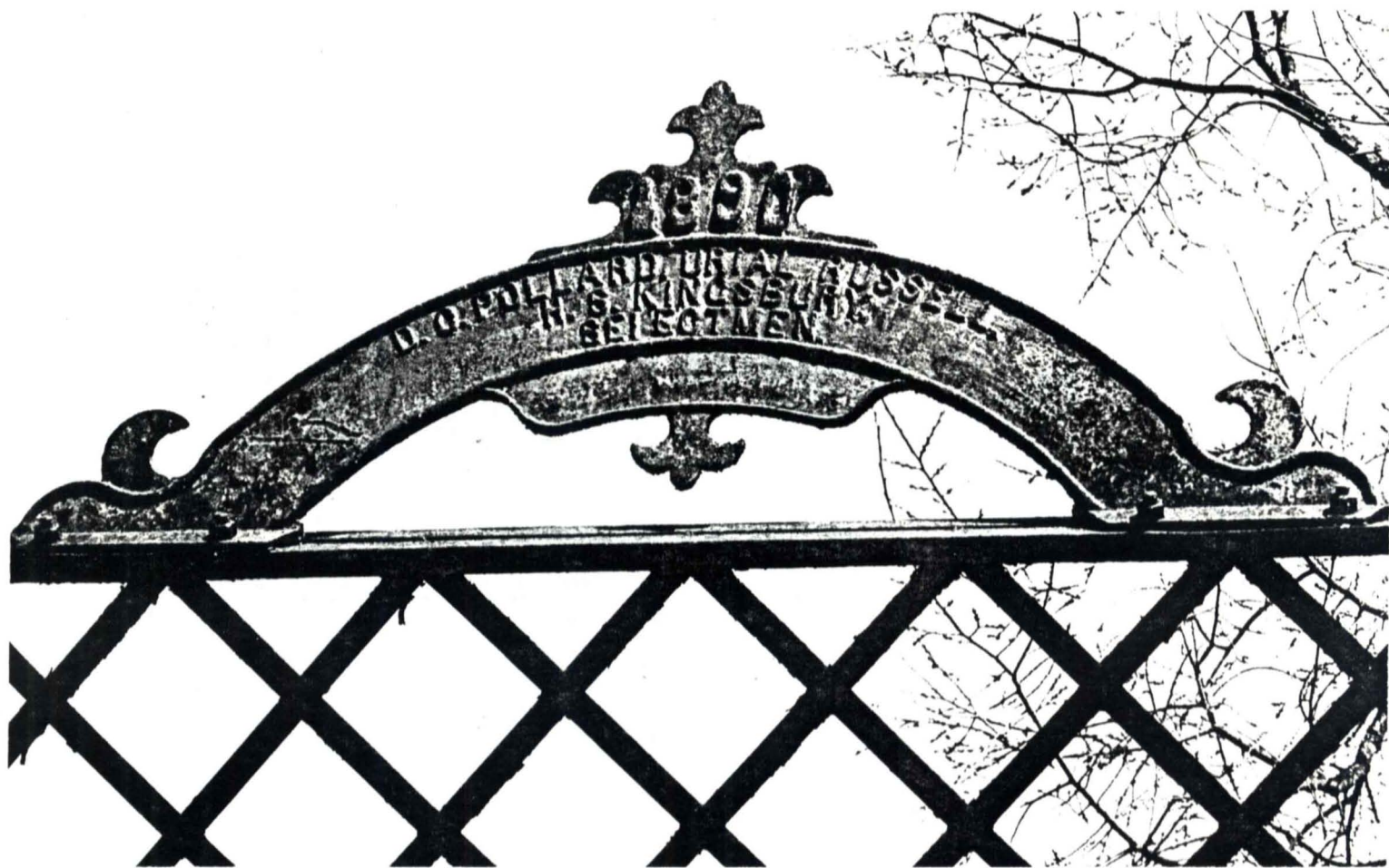
3.23 Cavendish, Vt., Howard Hill Road, Black River, Pratt through truss, 1890, NR, bridgeplate.
