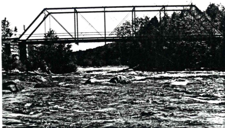
3.62 Saranac, N.Y., Ore Bed Road, Saranac River, Pratt through truss, 1898, elevation.
