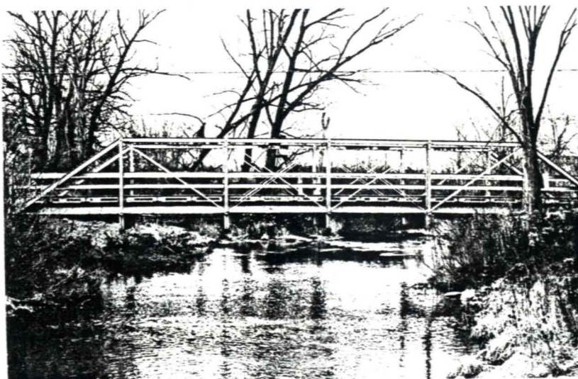
3.2 Ithaca, N.Y., German Cross Roads, Six Mile Creek, Pratt pony truss, 1877, elevation, demolished.
