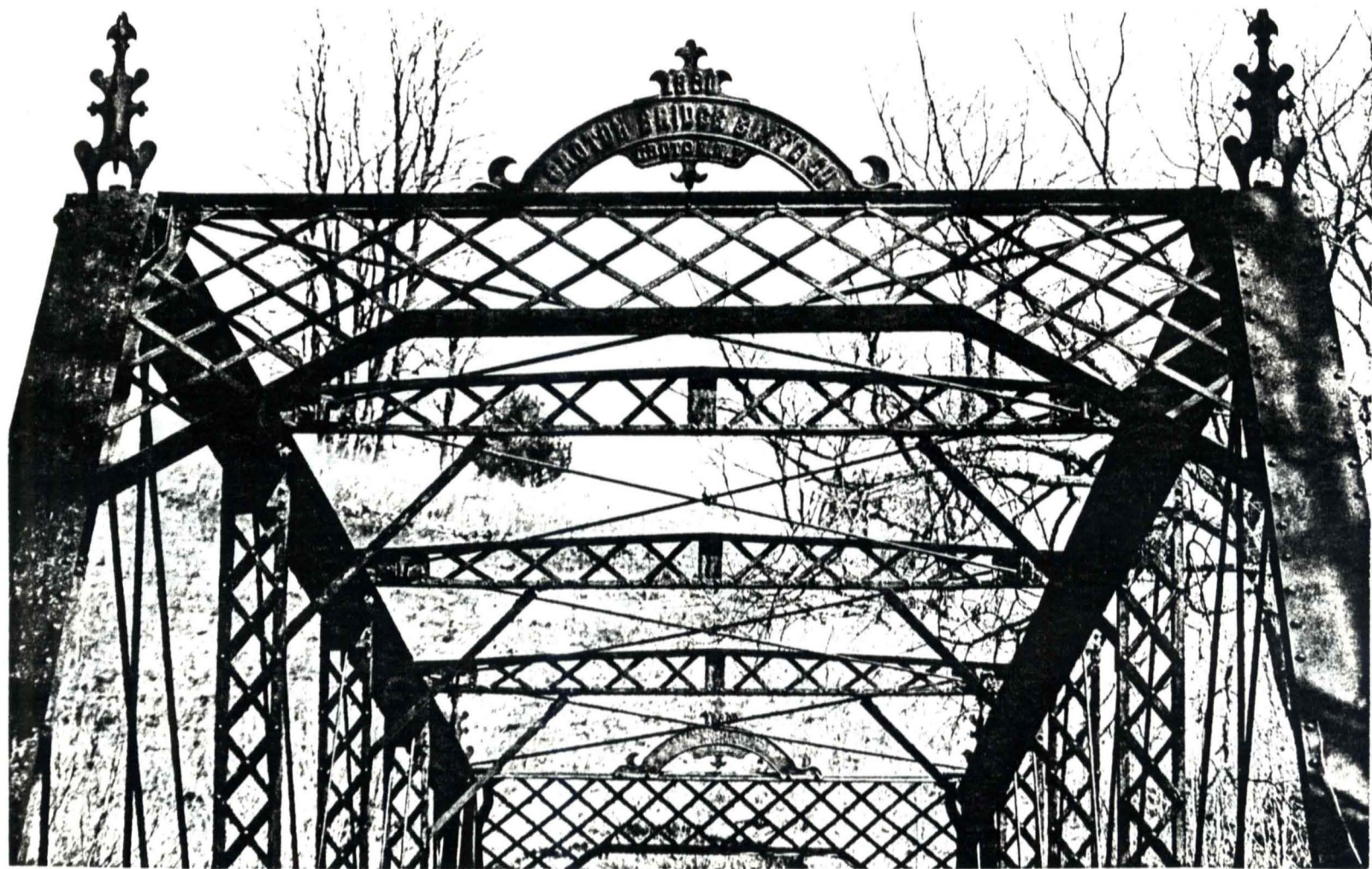
3.22 Cavendish, Vt., Howard Hill Road, Black River, Pratt through truss, 1890, NR, decorated portal.
