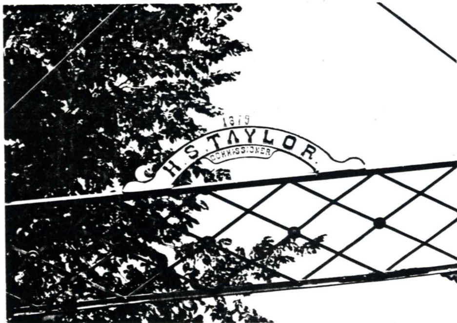
3.53 Pearl Creek, N.Y., Crossman Road, Catka Creek, Pratt through truss, 1879, potential NR, latticed portal, bridgeplate.
