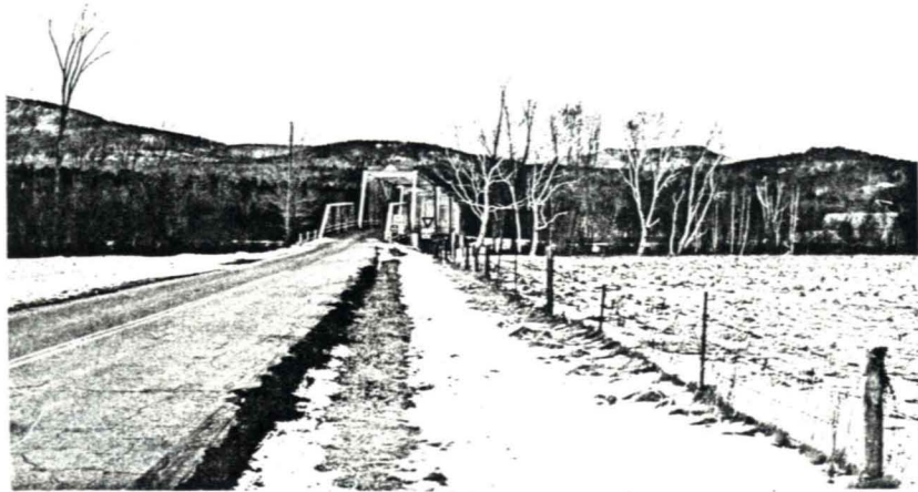
3.12 Shelburne, N.H., North Road, Androscoggin River, 5 span Pratt truss, 1897, NR, approach.
