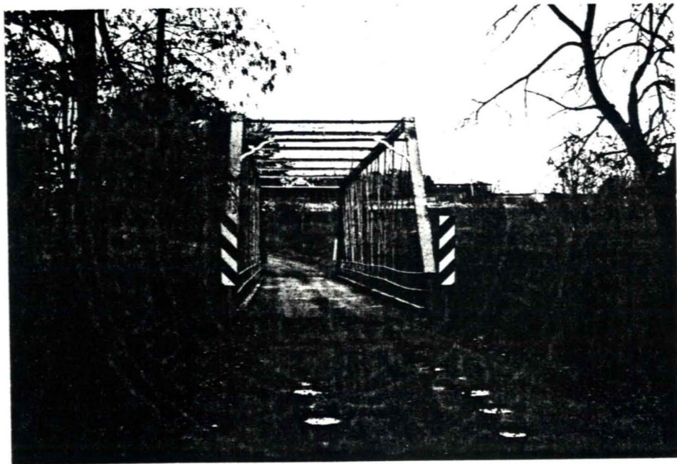
3.51 Pearl Creek, N.Y., Crossman Road, Catka Creek, Pratt through truss, 1879, potential NR, end approach.
