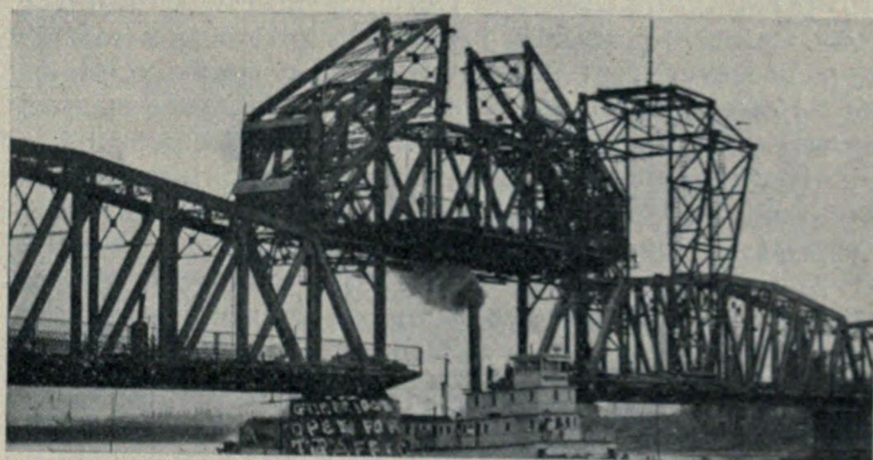
The lift span open. This span is fifty feet above high-water mark.
