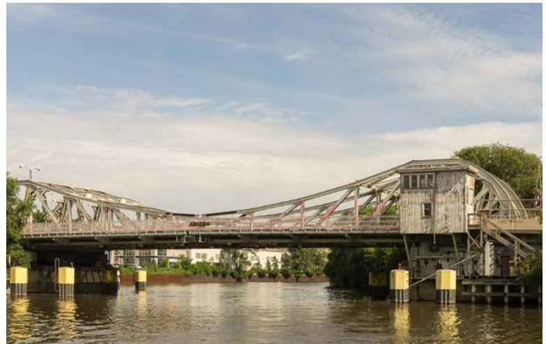
Division St Bridge across the North Branch
