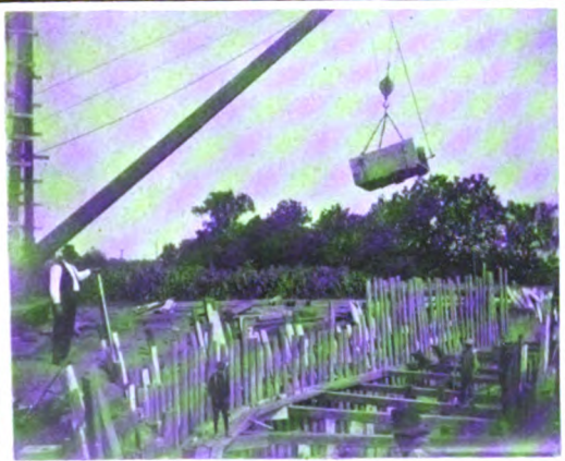
Open Cut Intercepting Sewer Lawrence Ave. Near River
