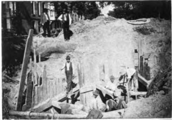
Cut Intercepting Sewer 21 st and Prairie Ave.
