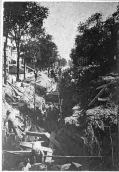
Open Cut Looking South on Prairie Ave.
