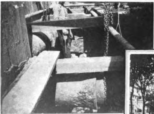
Intecepting Sewer at Intersection of 14 th St. and Clark
