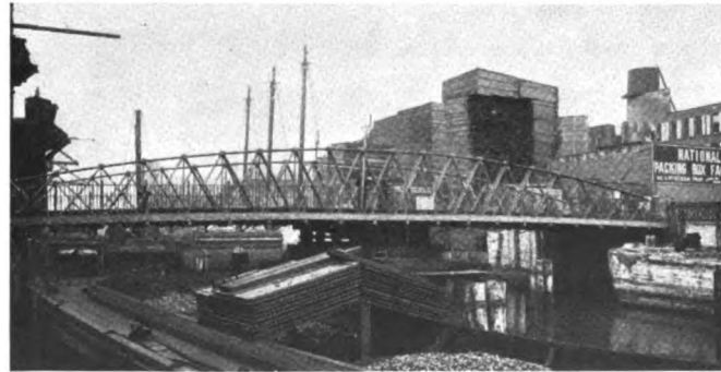
Old type of obstructive center pier swing bridge in a congested location.
