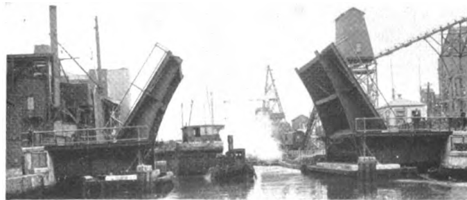
Highway Scherzer Rolling Lift Bridge across Gowanus Canal, Brooklyn, New York.
