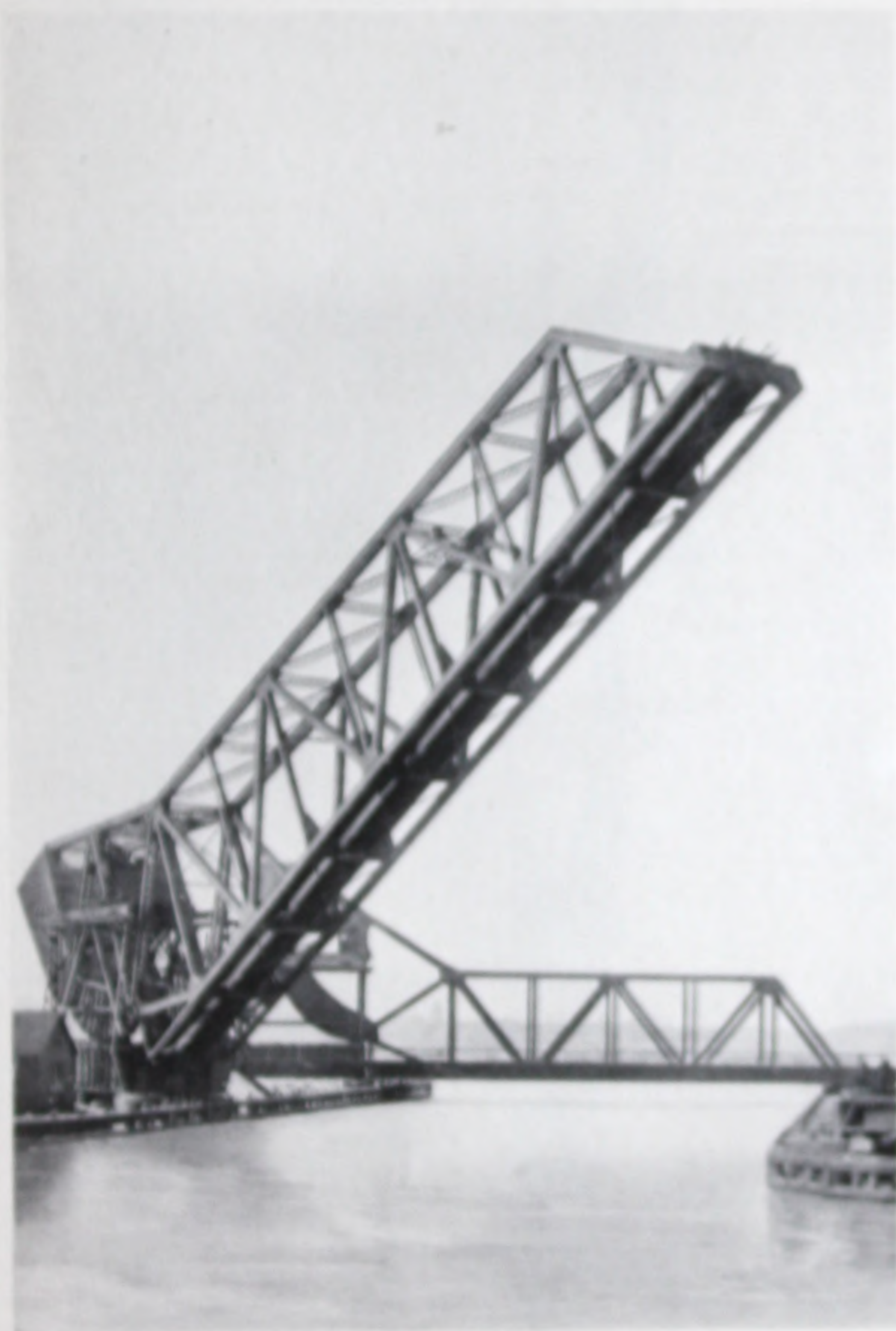
Scherzer Rolling Lift Bridges Across the River Rouge at Detroit, Michigan. for the Solvay Process Company The latest Scherzer bridges
