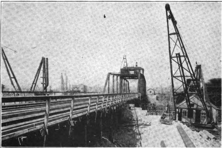
Fig. 3. Temporary Bridge. Excavating for Retaining Walls.
