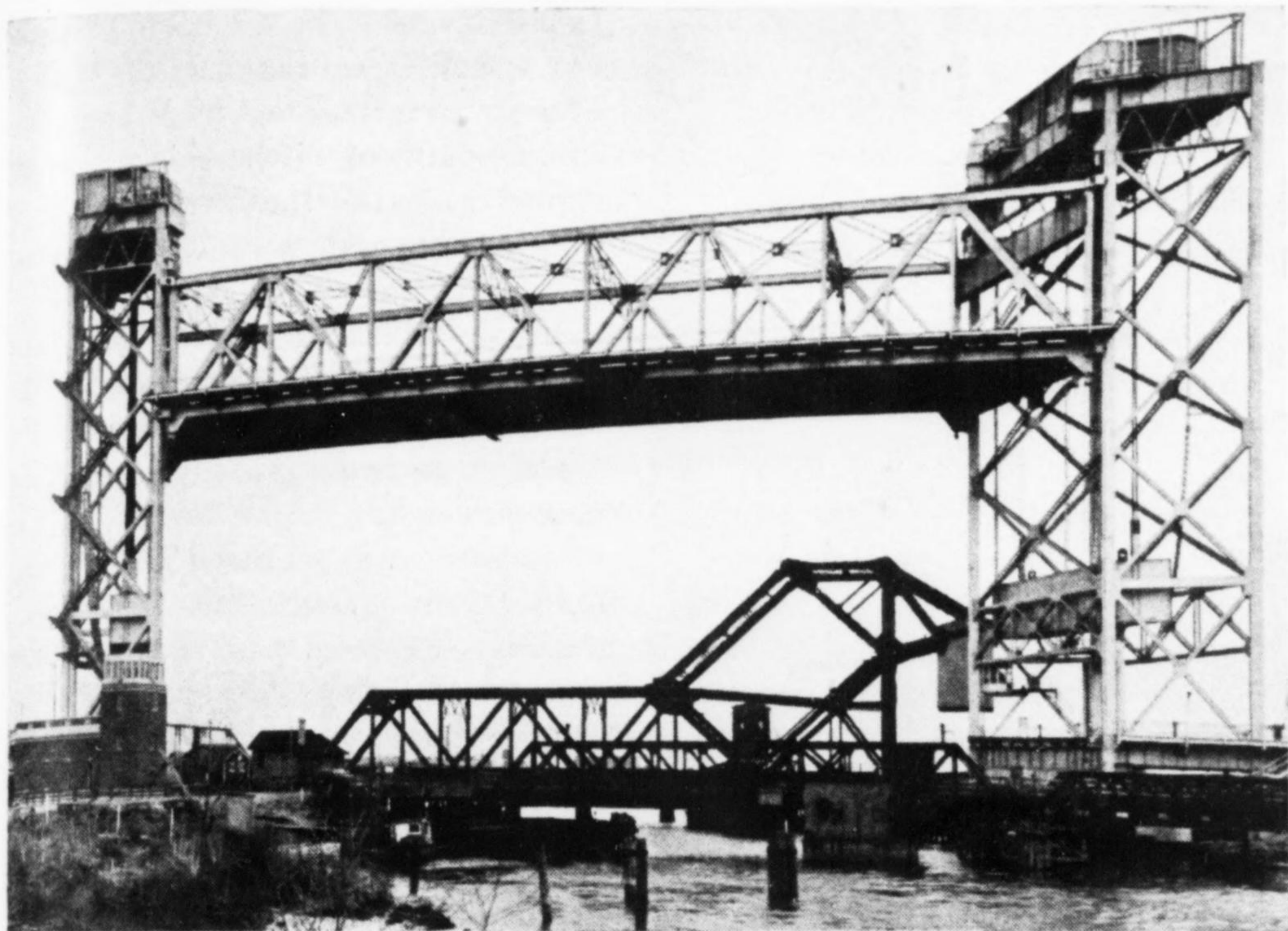
Fig. 1. Chicago lift bridge, built on a skew, is raised by 80 wire ropes operating over 15 ft. dia. sheaves
