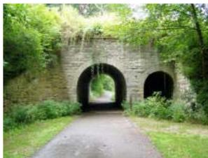
**Bridge Type:** Semicircular stone arch bridge widened on one side with concrete.
