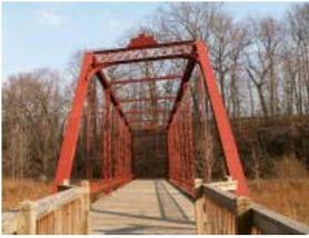
**Bridge Type:** Seven panel Pratt through truss with pinned connections.
