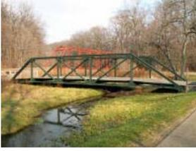
**Bridge Type:** Five panel full-slope Pratt pony truss with riveted connections.
