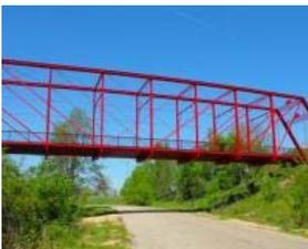
**Bridge Type:** Eleven panel Whipple through truss with pinned connections.
