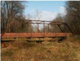
**Bridge Type:** Six panel Pratt through truss with pinned connections.
