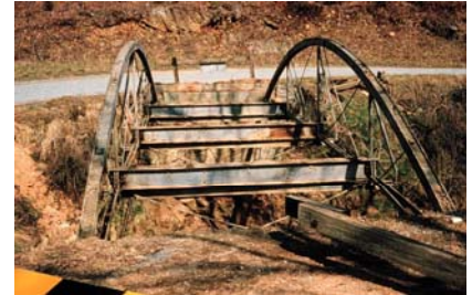
Figure 1. The bridge in its original location in Bedford, VA being dismantled for relocation to the Ironto Wayside.
