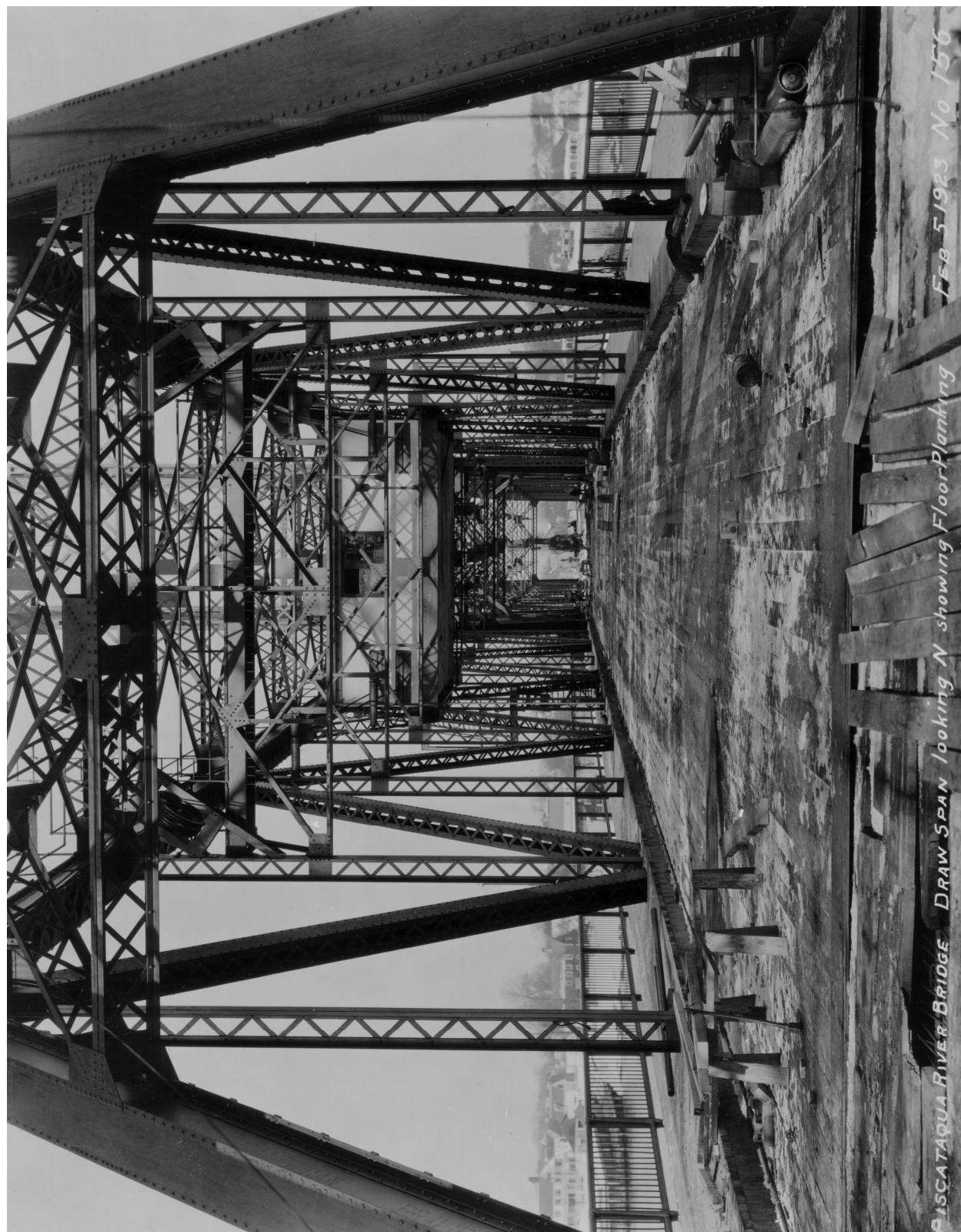
Plate N-54: Draw Span looking North Showing Floor Planking Feb 5 1923 No. 156 (Portsmouth Athenaeum-Norris Collection 1476)
