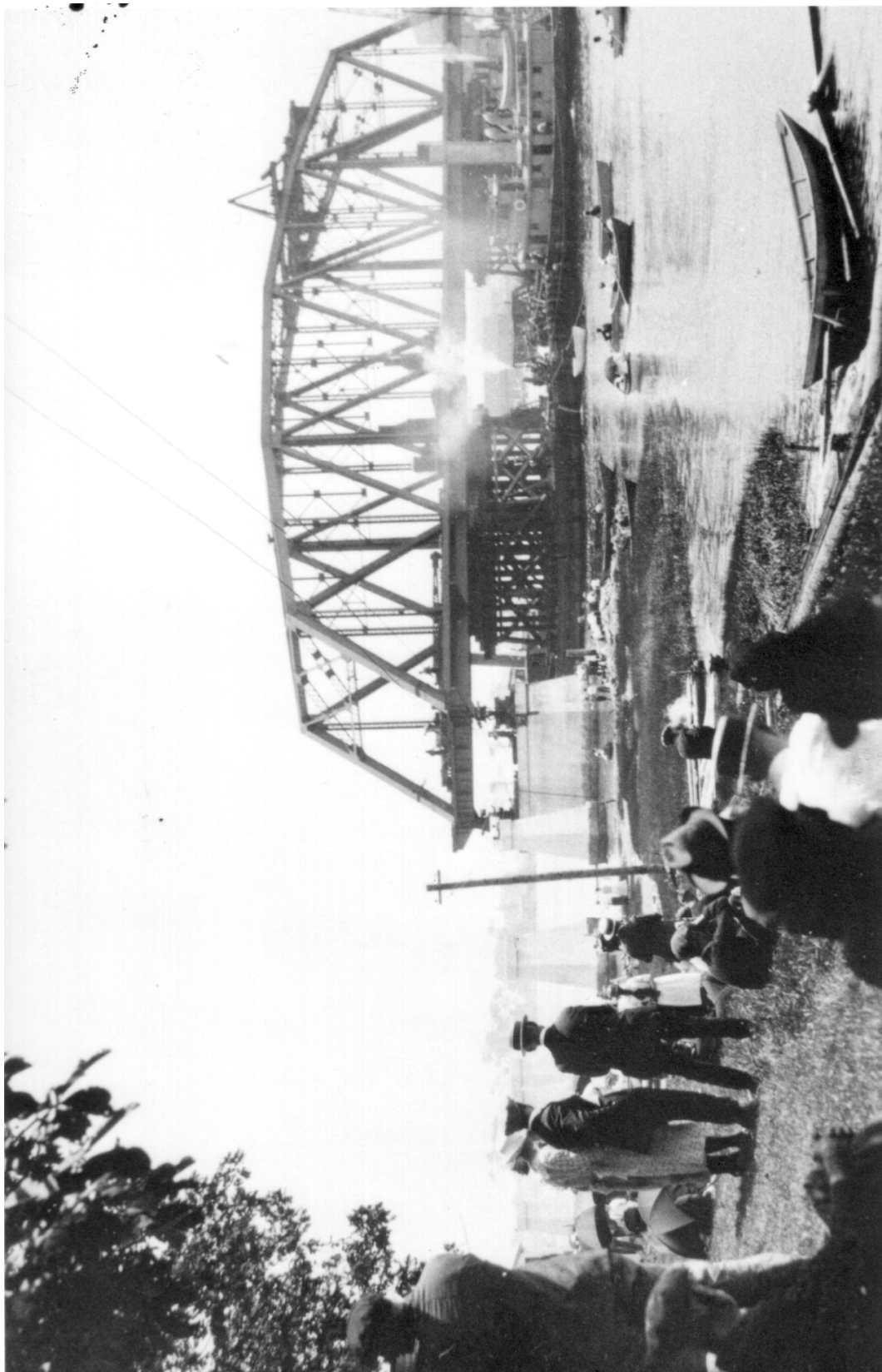
Plate N-28: Placing North Span, July 8 1922 (Portsmouth Athenaeum-Norris Collection PG 158B)
