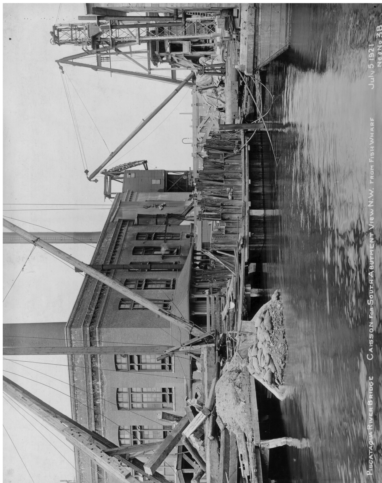
Plate N-16: Caisson for South Abutment, July 5, 1921 (Portsmouth Athenaeum-Norris Collection 1382)
