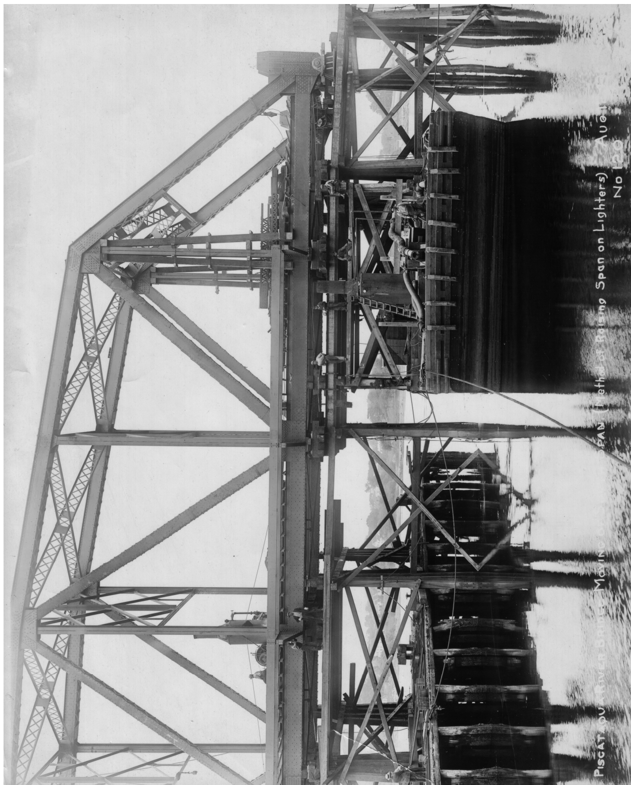
Plate N-32: Raising South Span on Lighters Aug 7 1922 No. 120 (Portsmouth Athenaeum-Norris Collection 1422)
