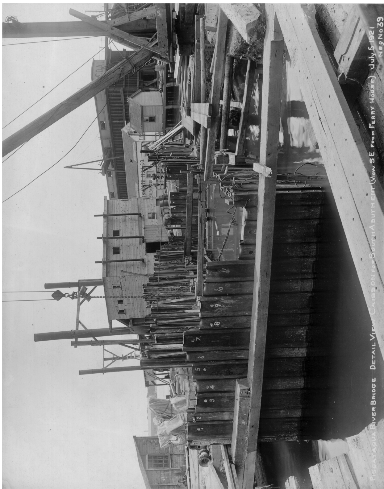
Plate N-17: Caisson for South Abutment, July 5, 1921 (Portsmouth Athenaeum-Norris Collection 1383)
