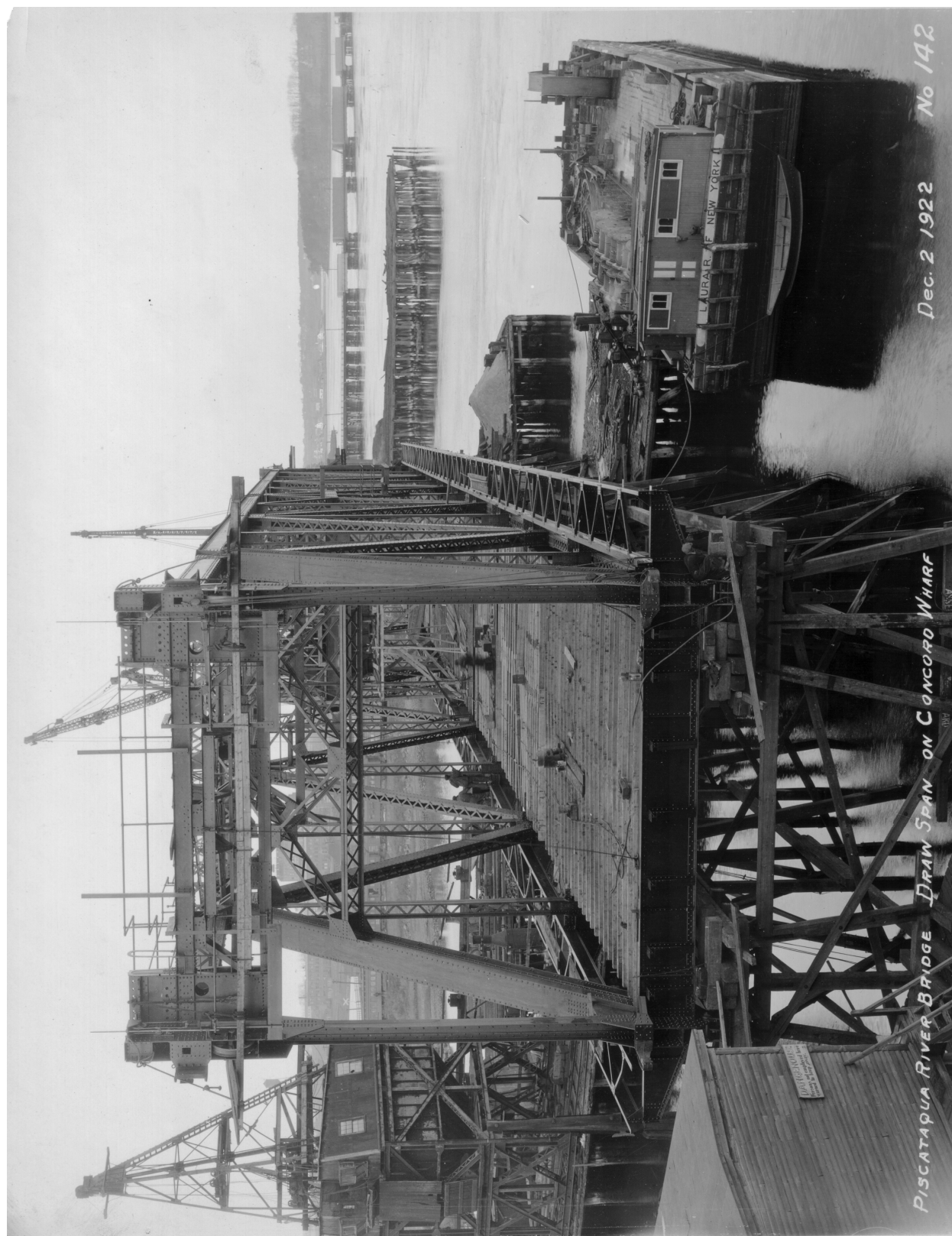
Plate N-46: Draw Span on Concord Wharf, Dec. 2 1922 No. 142 (Portsmouth Athenaeum-Norris Collection 1441)
