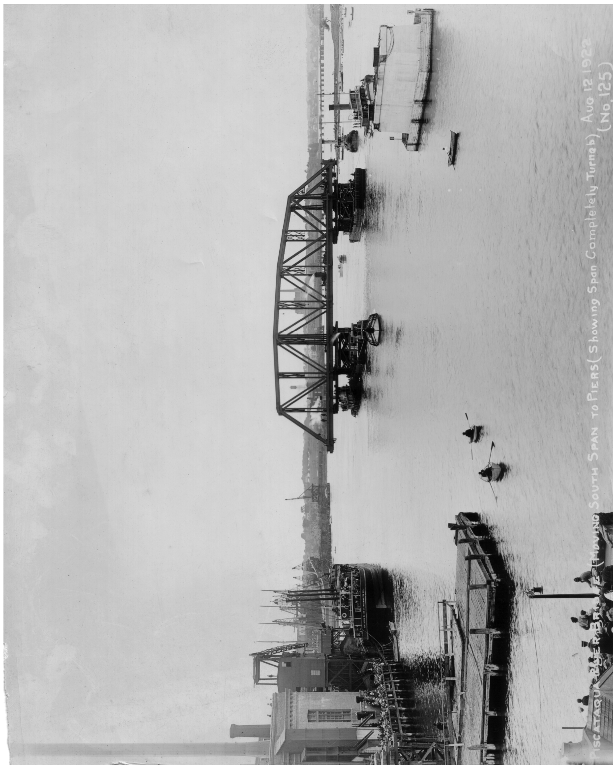
Plate N-36: Moving South Span to Piers (Showing Span Completely Turned) Aug 12, 1922 No. 125 (Portsmouth Athenaeum-Norris Collection 1425)
