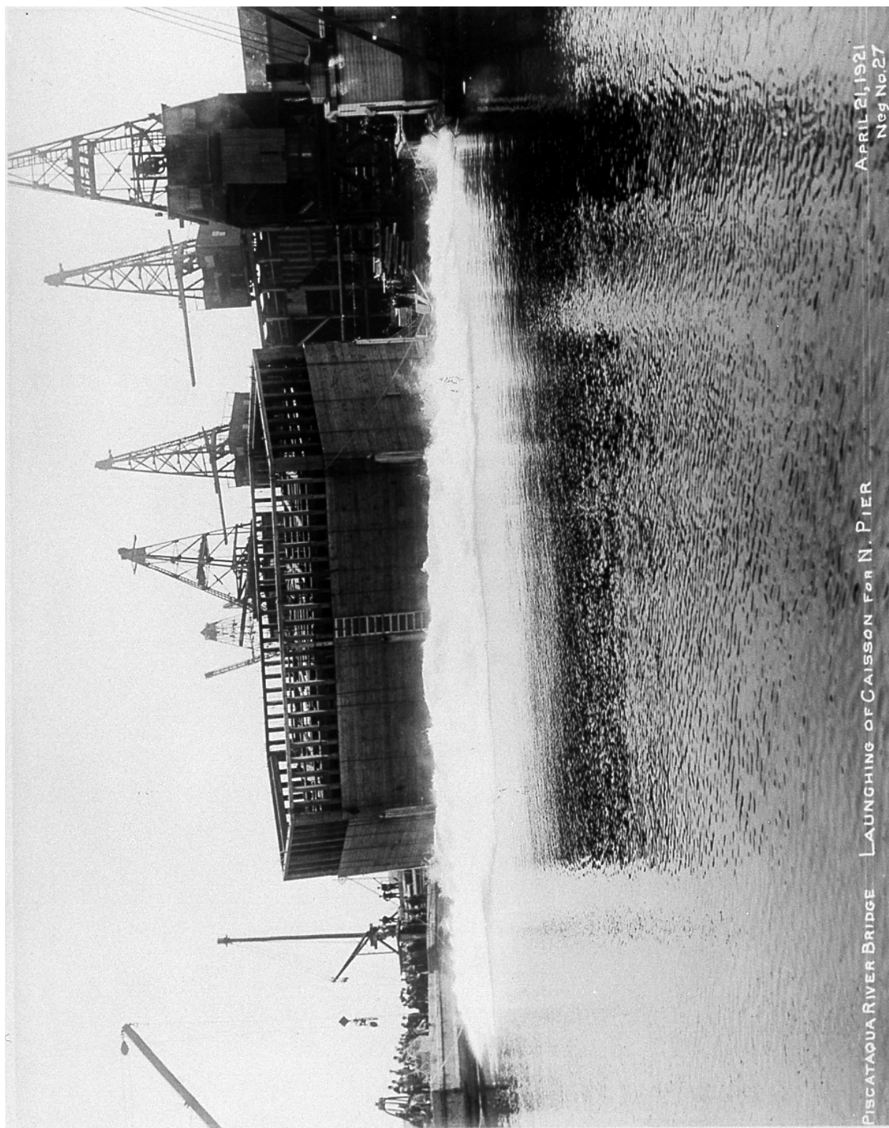
Plate N-11: Launching of Caisson for North Pier, April 21, 1921 (Maine DOT ME026)
