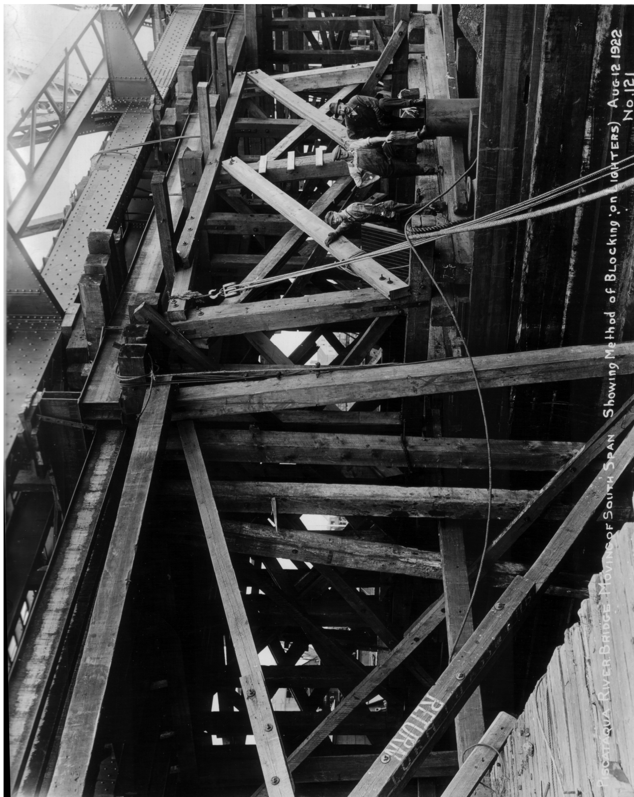
Plate N-34: South Span – Showing Blocking on Lighters, Aug 12 1922. No 121(Portsmouth Athenaeum-Norris Collection 1423)
