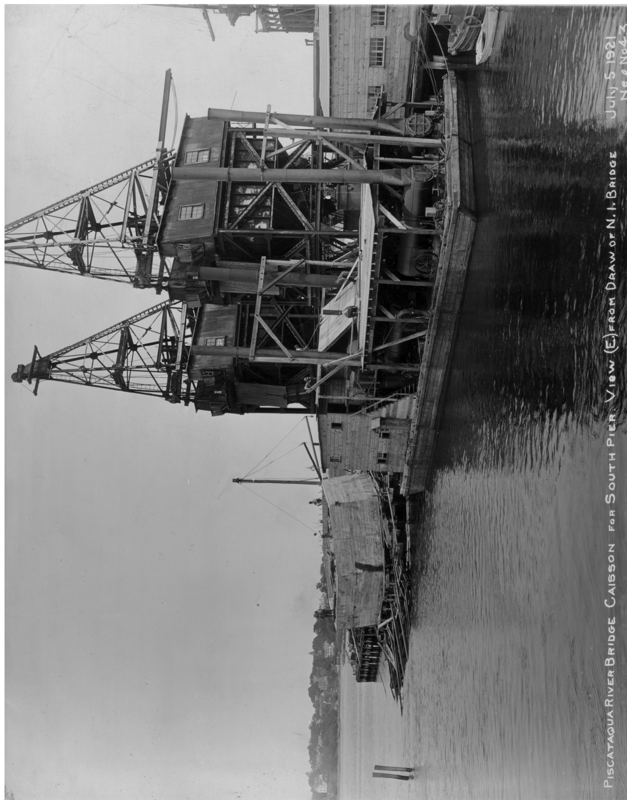
Plate N-18: Caisson for South Pier, July 5, 1921 (Portsmouth Athenaeum-Norris Collection 1385)
