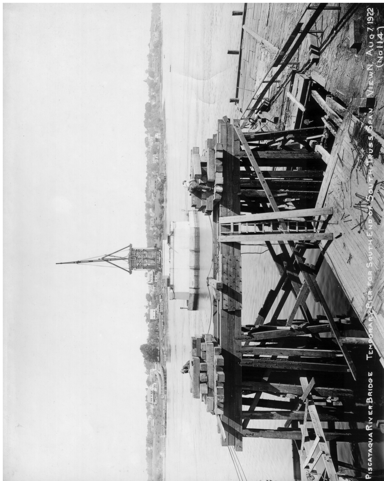
Plate N-29: Temporary Pier for South End of South Truss Span, Aug 7 1922 (Portsmouth Athenaeum-Norris Collection 1417)
