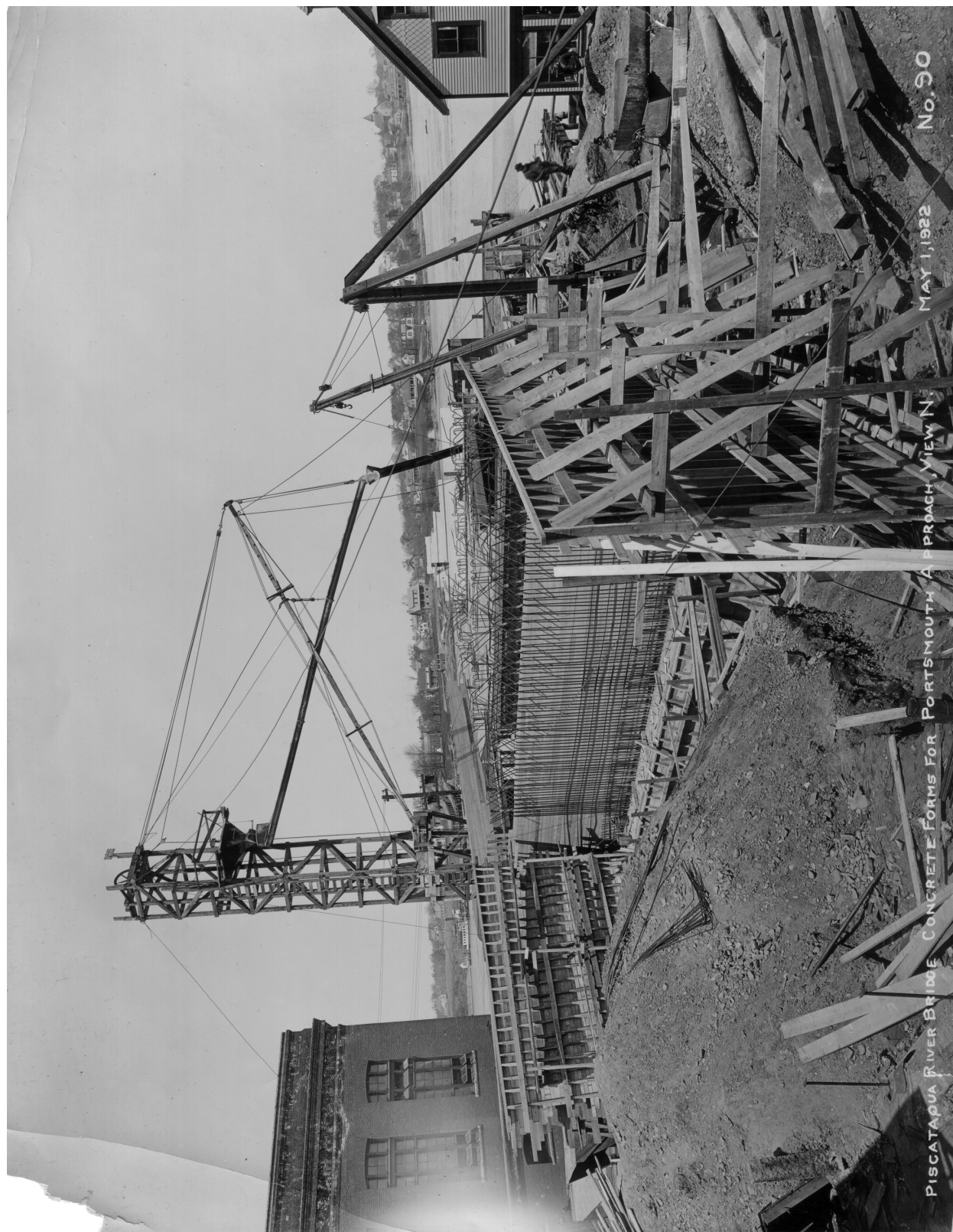
Plate N-25: Concrete Forms for Approach, May 1 1922 (Portsmouth Athenaeum-Norris Collection 1399)
