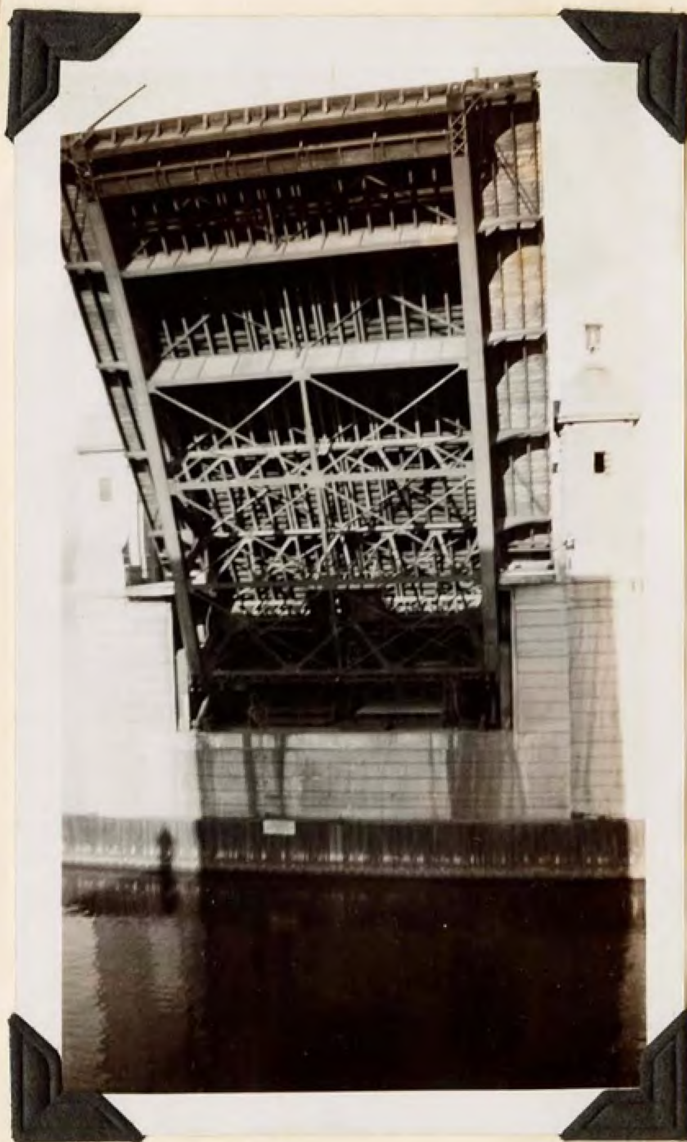
View showing the under side of the south leaf of the Bascule, taken while the draw was open.
