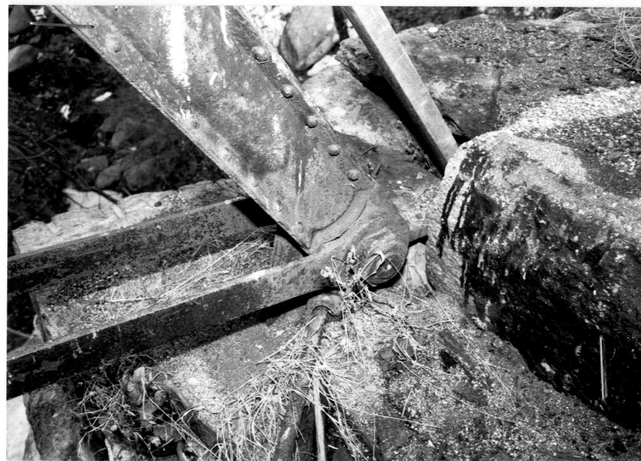
S TRUSS, W END, BEARING ON ABUTMENT, FROM NE 11-17-87
