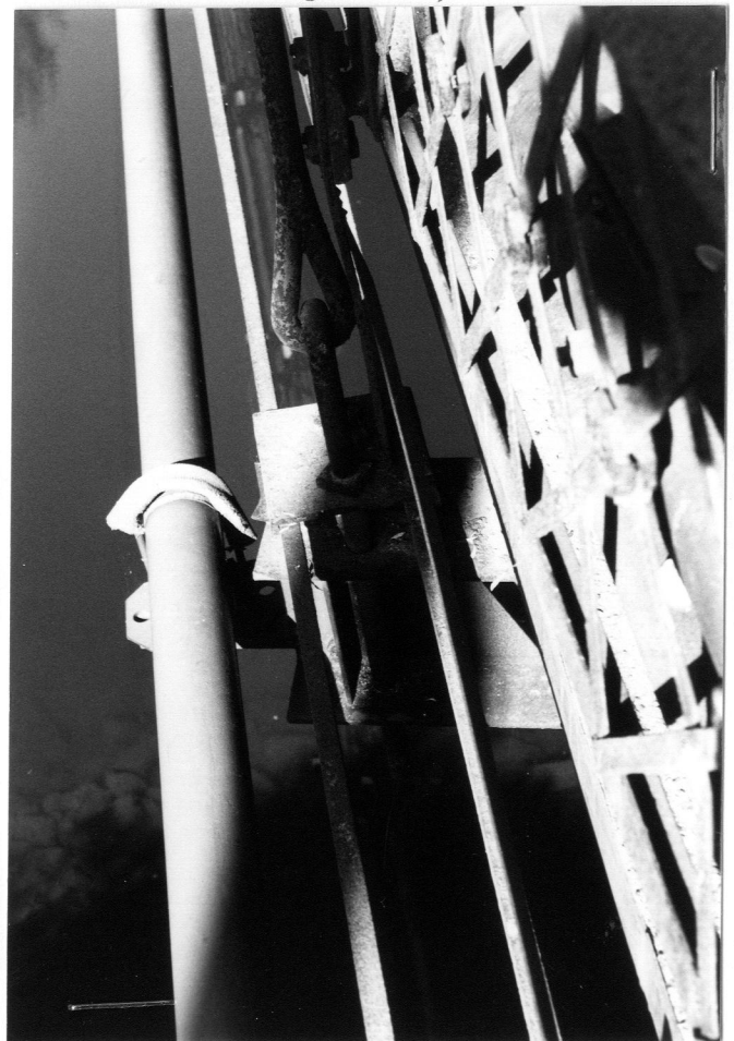
S TRUSS, POWER END PANEL POINT (7-18-85)
