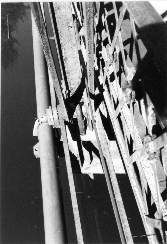
S TRUSS, LOWER INTERMEDIATE PANEL POINT (7-18-85)
