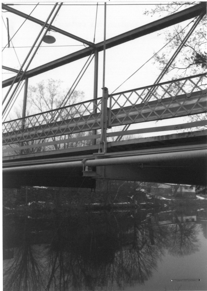
S TRUSS, EASTERN HIP VERTICAL LOWER PANEL POINT, FROM SE (11-17-87)
