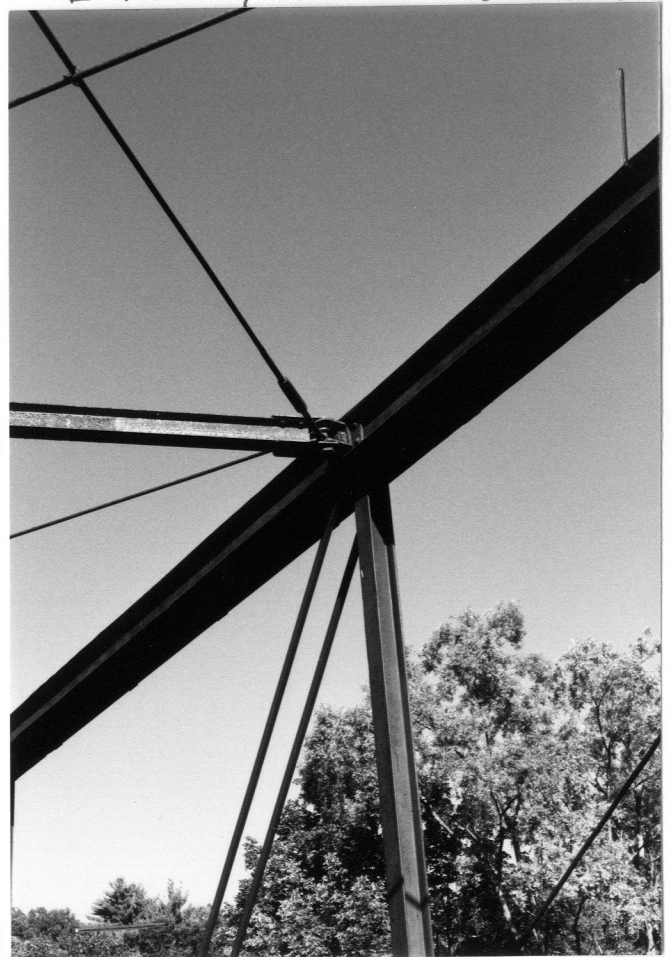
N TRUSS, UPPER INTERMEDIATE PANEL POINT (7-18-85)
