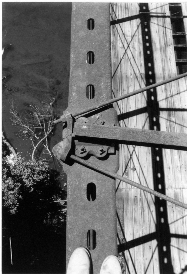
SE TRUSS, UPPER CHORD LATERAL CONNECTION (7-24-85)
