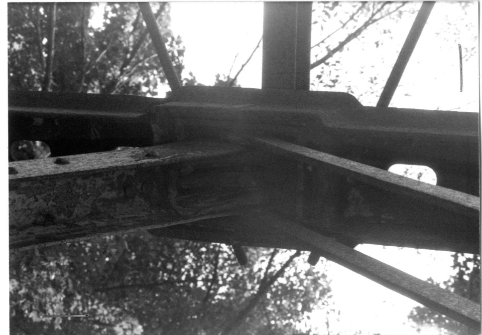
SE TRUSS UPPER CHORD PANEL POINT, FROM BELOW (8-14-86)
