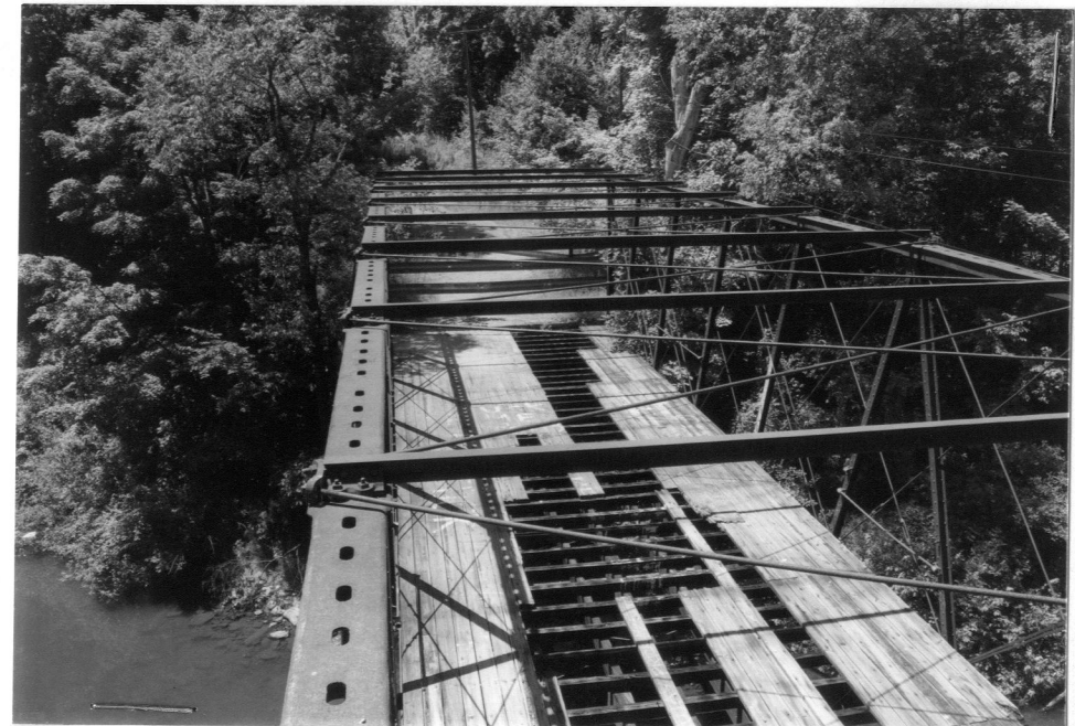
UPPER CHORDS + LATERAL SYSTEM FROM NE END OF SE TRUSS, LOOKING SW
