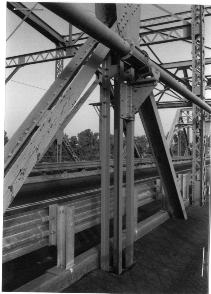
TYPICAL REPLACED SUBVERTICAL, 2ND SPAN FROM N, EASTERN TRUSS, FROM SE
