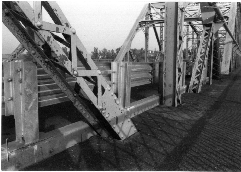
TYPICAL TRUSS WEB REINFORCEMENT, S SPAN, EASTERN TRUSS, NORTHERN END, FROM SE
