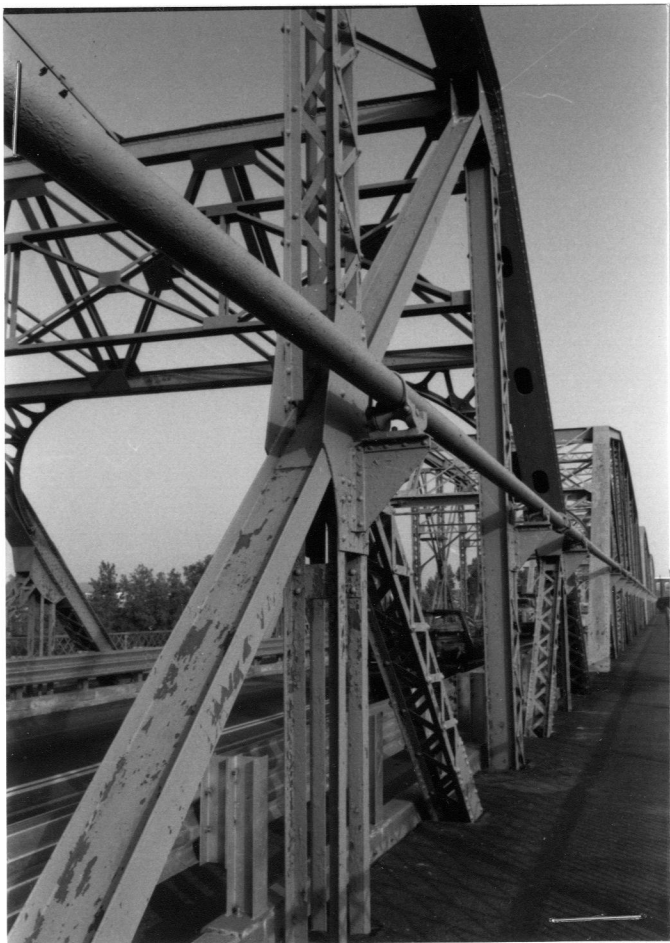
TYPICAL TRUSS REPLACEMENTS, S SPAN, EASTERN TRUSS, NORTHERN END, FROM SE
