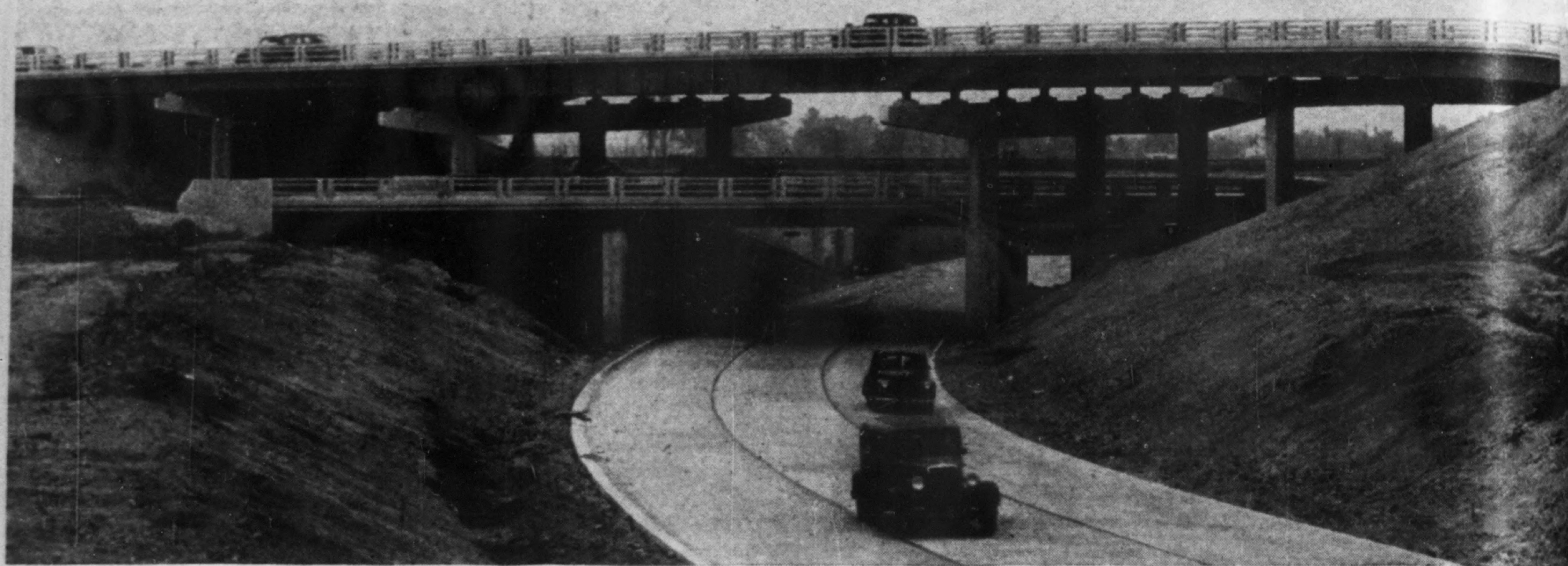
Fig. 1. Three-level crossings are required to separate through traffic from traffic flowing to and from the bomber plant.
