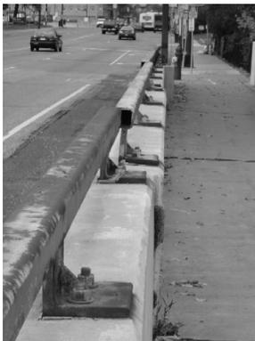
Figure 4. Looking north at the east vehicular railing on the north approach. Settlement has led to shifting of the barrier both vertically and laterally.
