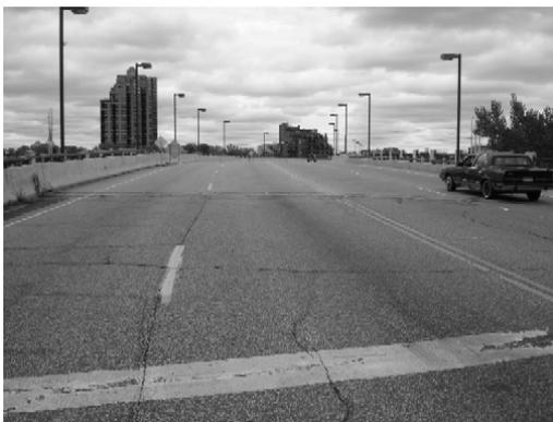
Figure 1. Looking north at the bridge from the south approach. The vehicle barriers are not symmetrical on the south end. A low profile barrier is provided on the east and a taller barrier is provided on the west. The approach roadway pavement is deteriorated and has extensive cracking.
