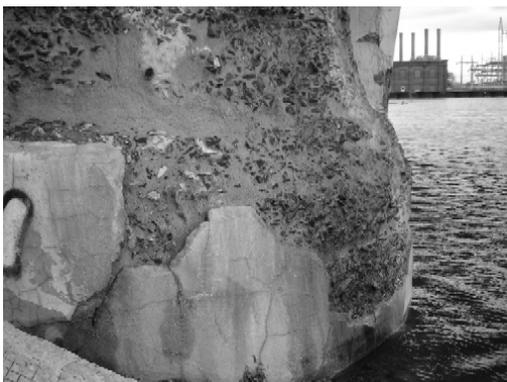
Figure 8. Looking east at the northernmost river pier. Shotcrete repairs to the pier have failed. Large spalled regions, with water draining out of the deteriorated area, were visible during the site visit.
