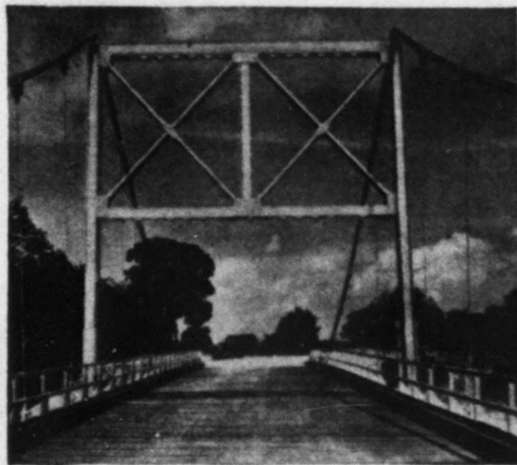
Fig. 3—Bridge roadway 20 ft. wide consists of 2x4-in. creosoted pine boards laid on edge.
