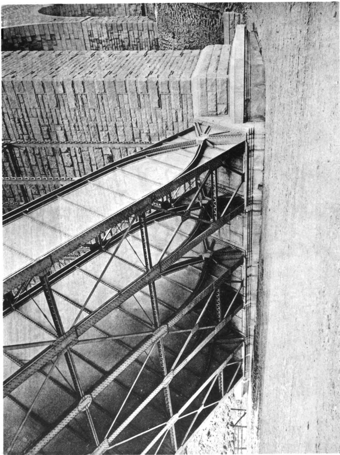
BEARING OF STEEL ARCH UPON PIER III.
