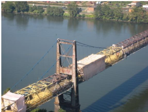
Photo taken from the hilltop on W. Va. side, showing the progress of the 2010 rehabilitation work by West Virginia DOT, taken Aug 28, 2010. Yellow paint on box truss frame visible as is the blue on the main cable. Tarps cover areas being sand blasted. Courtesy of Mrs. Donna Diserio of Follansbee, W. Va.
