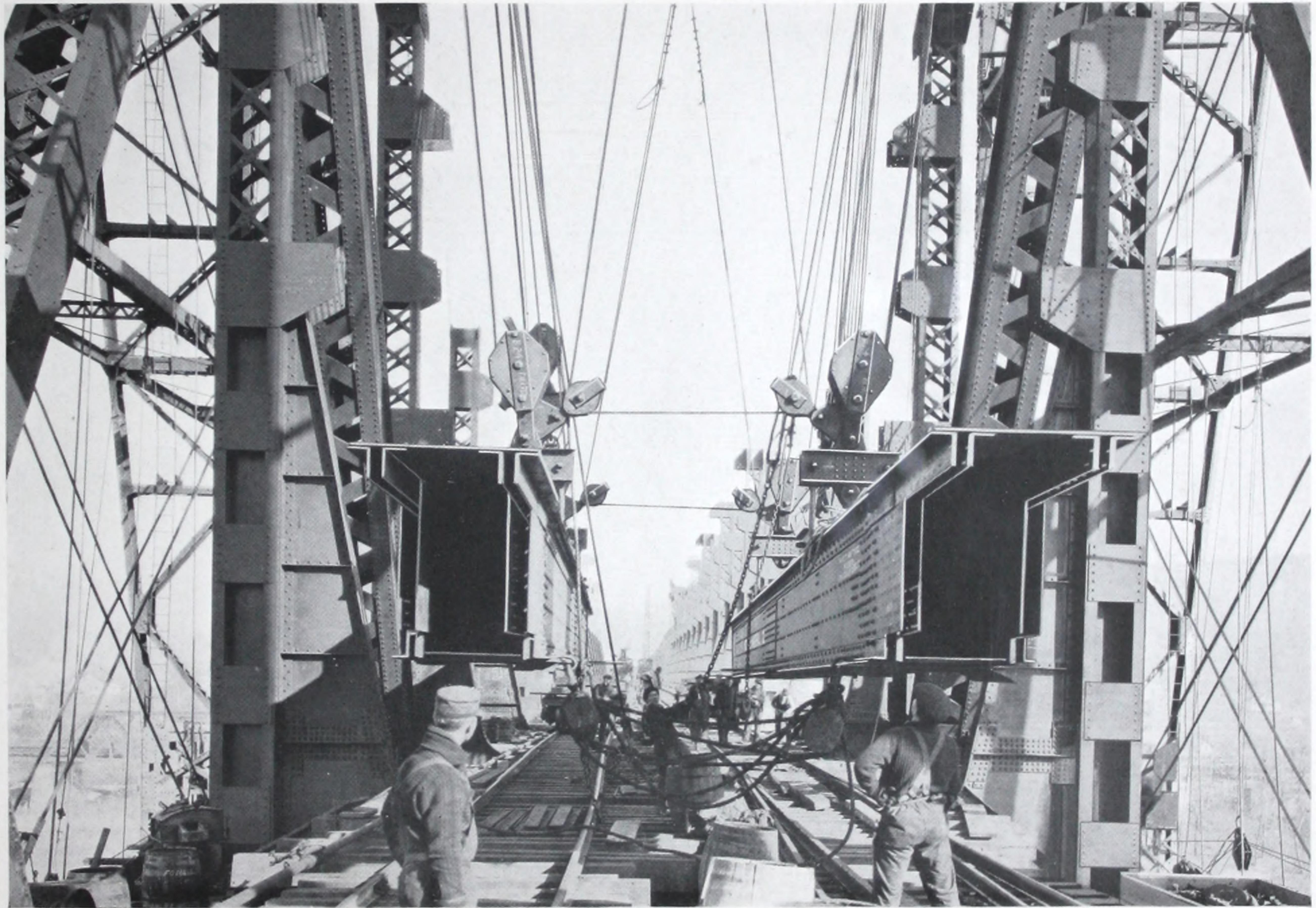
OHIO SPAN—Members for both trusses being lifted simultaneously by falls from gantry traveler.
