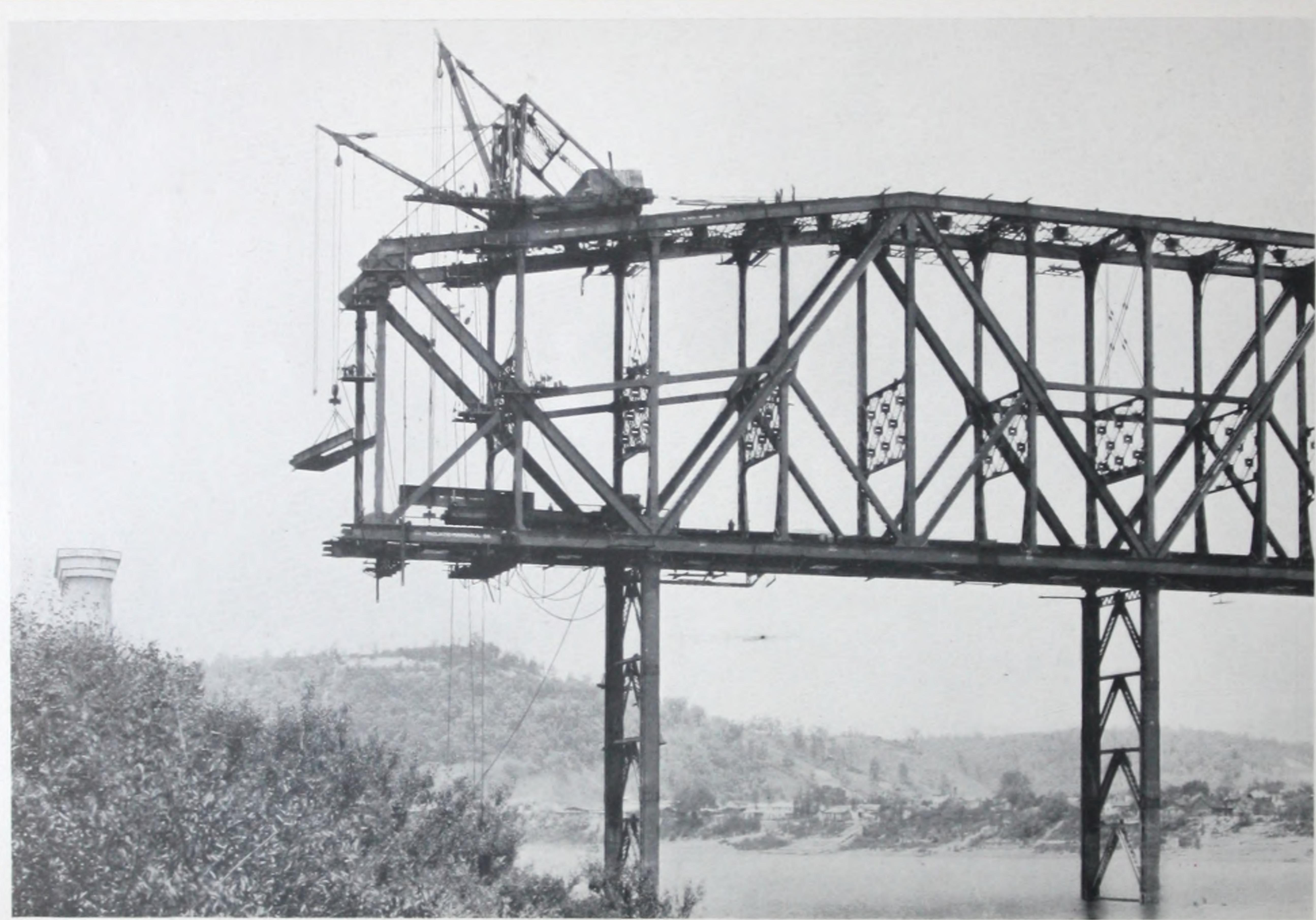
KENTUCKY SPAN—Showing creeper traveler and steel falsework bents at L-8 and L-4.
