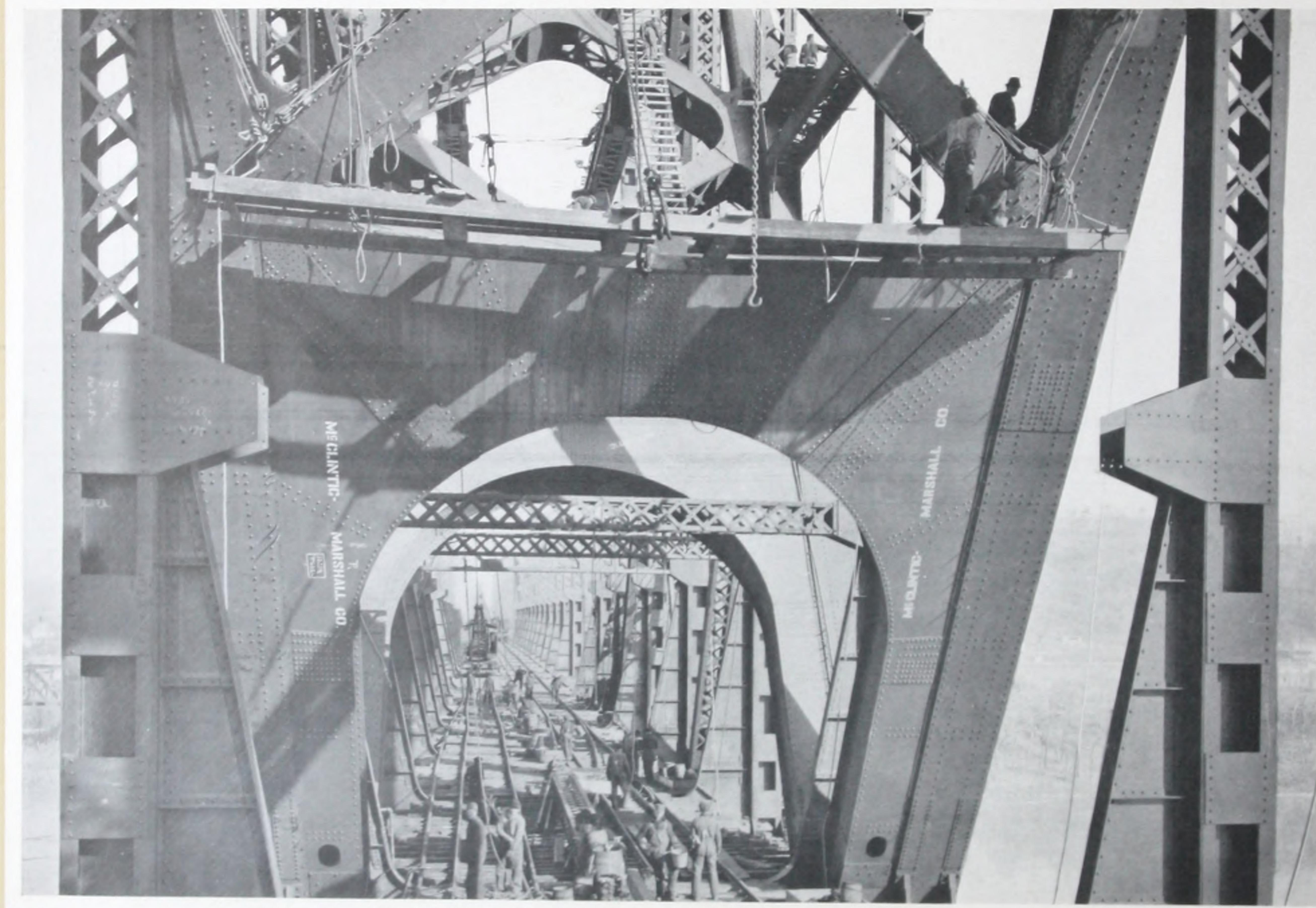
CENTER PIER.—Riveted plate portals at junction of Ohio and Kentucky spans.
