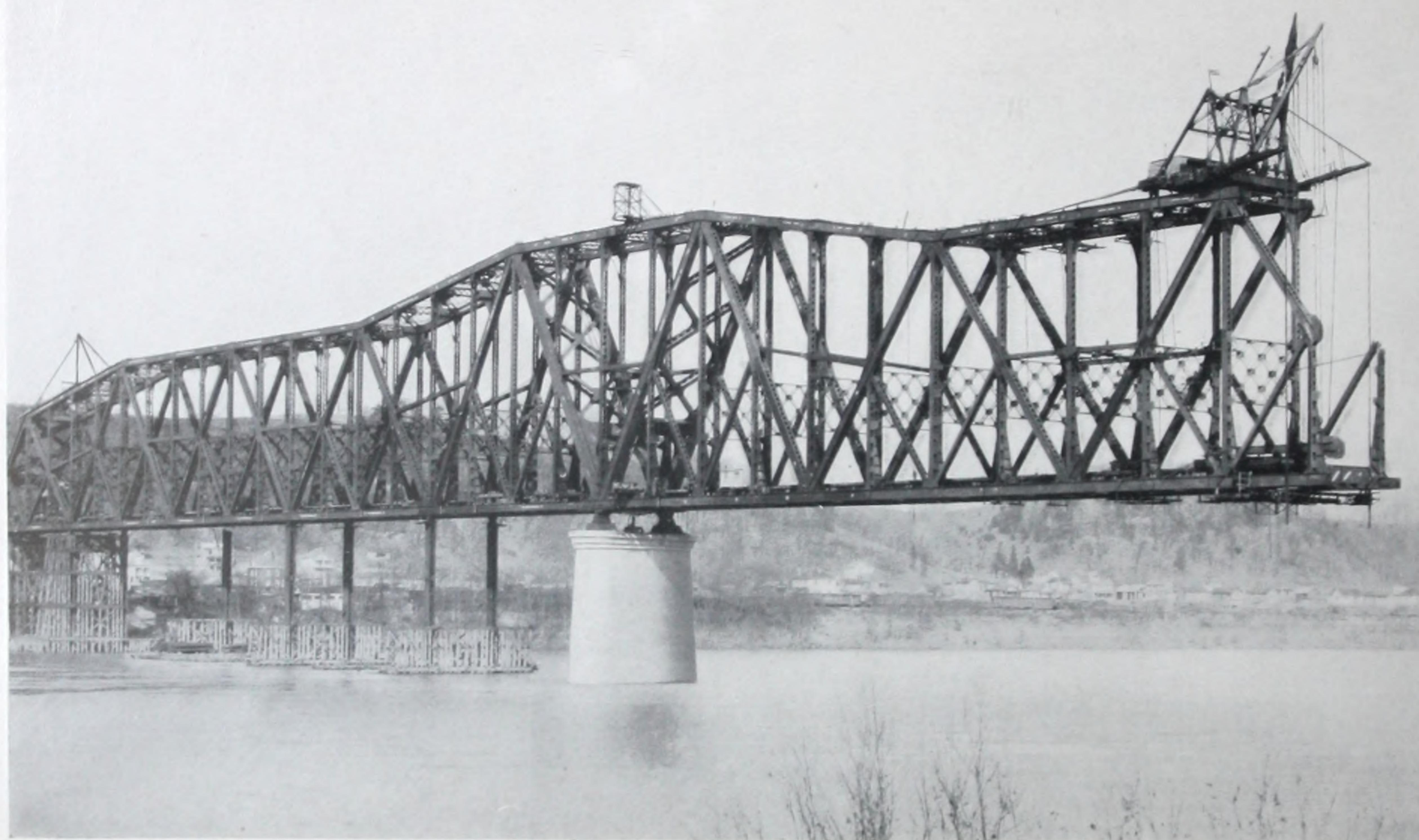
OHIO SPAN—View from Kentucky side showing Ohio span swung free from falsework which is partially removed.
