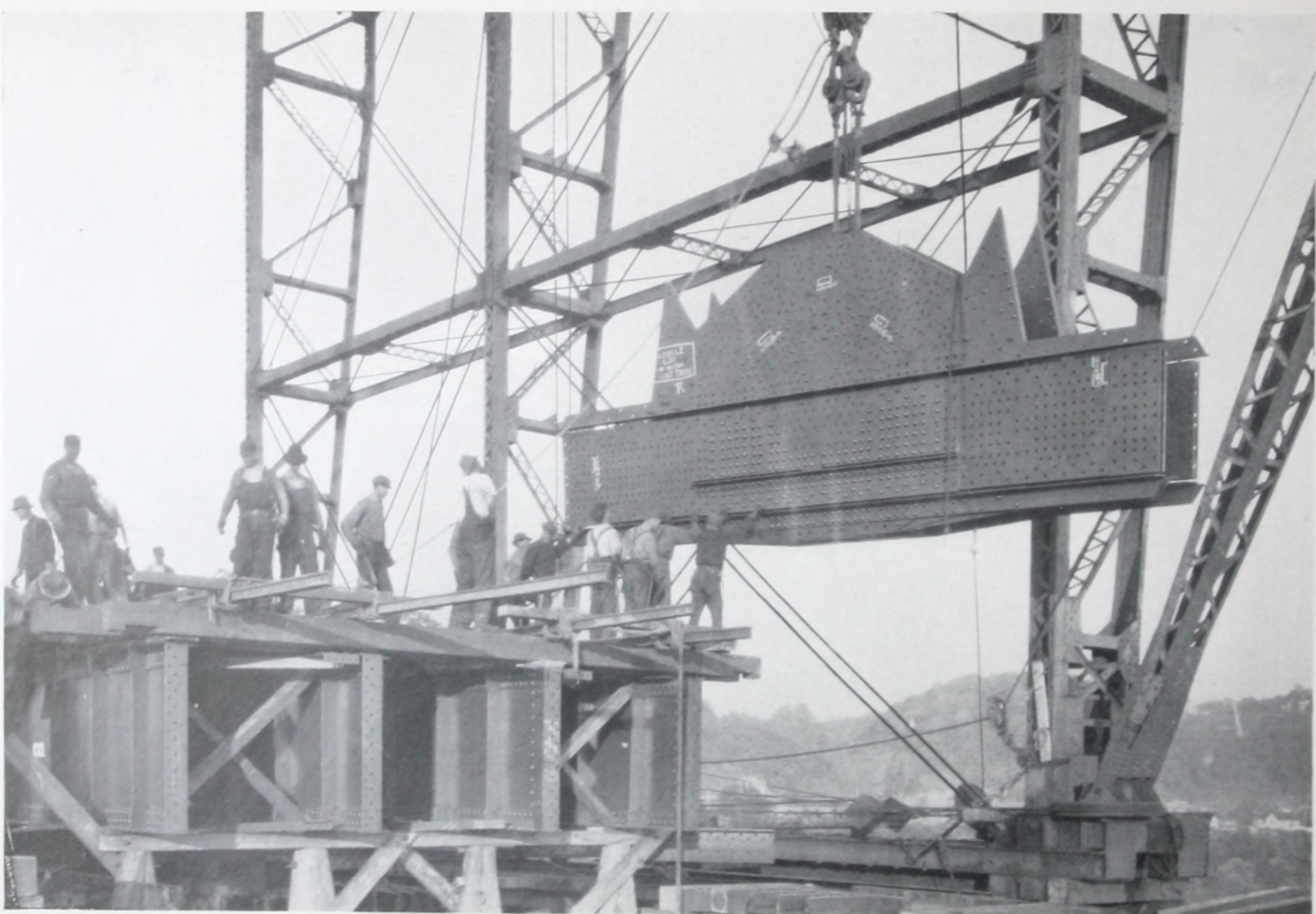
CENTER PIER—Setting center lower chord section with gussets over center pier bearing. Weight 40 tons.
