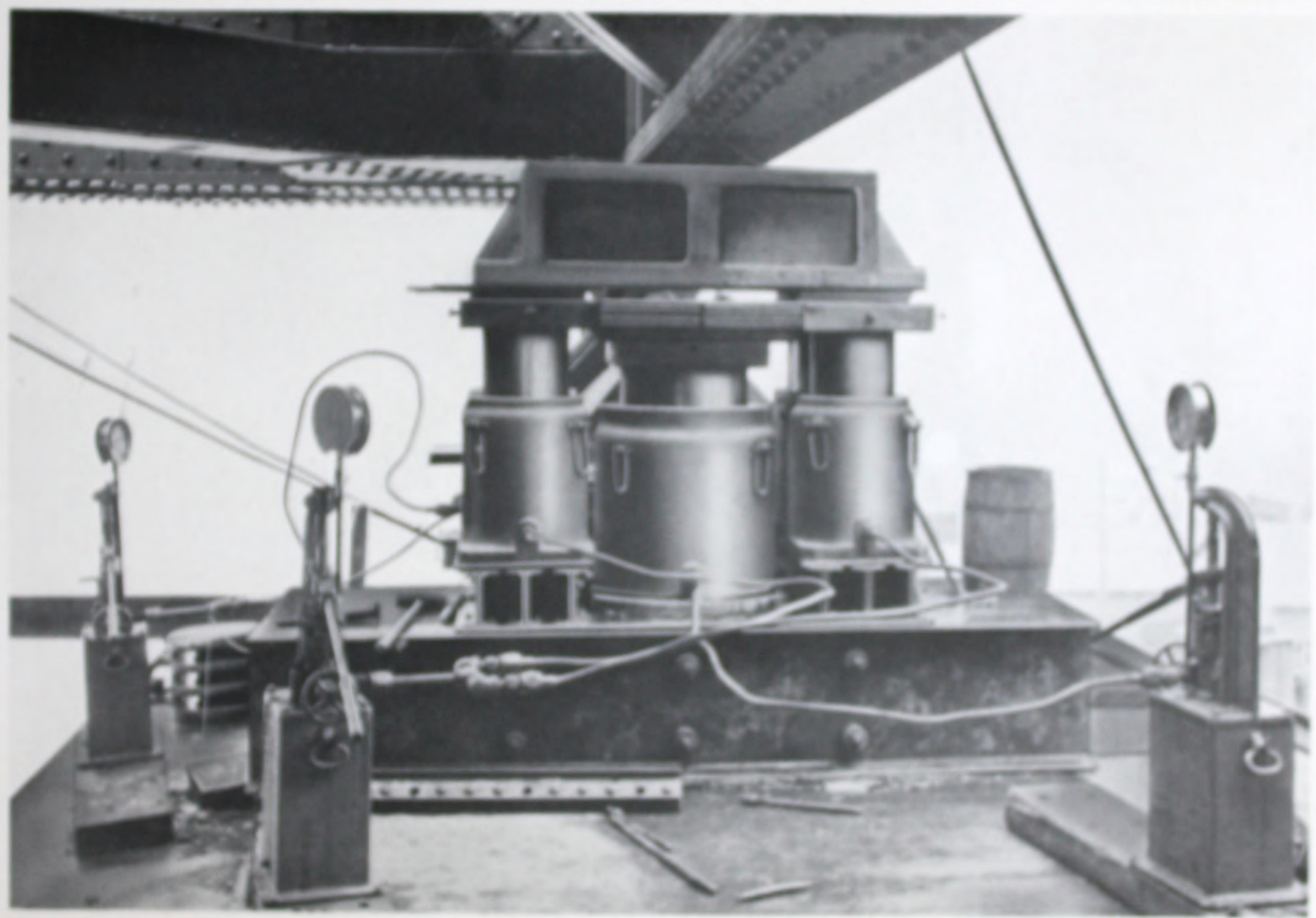
SWINGING SPAN—View showing arrangement of one 500-ton and four 200-ton hydraulic jacks used under scaffolding and floor beams to swing both spans.
