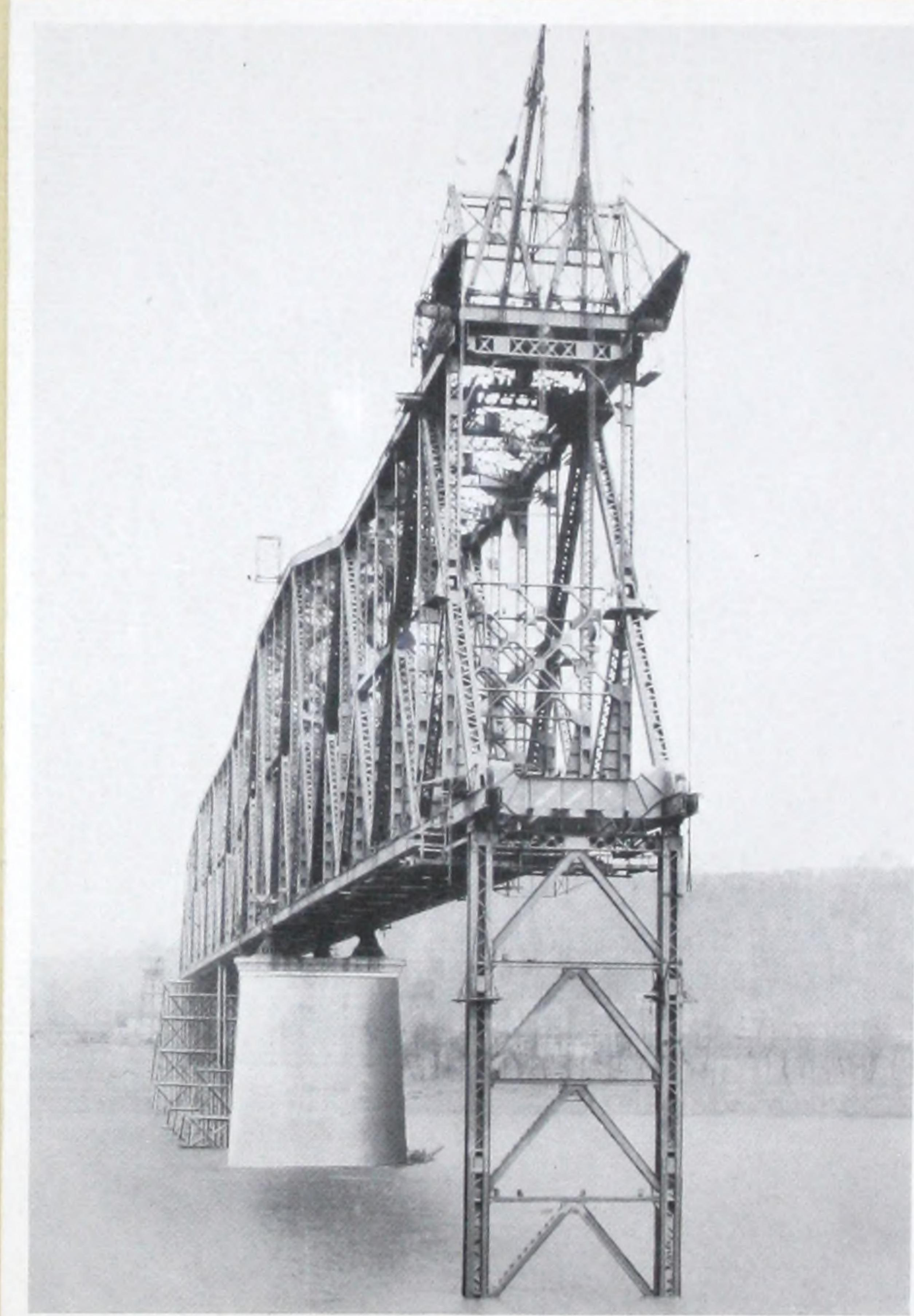
**KENTUCKY SPAN**—Showing Kentucky span with panel points L-8 resting on steel tower after being cantilevered 465 ft.
