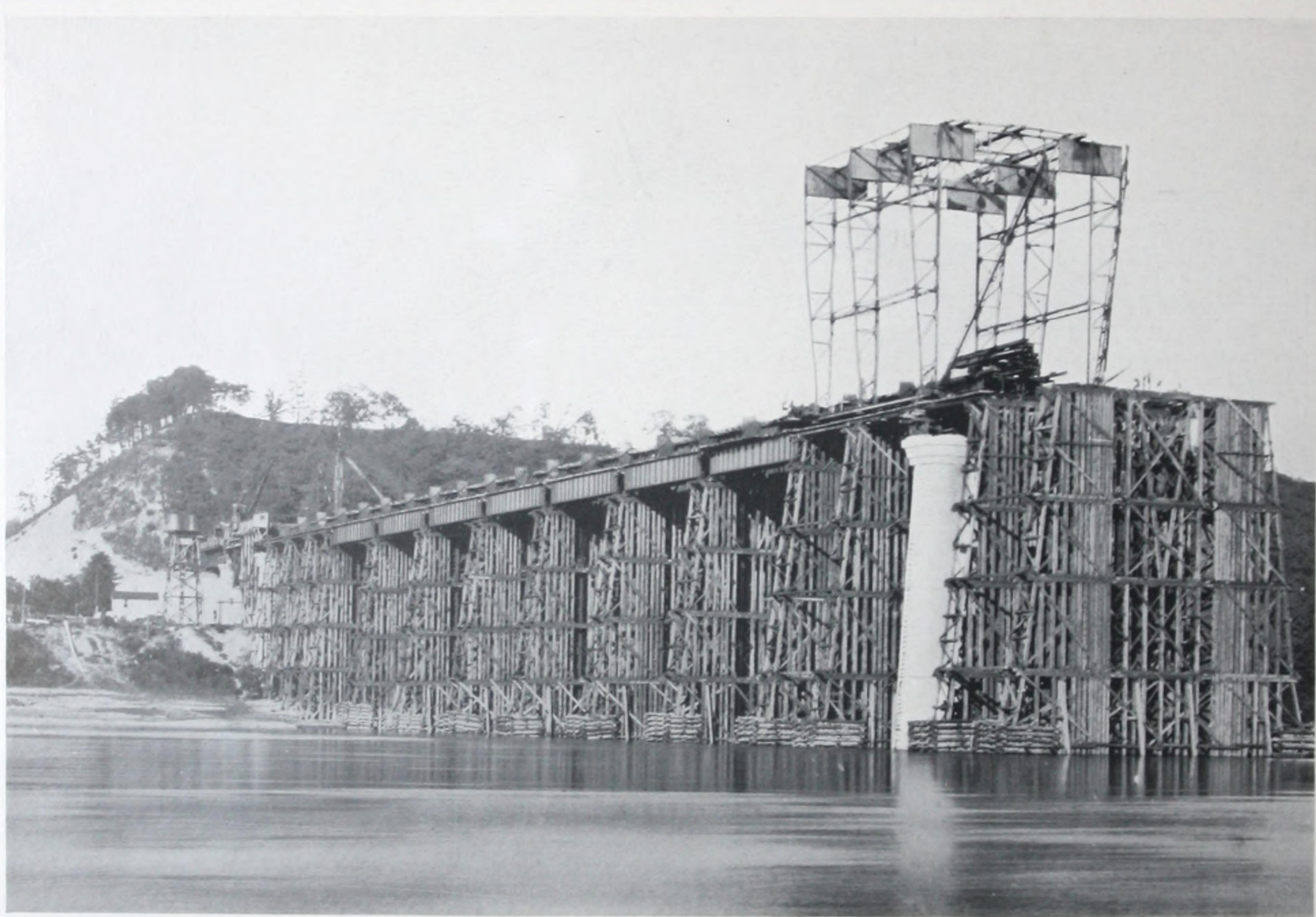
OHIO SPAN—Falsework completed,—1,250,000 Ft. B. M. used. Gantry traveler 60 ft. high with two 80 ft.
