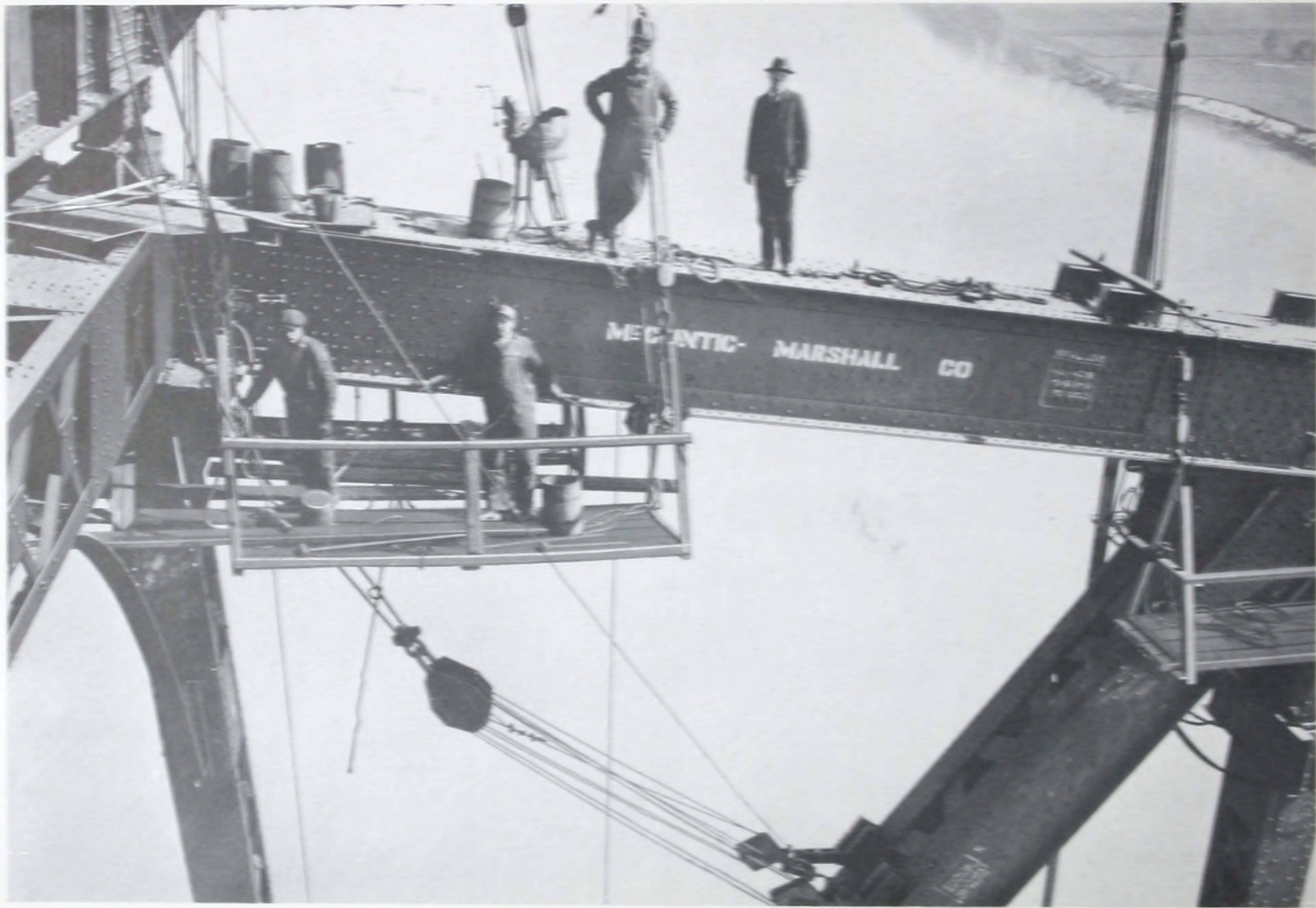
KENTUCKY SPAN—Steel cable falls used to connect main diagonal to top chord gusset.
