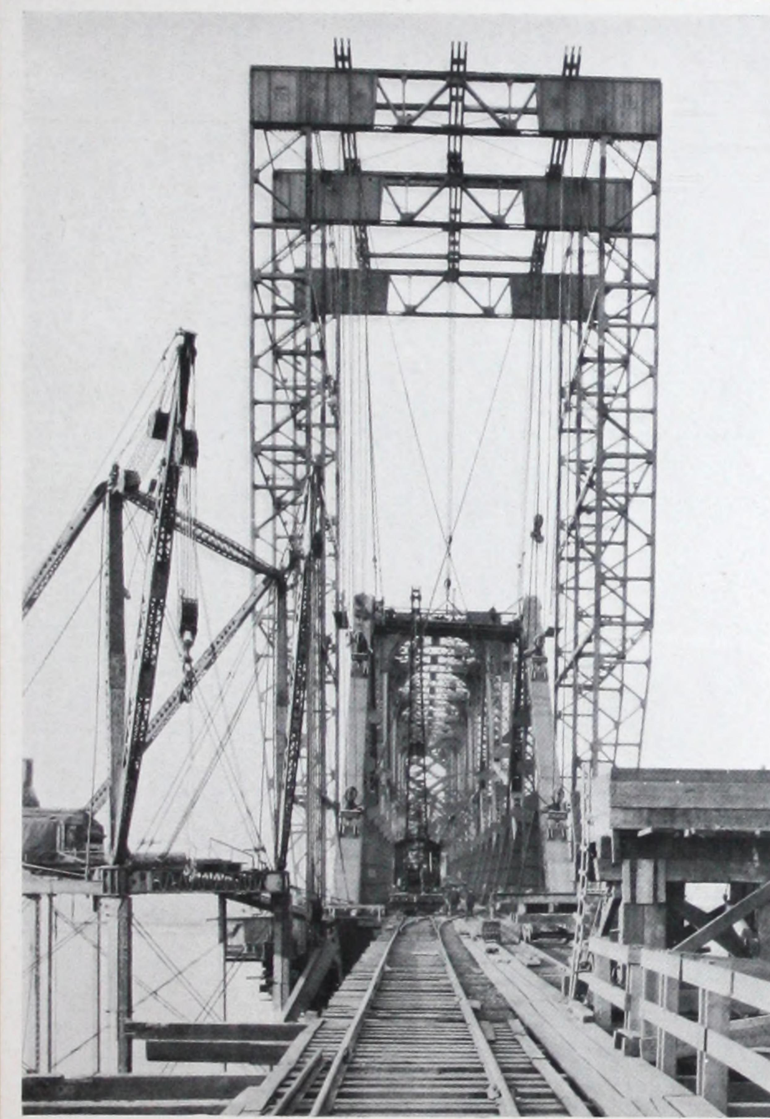
**OHIO SPAN**—Gantry traveler 160 ft. high setting the end posts; at left 2-boom lifting tower used to hoist steel from storage yard to bridge deck.
