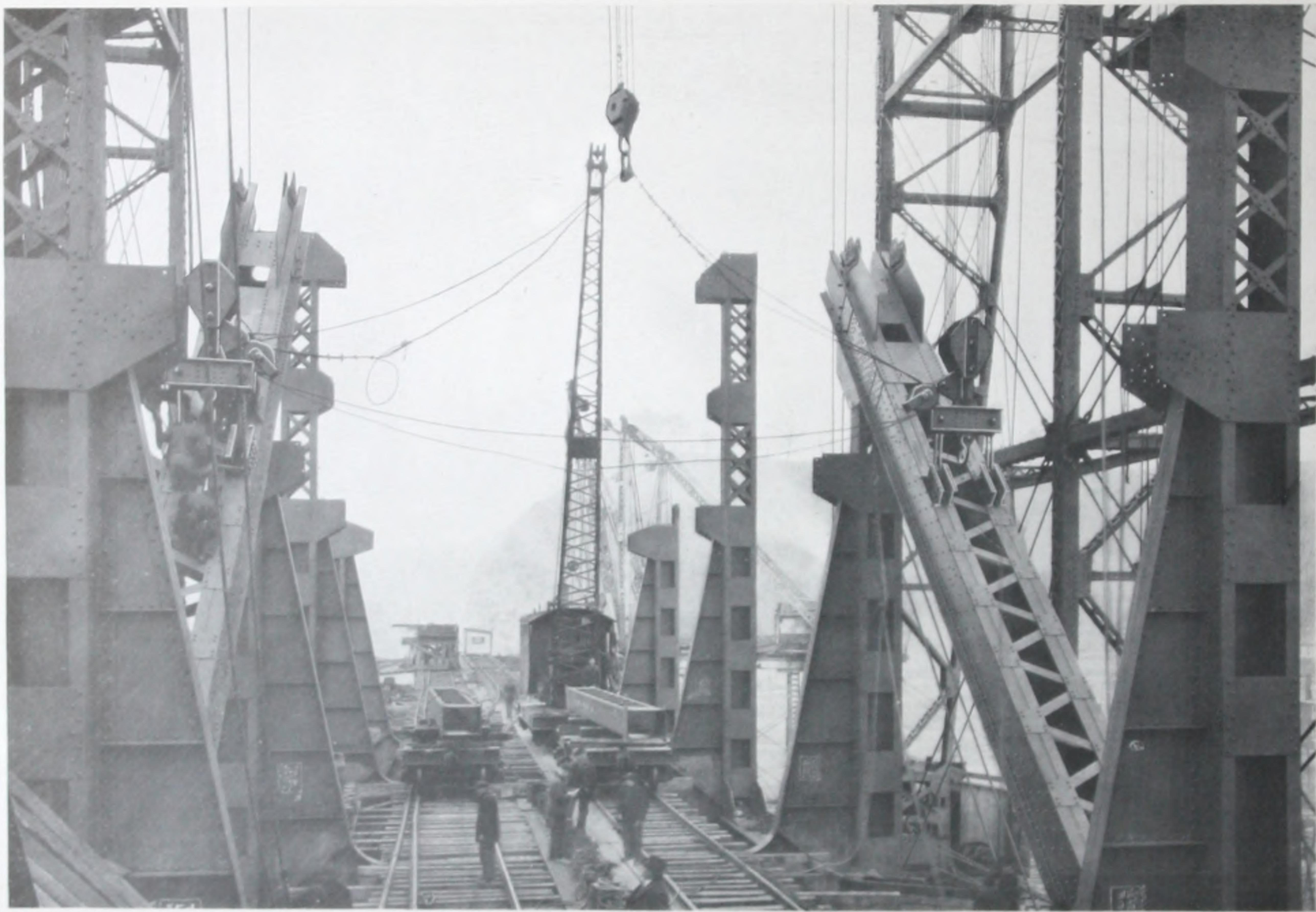
OHIO SPAN—Showing special lifting devices used on all main members.
