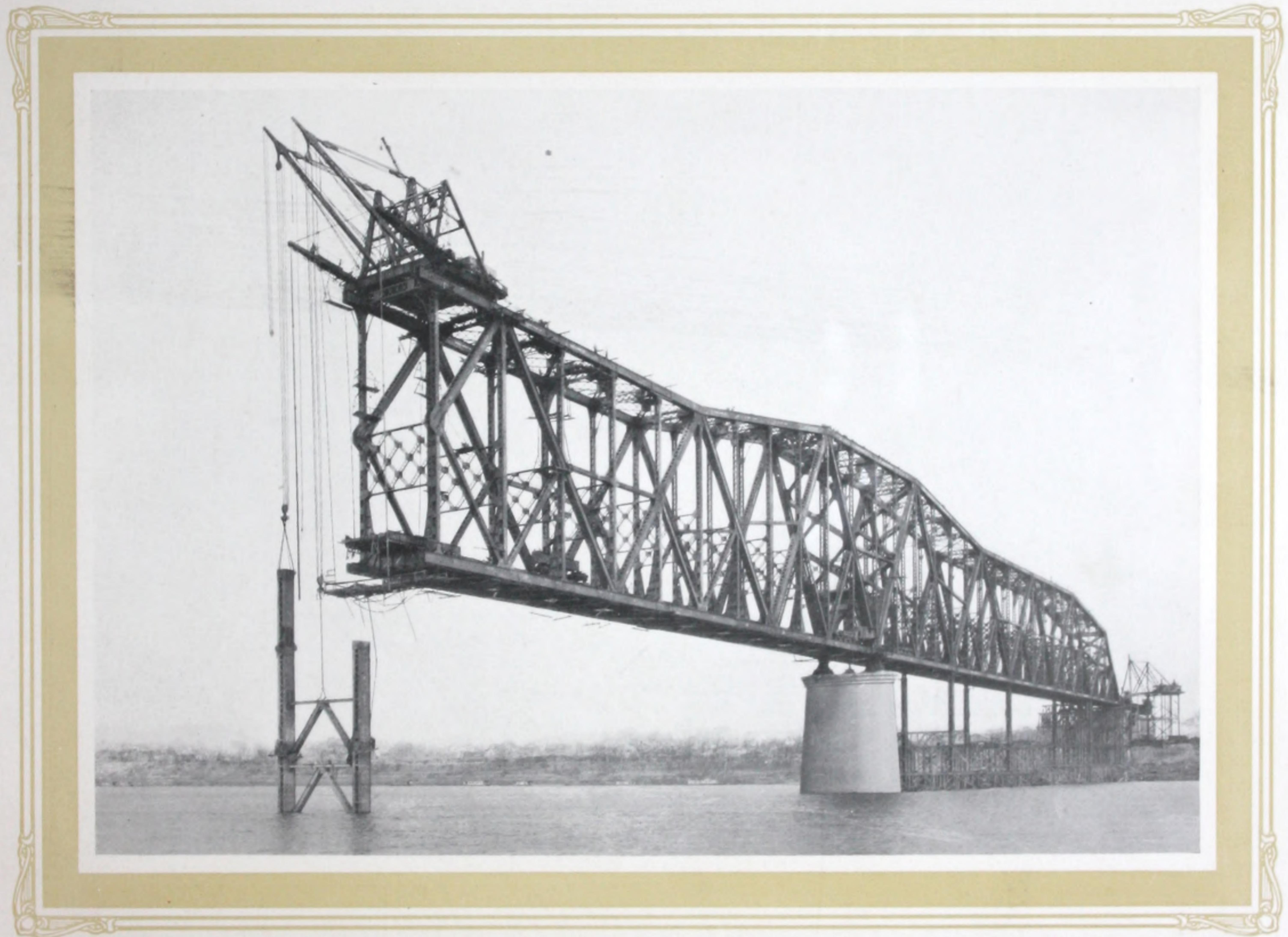
KENTUCKY SPAN—Erecting steel falsework bent at L-8. Kentucky span cantilevered 426 ft. 3 in.
