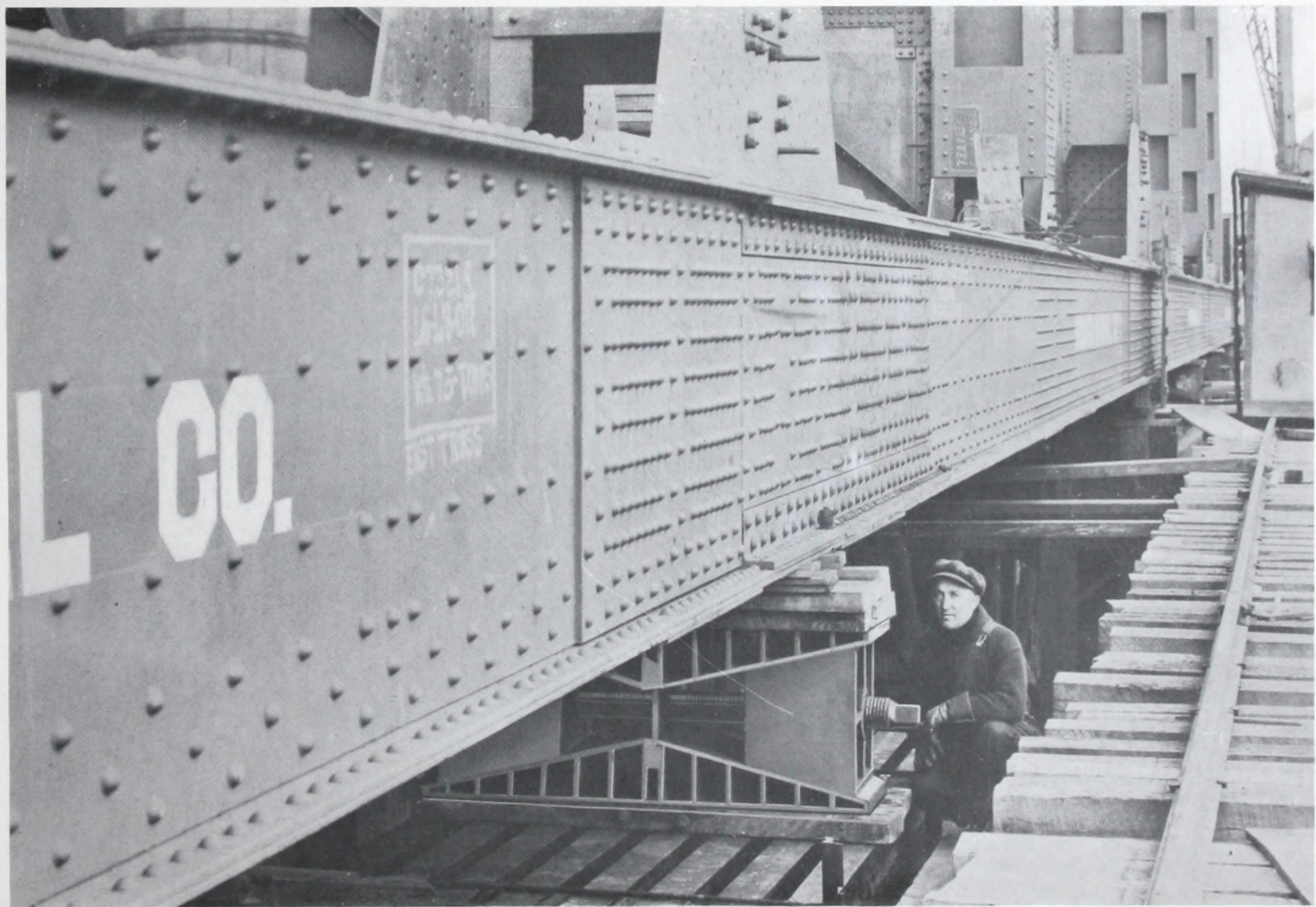
OHIO SPAN—Showing wedge jacks supporting lower chord on top of timber falsework towers.
