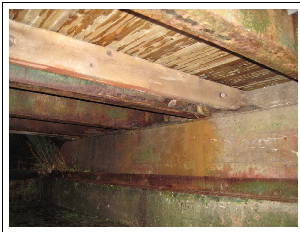
Photo 11 Severe Corrosion of Stringers at East Abutment
