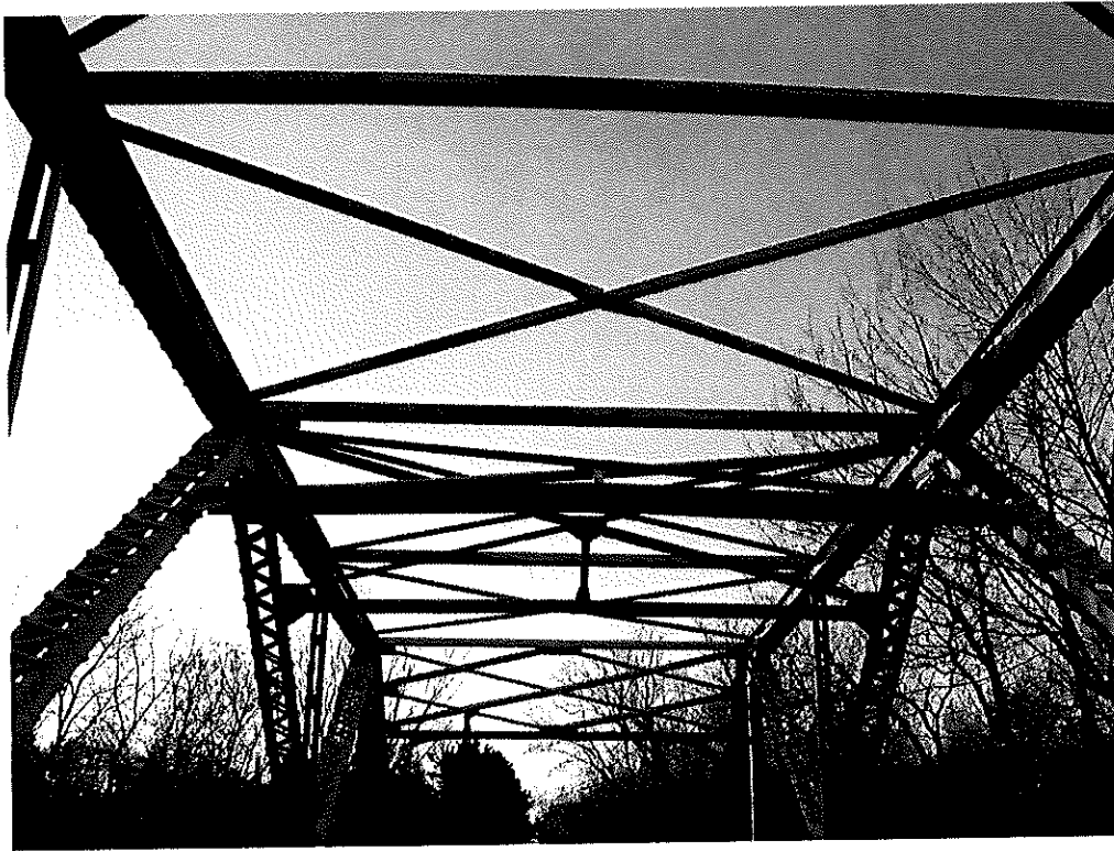
Plate 13 View of the Pattern of Construction of the Superstructure to the South from the North Edge of Collingwood Street Bridge
