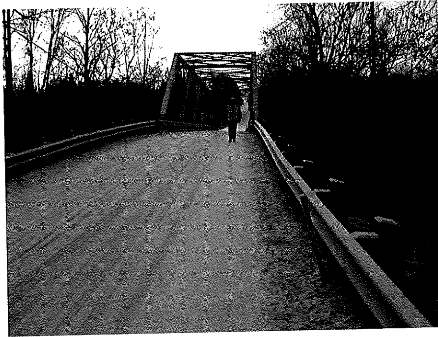
Plate 1 Collingwood Street Bridge (Bridge #000141) looking South from the North Approach
