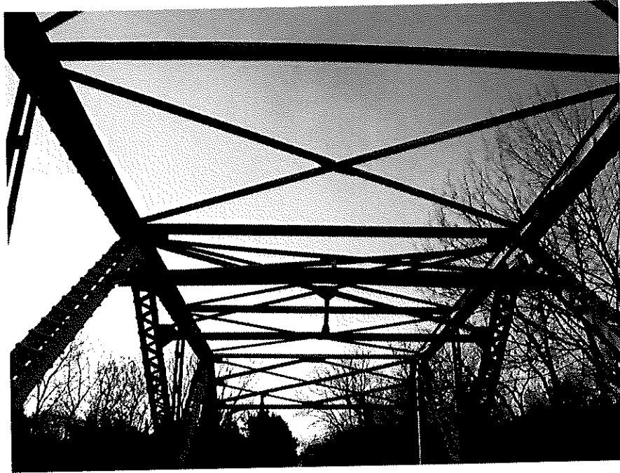
Plate 13 View of the Pattern of Construction of the Superstructure to the South from the North Edge of Collingwood Street Bridge
