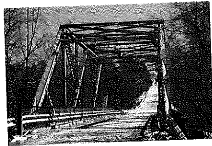
Collingwood Street Bridge Rehabilitation
