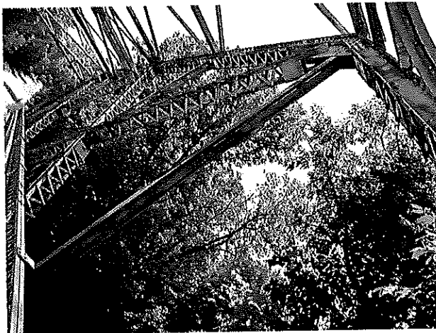
. Showing medium condition.
