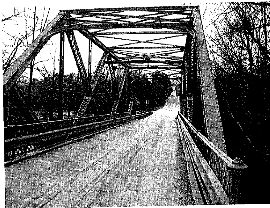
Plate 2 Collingwood Street Bridge (Bridge #000141) looking South from the North Edge of the Bridge
