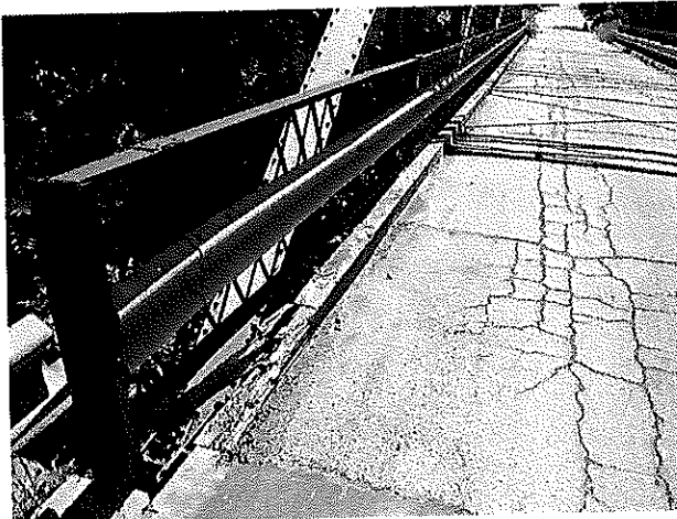
East Side. Showing severe deterioration.
