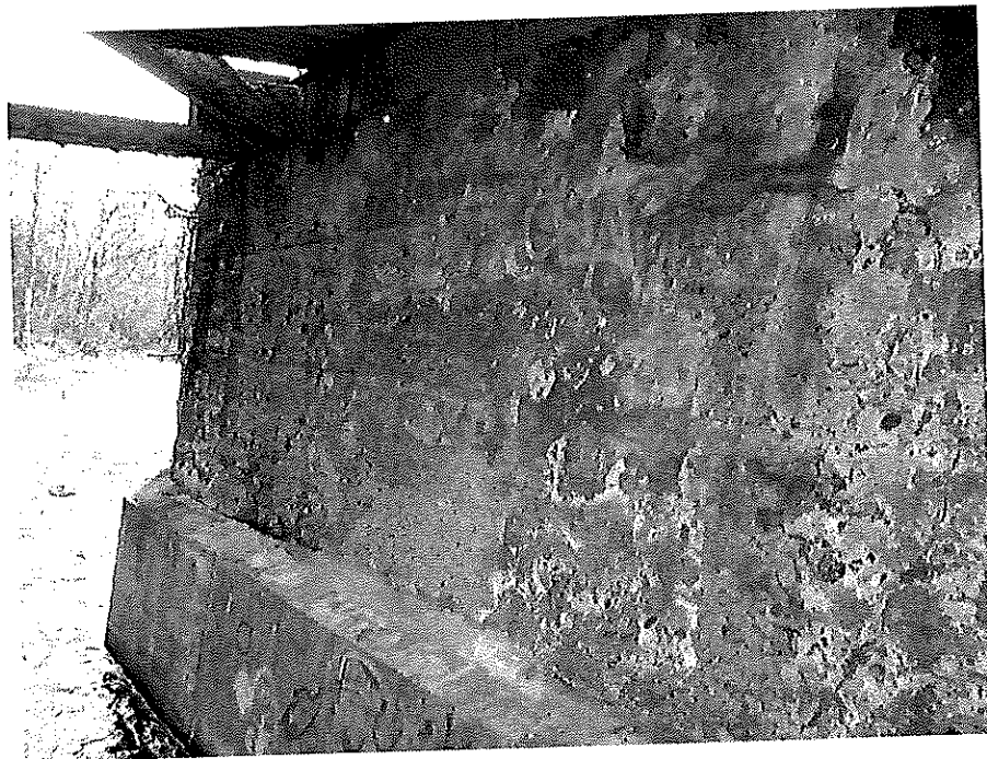
Plate 10 North Bank Abutment of Collingwood Street Bridge
