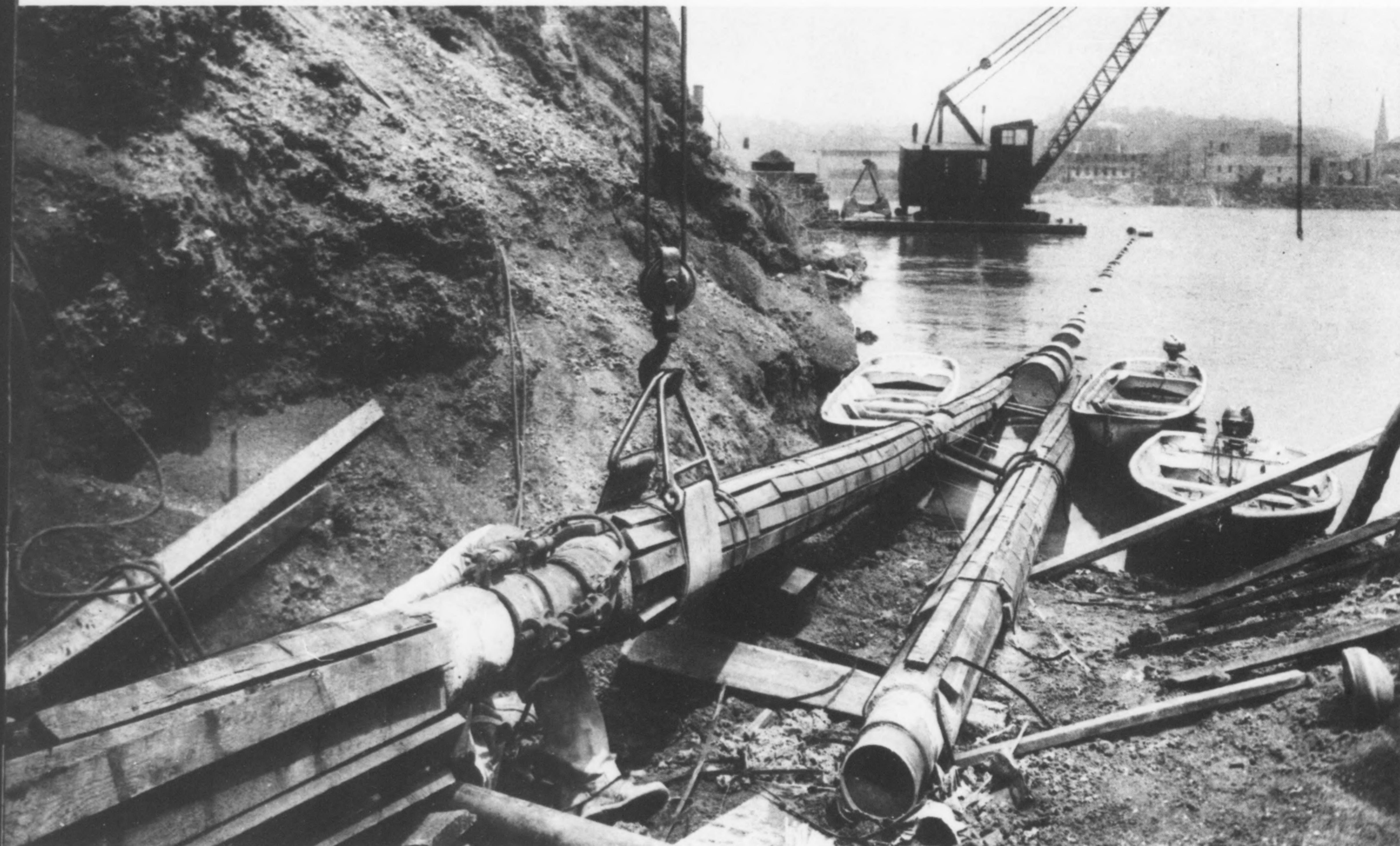
Preparing to weld pipe for Ohio River crossing. Pipe has a heavier wall to provide additional margin for burning in case of a line-to-ground fault in a river section.
