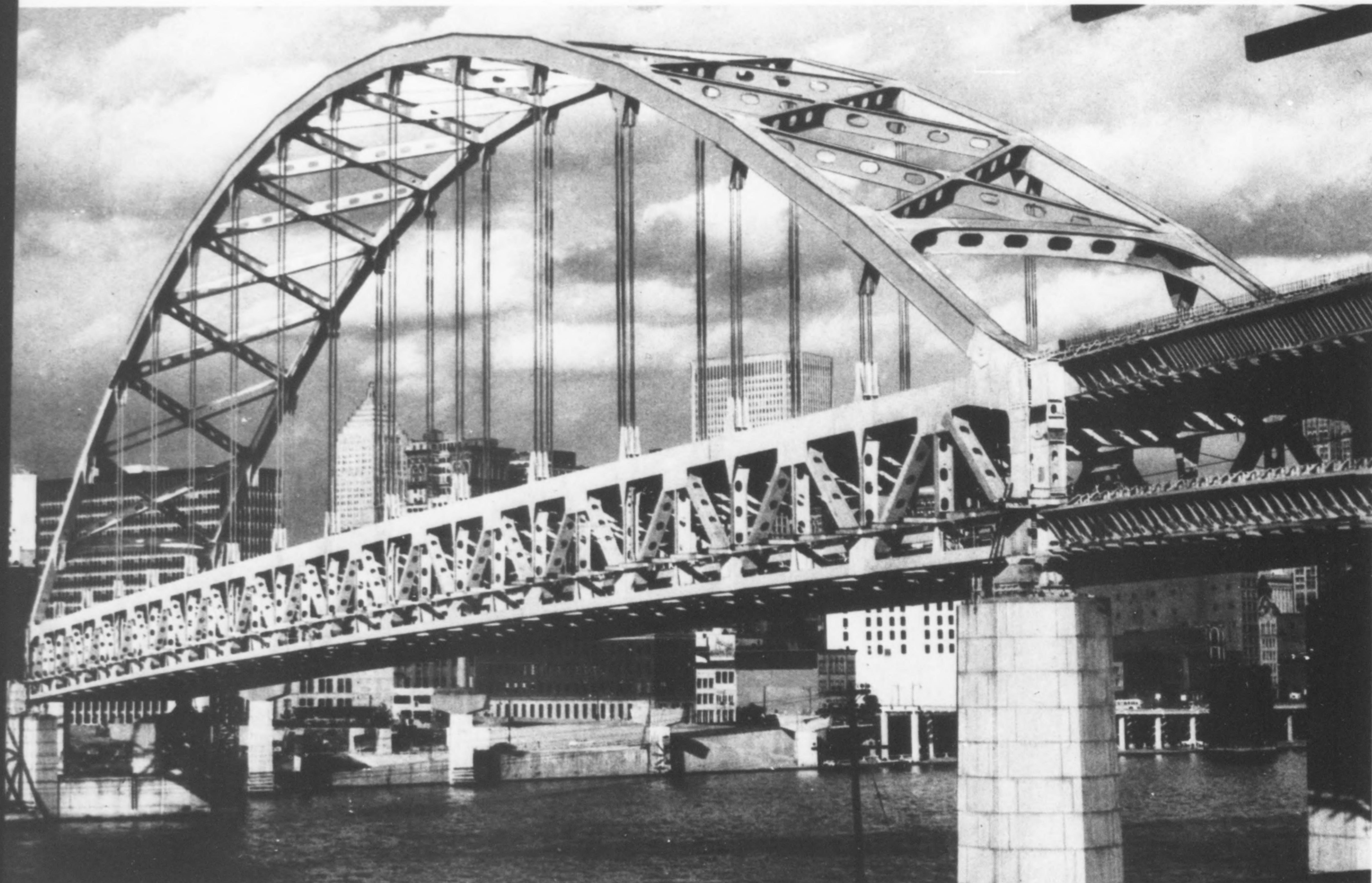
Pittsburgh's Fort Pitt Bridge was built with a steel with a reputation—USS MAN-TEN Brand High-Strength Steel. About 5,800 tons of MAN-TEN Steel were used in the 750-foot span. This steel is about 50% stronger than structural carbon steel and saves weight and money.
