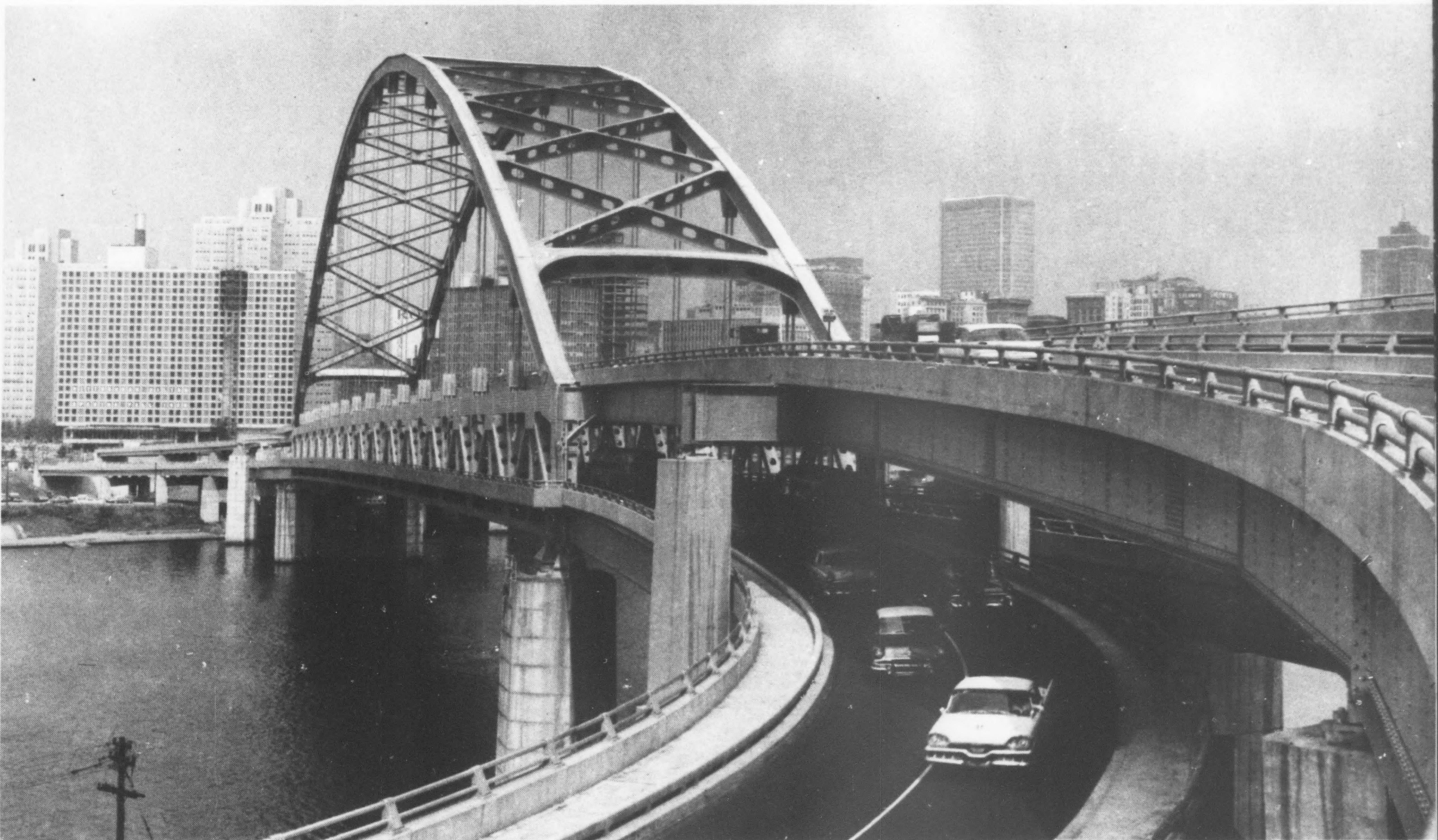
**New Gateway to the West—Fort Pitt Bridge** carries the Lincoln and Wm. Penn highways across the Monongahela River at the Point. It is an 8-lane, double-deck structure with a tied-arch span 752 feet long. Erected by American Bridge Division. The Fort Duquesne Bridge, of similar design, is under construction over the Allegheny River.
