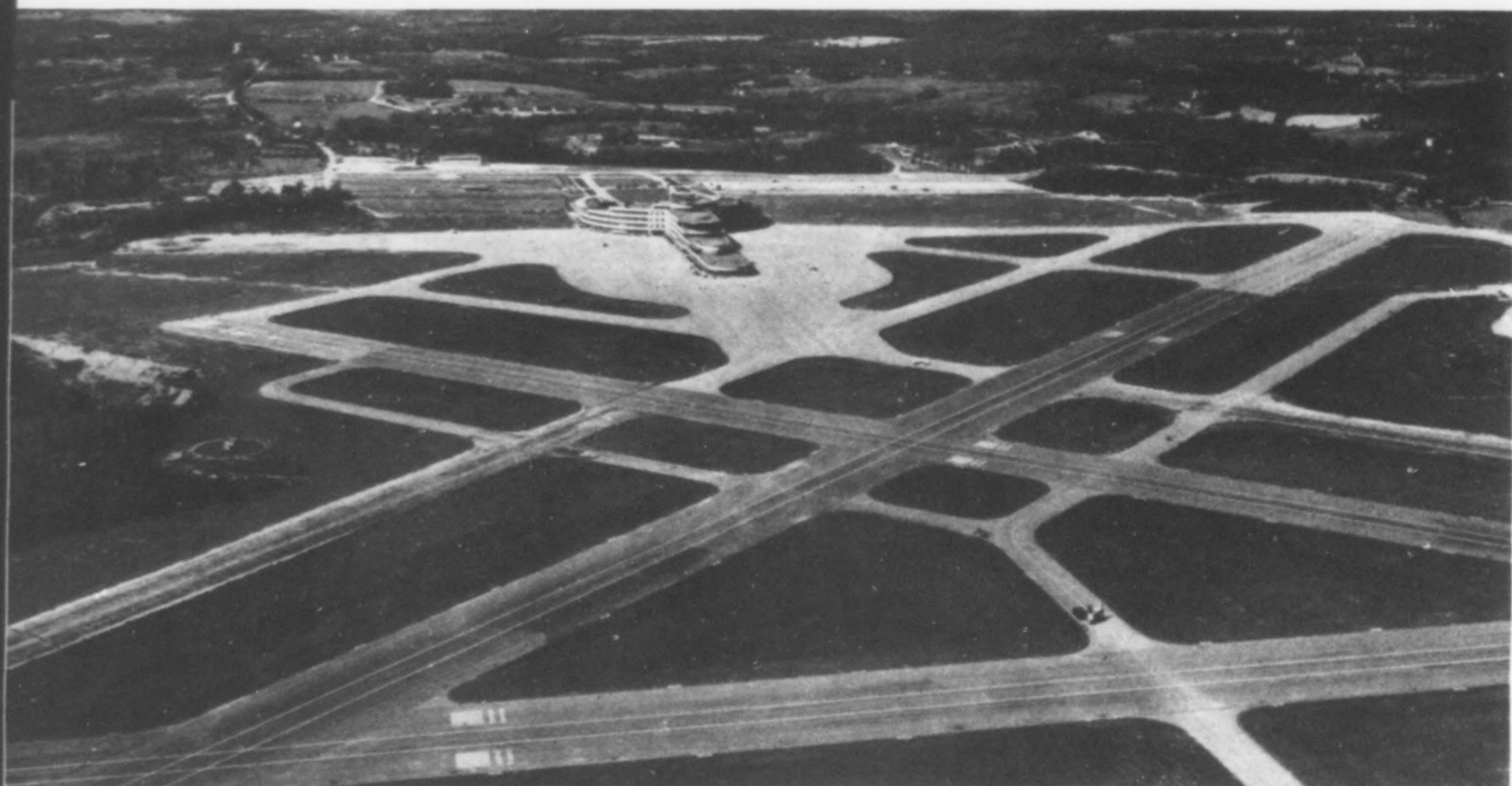
**Greater Pittsburgh Airport.** Almost 1,000,000 square yards of concrete and bituminous paving included air-cooled blast furnace slag as the coarse aggregate where concrete failure could not be tolerated.
