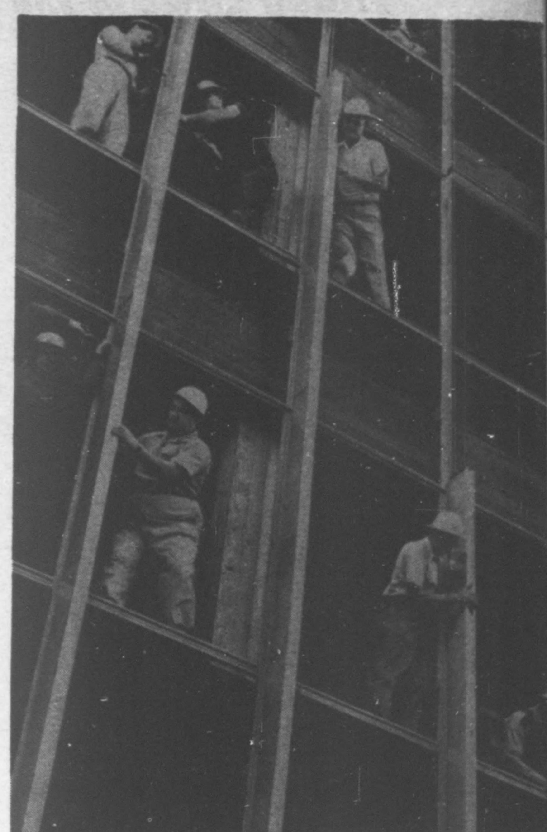
**Stainless steel mullions, fastened to zinc-coated steel framing, accent vertical in Gateway building.**
