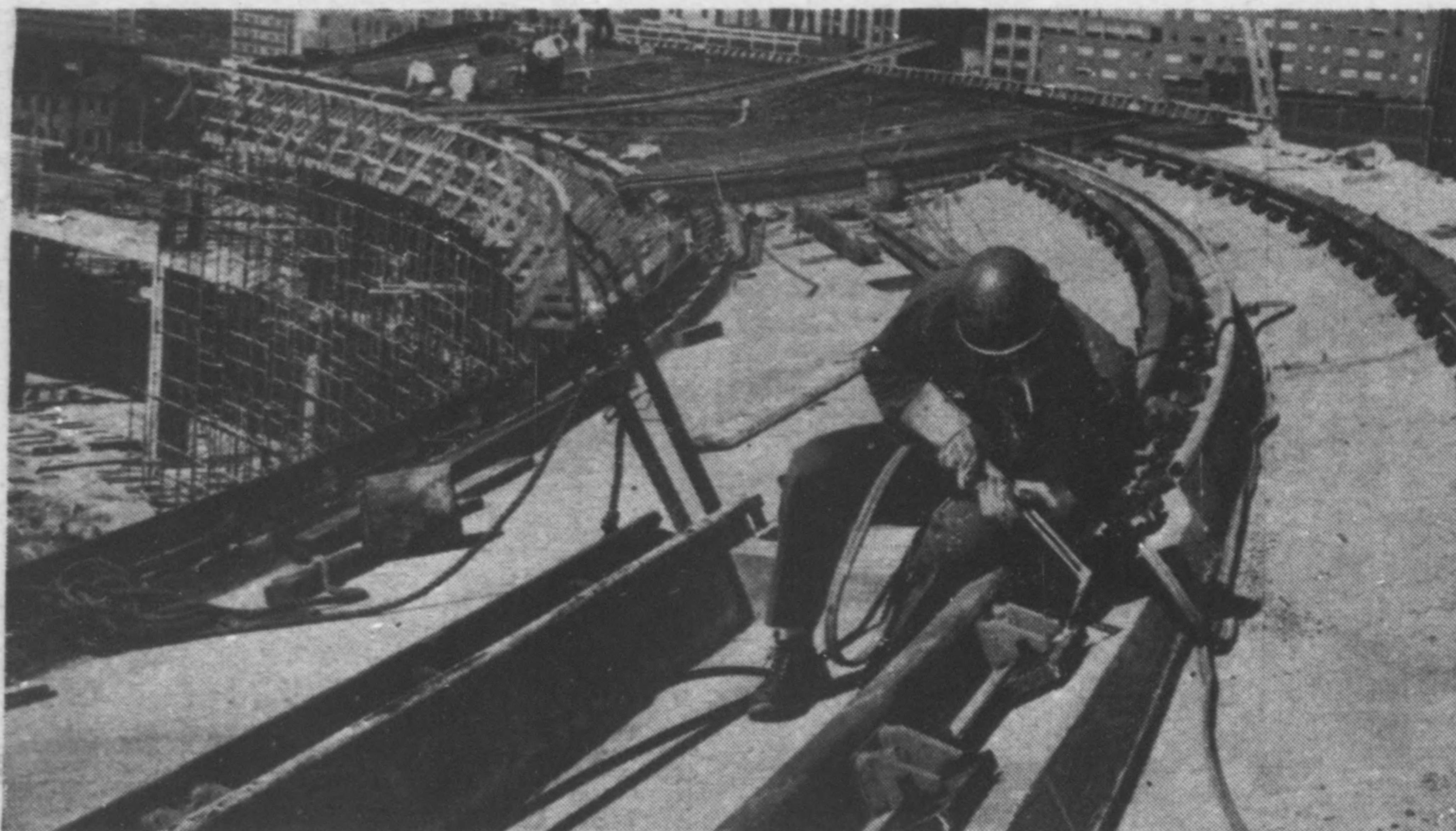
**WELDER** anchors rail clip to base plates. Neoprene gaskets at bottom of movable roof will be pressed against a pipe-top plate (right) to seal out weather.
