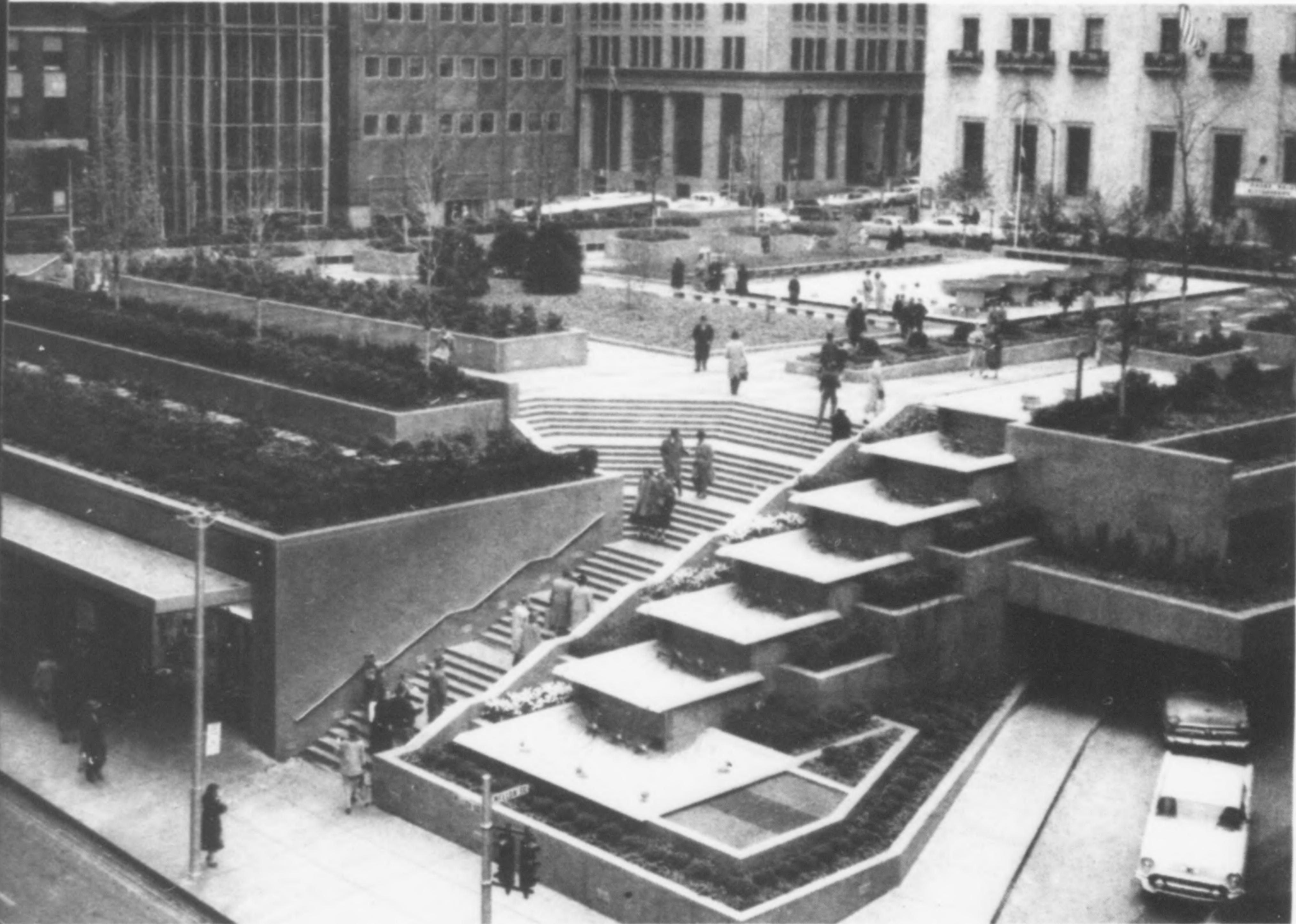
**Mellon Square Park** and a six-floor underground parking garage. Built with reinforced concrete in which all the coarse aggregate was USS Blast Furnace Slag.
