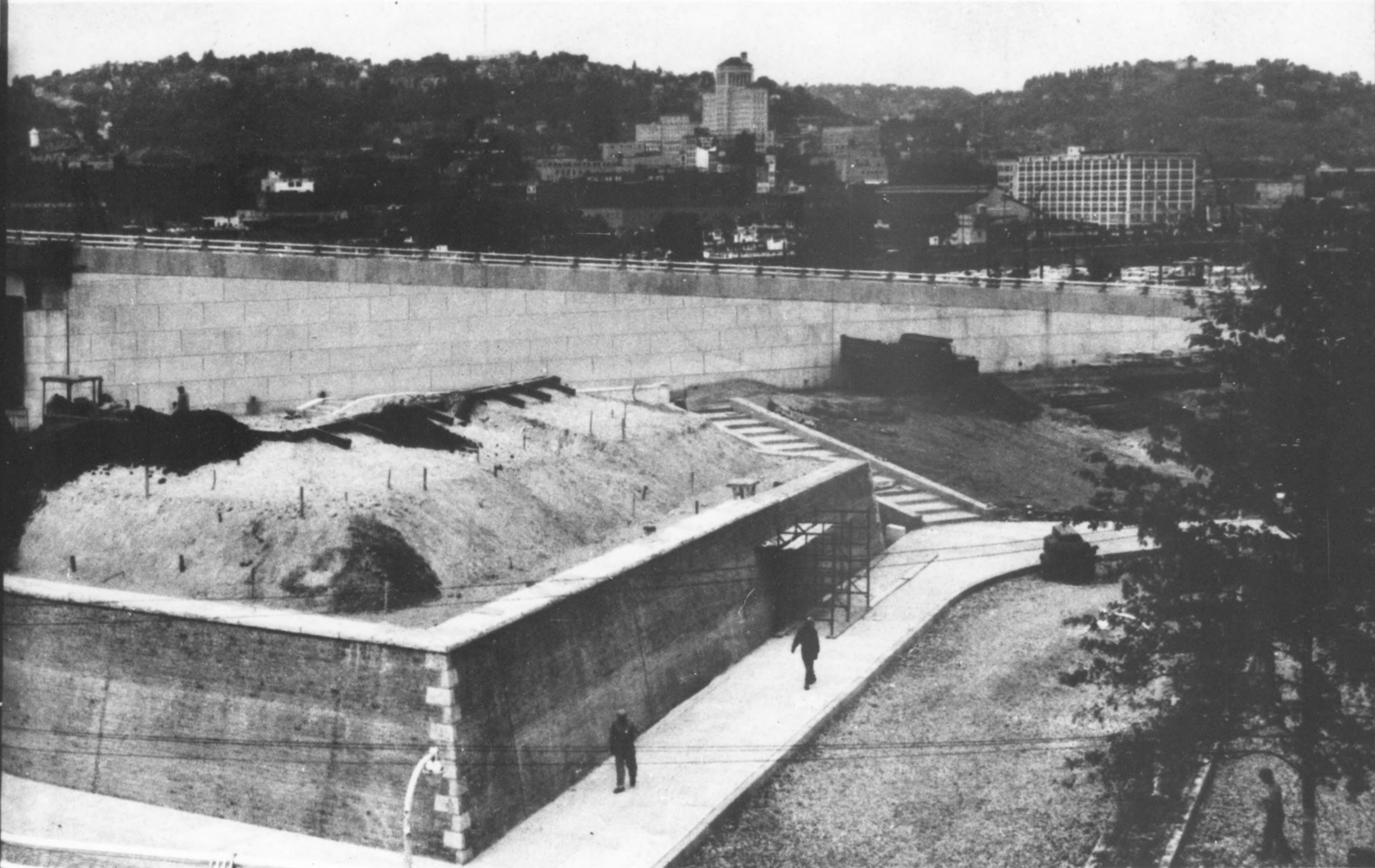
**Fort Pitt Restoration** at the historic point where the Monongahela and Allegheny Rivers merge to form the Ohio. 10,000 tons of USS Granulated Blast Furnace Slag were used as permanent fill in the flag bastion to a depth of 20 feet.
