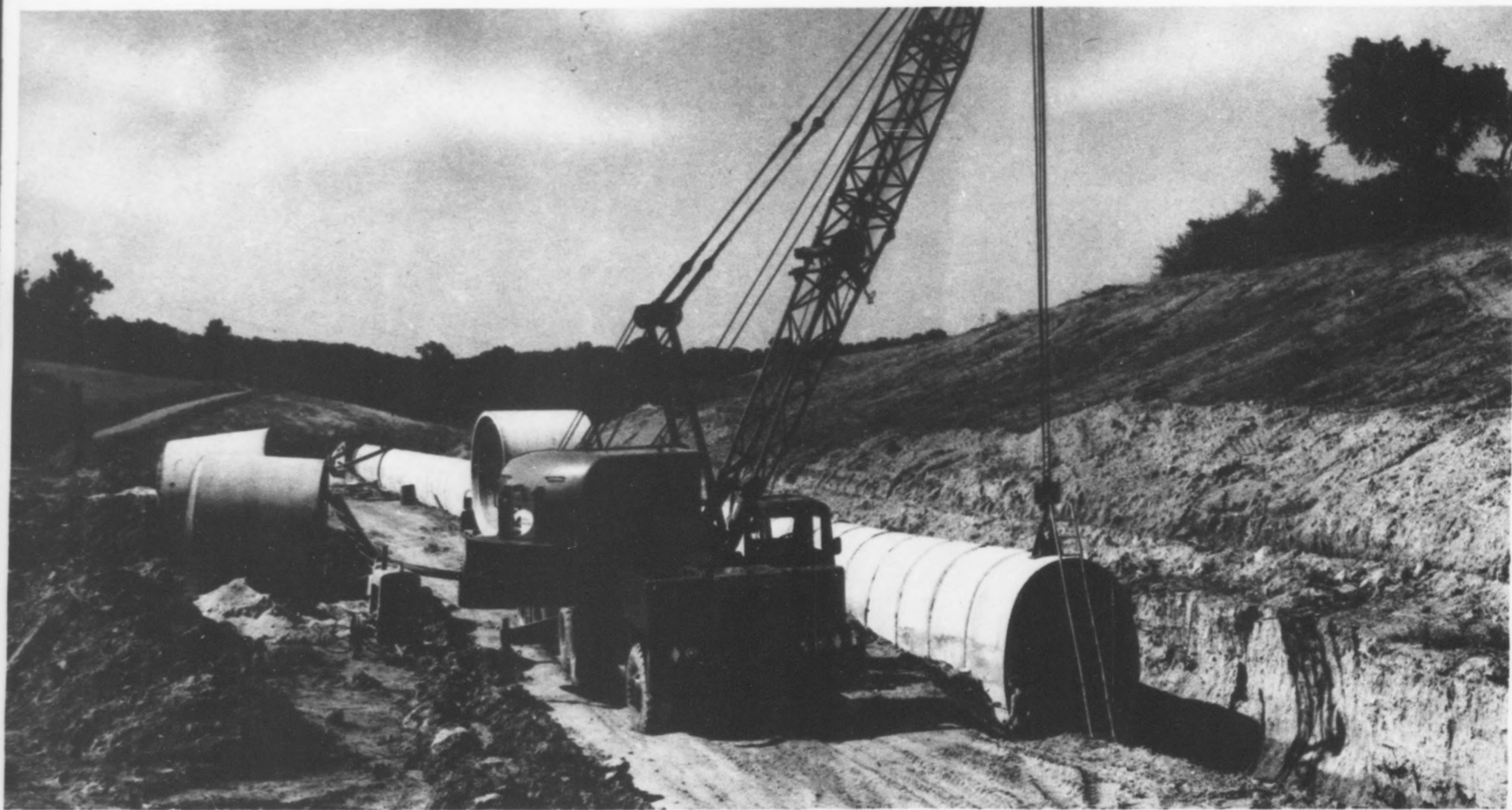
**Concrete culvert pipe for the jet-plane runway is reinforced with heavy-duty USS AMERICAN Welded Wire Fabric. Triple cages of reinforcing provide extra strength for supporting a 90-foot fill. Concrete pipe reinforced with steel means long life, great strength and durability, plus low maintenance cost.**
