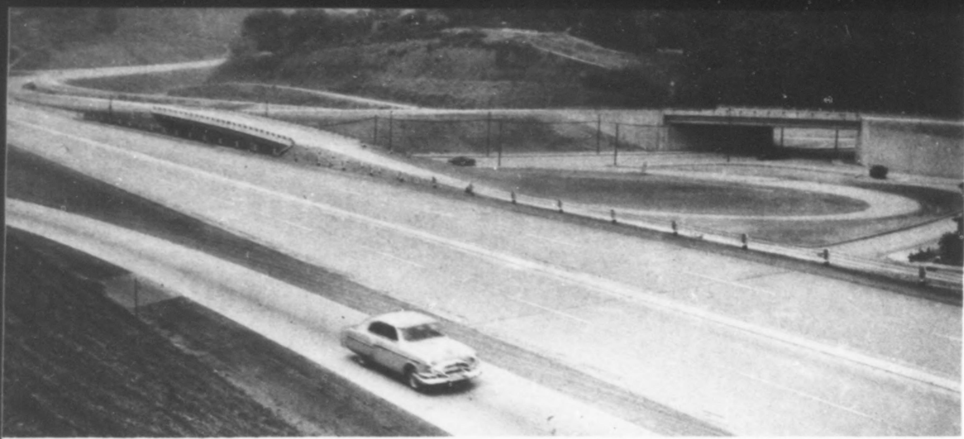
**Penn-Lincoln Parkway** contains five miles of non-skid slag concrete pavement, requiring 125,000 tons of slag aggregate. Another 143,000 tons were used for the sub-base to stabilize pavement.
