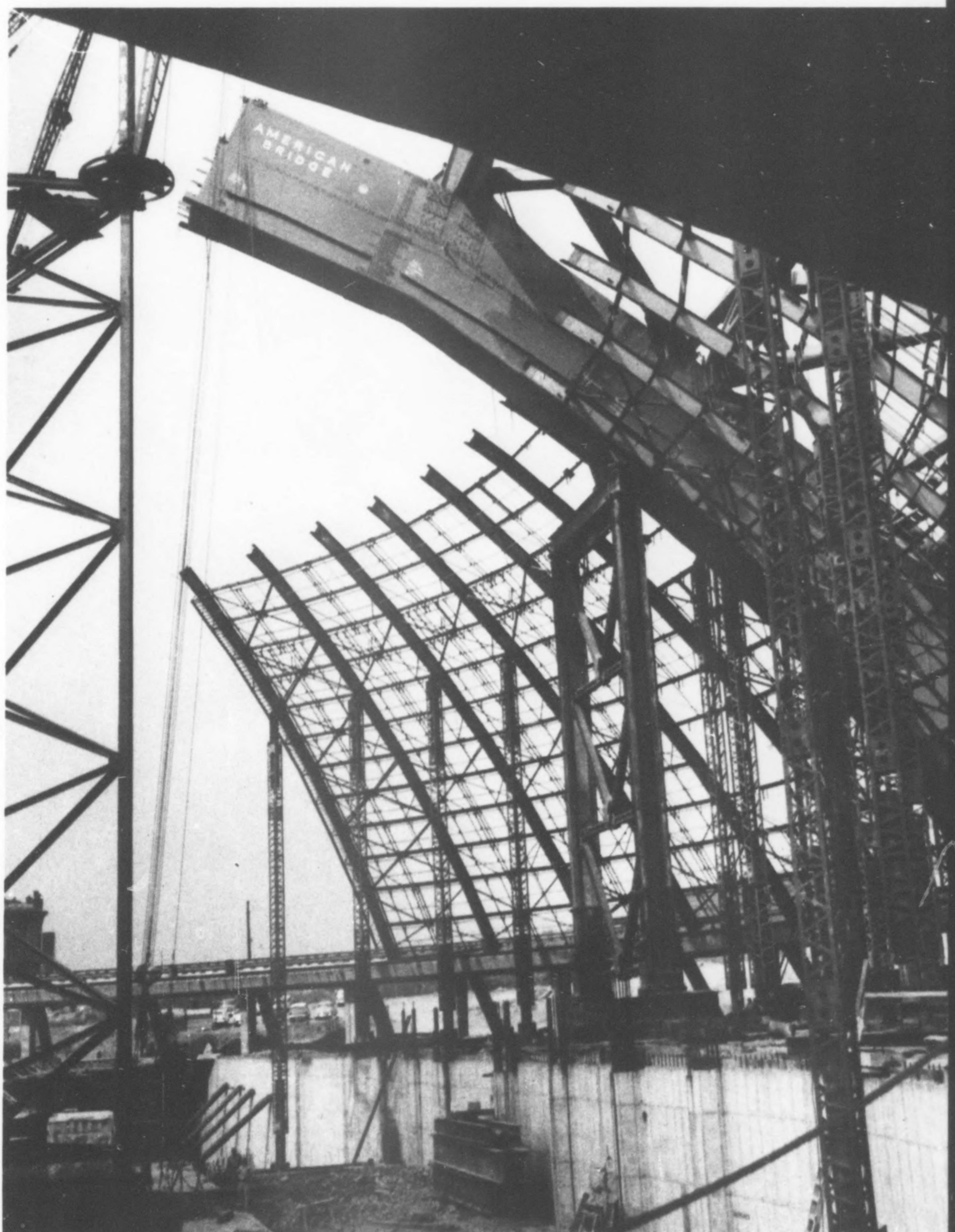
**USS Structural Steel** framework for the new Pittsburgh Auditorium. 3,425 tons are being used including USS TRI-TEN High-Strength, Low-Alloy Steel for members where extra strength is needed.
