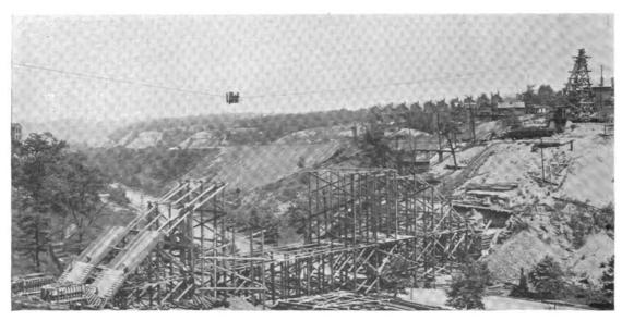
FIG. 1—THE LARIMER BRIDGE, JULY 15, 1911. SHOWING THE WORK ON THE TIMBER FALSEWORK.
