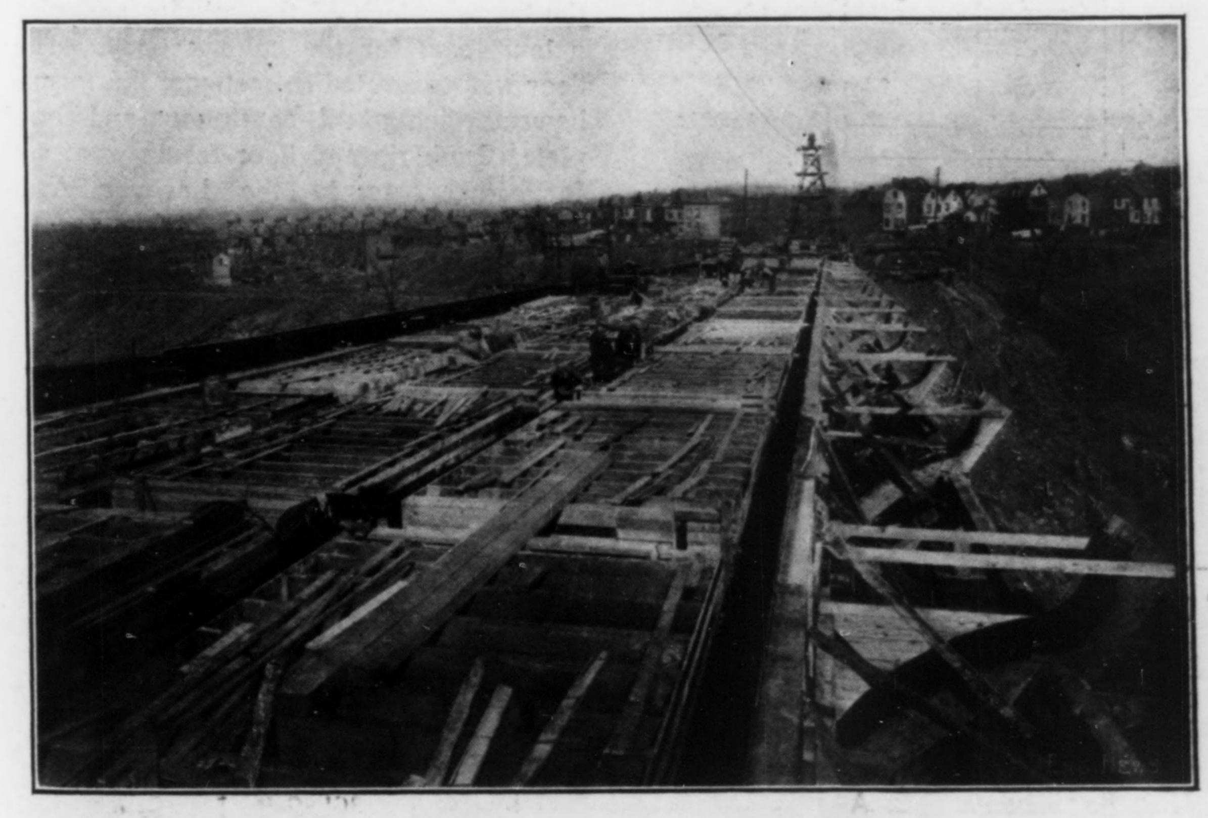
FIG. 11. LARIMER AVE. ARCH: FORMS FOR FLOOR FRAMING AND SLAB (MAR. 18, 1912)
