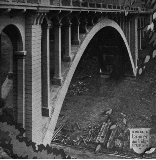
The pavement has a thickness of five inches and a width of twenty-six feet over all. There is a curb, six inches high and five inches thick, built on the pavement and anchored to it with steel loops every five feet. The reinforcement used is American Steel & Wire Co.'s No. 7 triangle mesh. There are expansion joints every thirty-three feet, protected with Baker steel plates, the joint being filled with tar.
