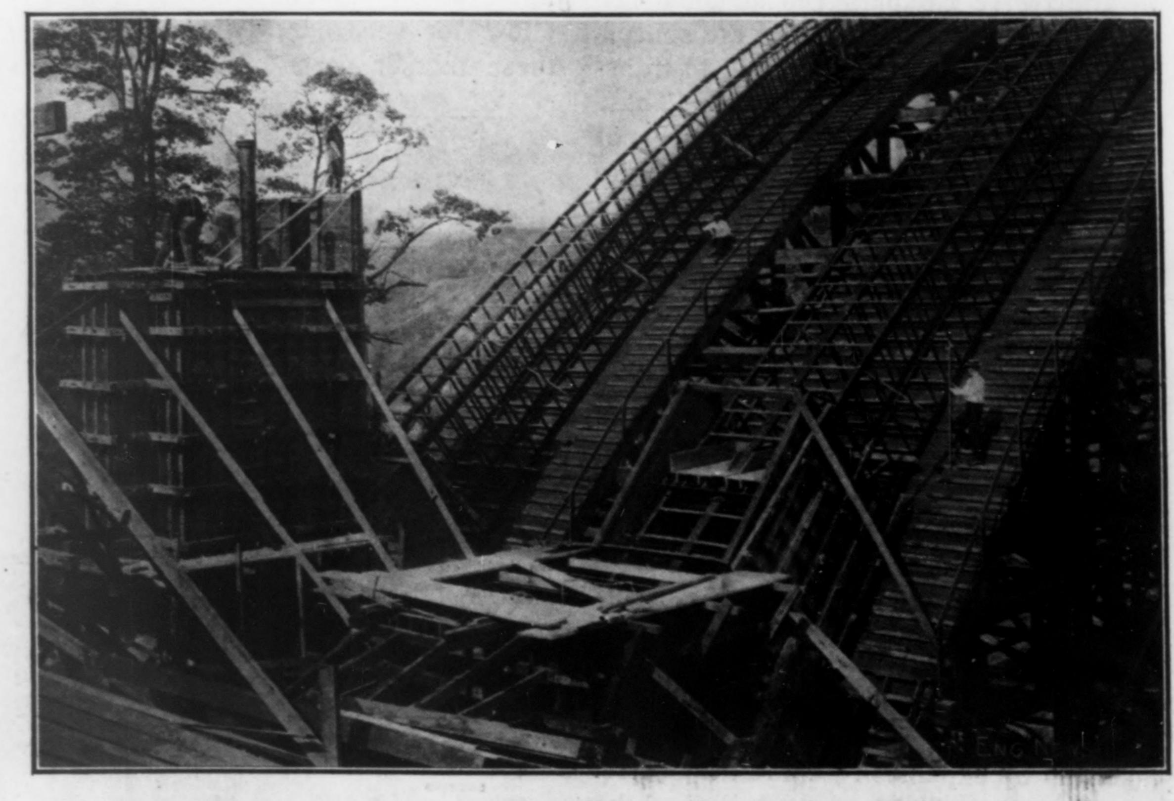
FIG. 8. LARIMER AVE. ARCH CENTERING, WITH RIB REINFORCING IN PLACE, AND FORMS FOR PARTS OF PIERS AND RIBS (West main pier, looking northeast, Aug. 21, 1911).
