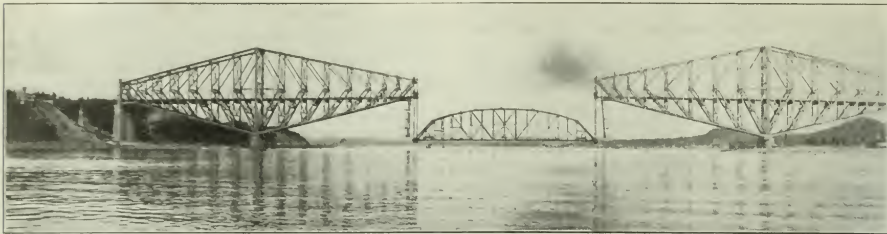
QUEBEC SUSPENDED SPAN HAD TO BE LIFTED 150 FEET AFTER IT HUNG CLEAR
