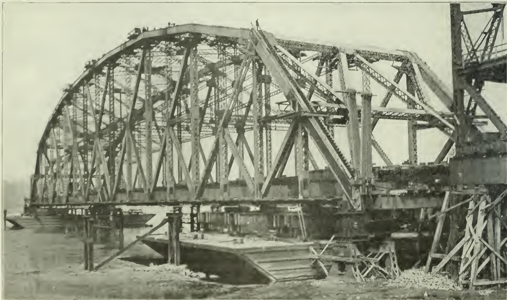
SUSPENDED SPAN OF QUEBEC BRIDGE JUST BEFORE IT WAS FLOATED TO PLACE AND RAISED THIS WEEK
