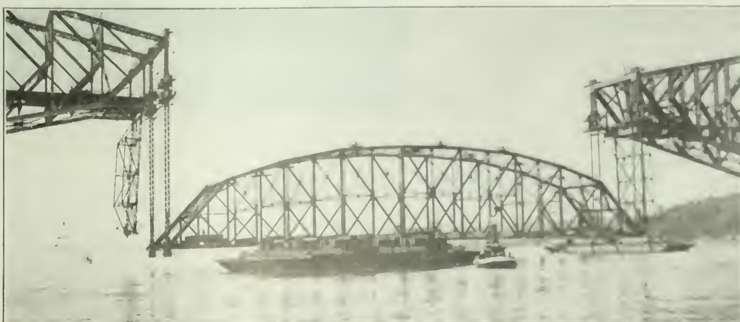
WHEN THE SUSPENDED SPAN WAS LIFTED FROM THE BOTTOM BY CABLES ATTACHED TO THE CANTILEVERS
