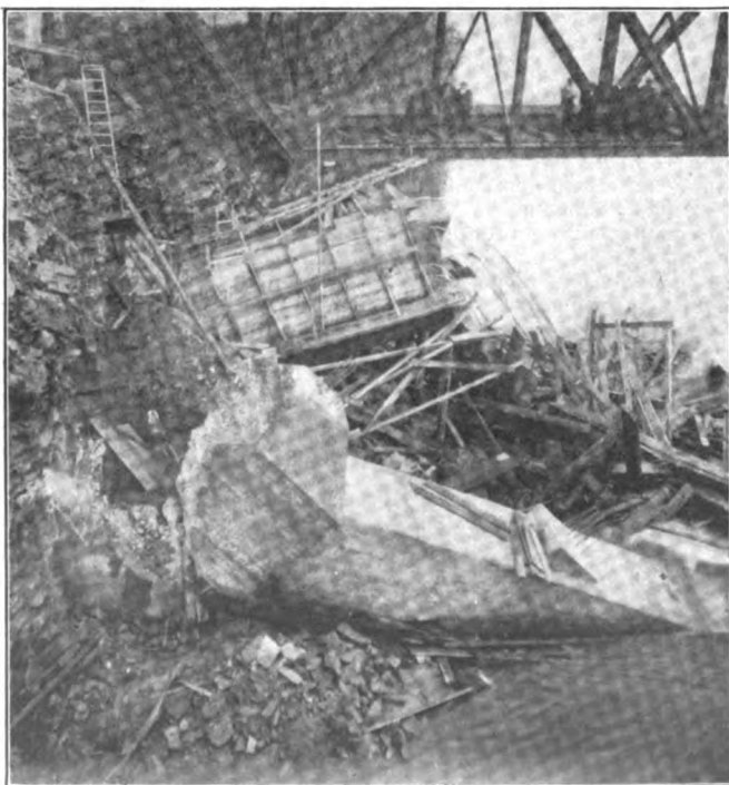
FIG. 1. POST ST. COLLAPSE AT EAST ABUTMENT
