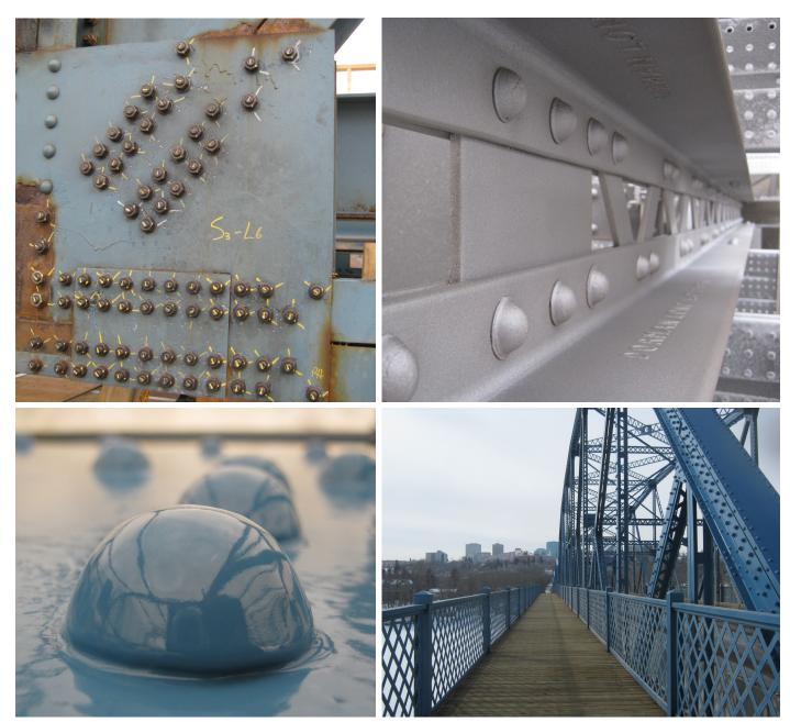
After completion of all truss strengthening and rivet replacement work, the entire superstructure was blast cleaned and recoated with a three-part organic zinc/epoxy/polyurethane system. This system is anticipated to last 25 years before overcoating is required.
