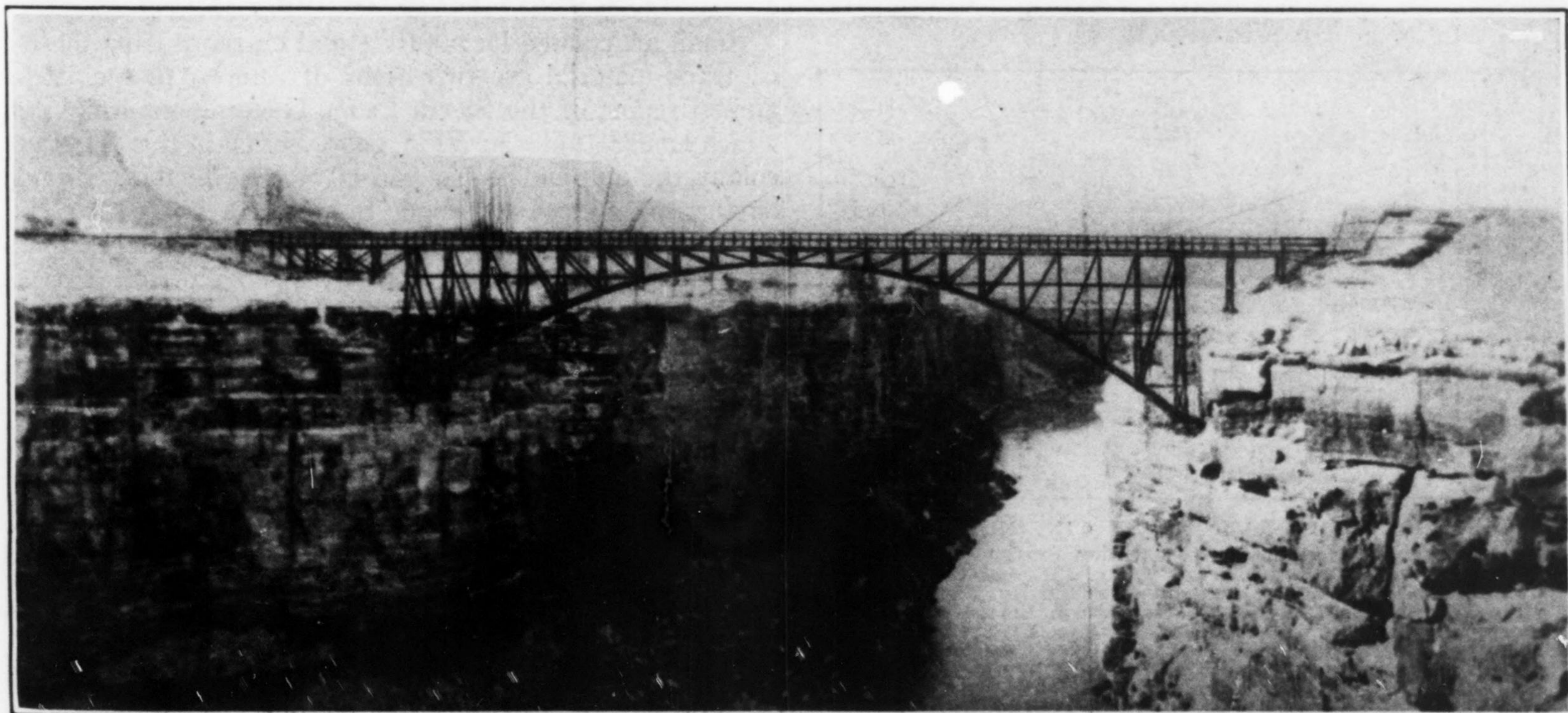
FIG. 2—STEEL ARCH HIGHWAY BRIDGE SPANNING GRAND CANYON Arch is 600 ft. long and crown is 467 ft. above the Colorado River.
