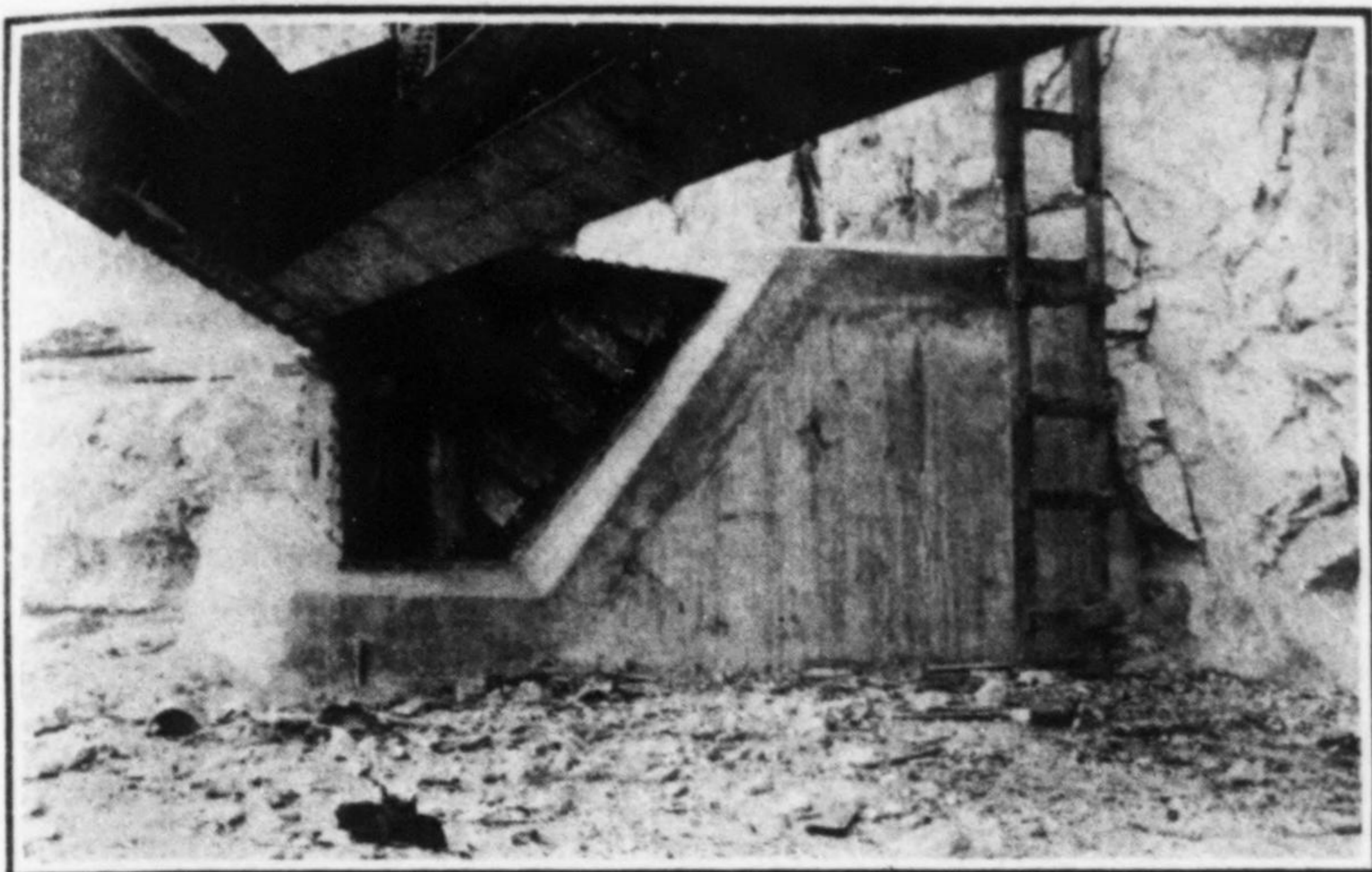
SHOE AND THRUST FOOTING AT NORTH ABUTMENT
