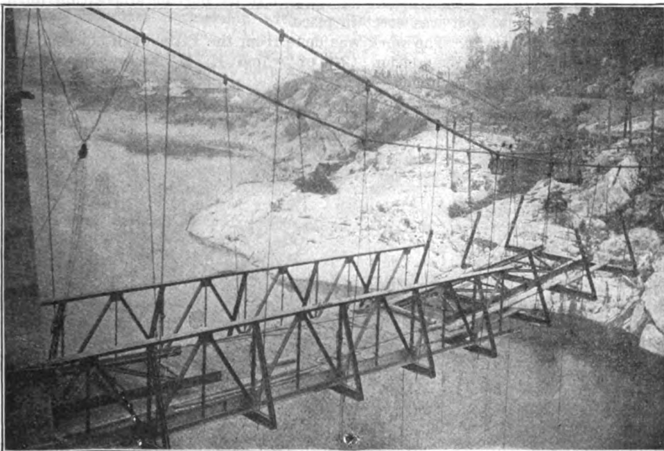
PLACING A THREE-PANEL SECTION OF SUSPENSION BRIDGE
