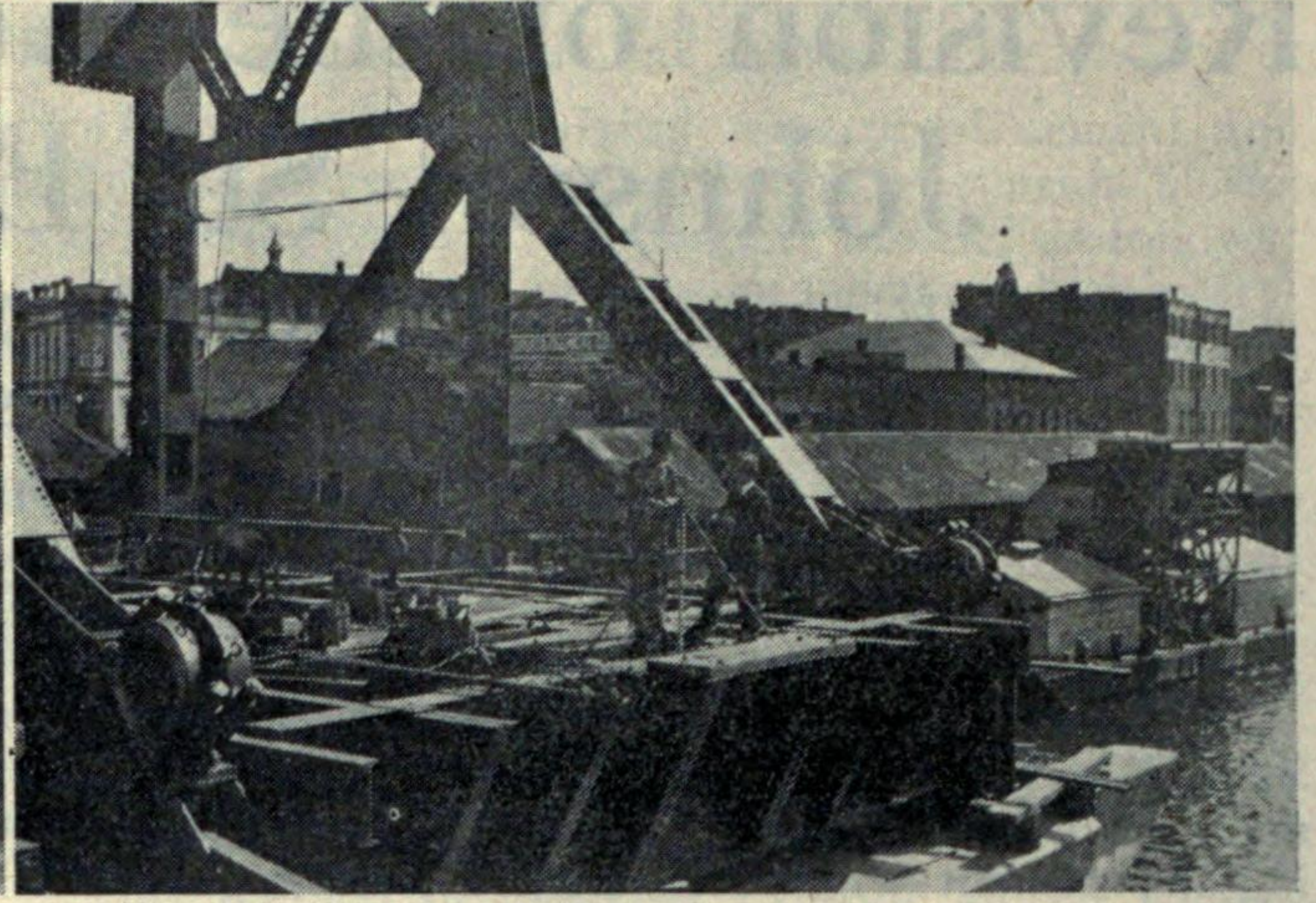
Setting main journals for bascule span
