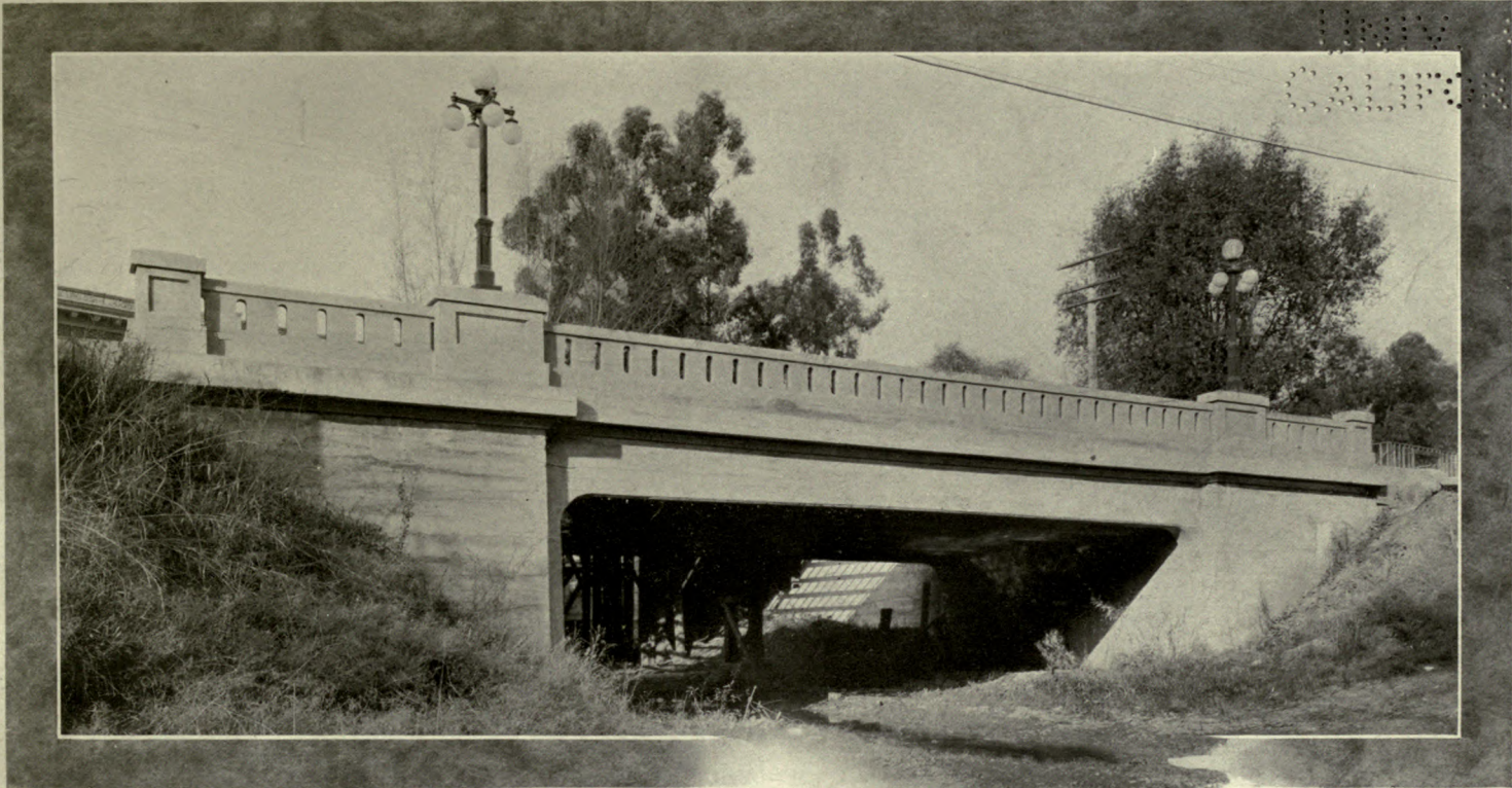
One of Marin County's artistic bridges; of the concrete girder type, simple and massive in design
