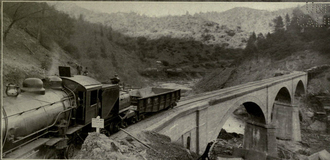
This bridge stands 75 feet above the river, and the skew or angle at which the bridge crosses the river is here plainly seen. Note the heavy Mallet compound engine, indicating the unusual demand upon the structure
