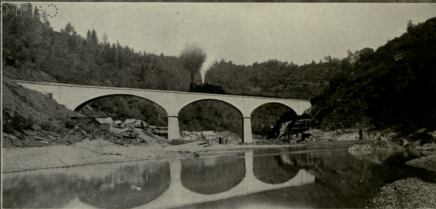
A 45 degree skew bridge, the railroad meeting each end on a 16 degree curve. Built on solid rock and carrying the heaviest locomotives hauling cars heavily laden with limestone
