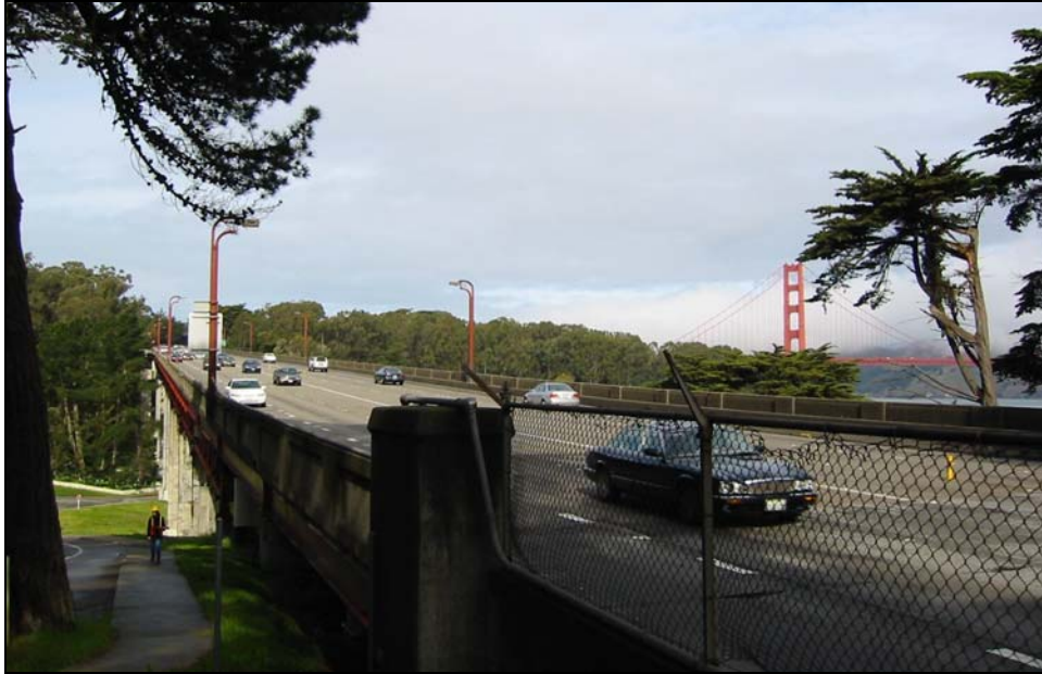
Doyle Drive (Presidio Viaduct) from east abutment, camera facing northwest.
