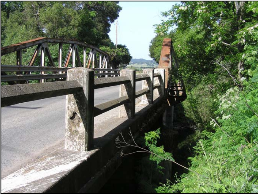
Figure 2. Cast concrete rails used on the approach.
