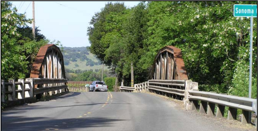
Figure 1. View across the bridge, facing west.
