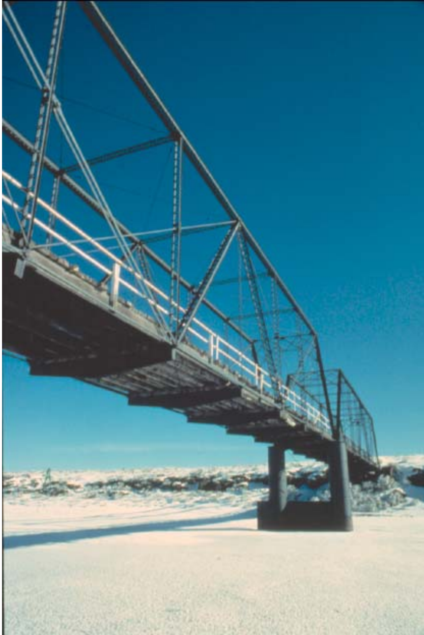
Costilla Crossing Bridge 5CN628-2(C)
