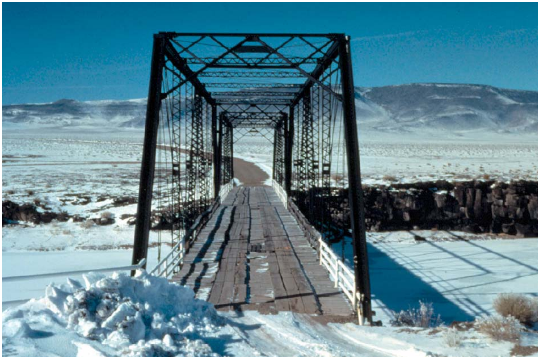
Costilla Crossing Bridge 5CN628-1(C)
