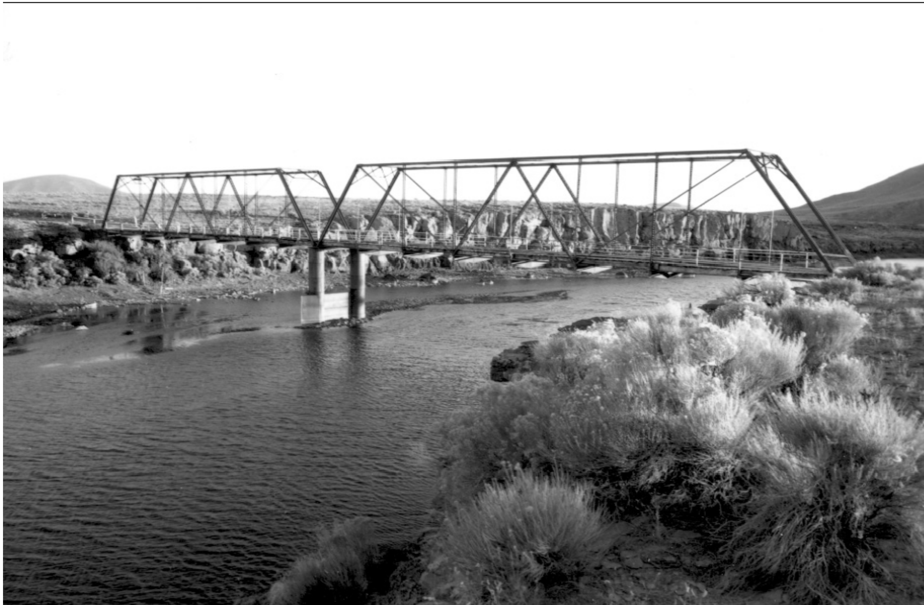
Costilla Crossing Bridge 5CN628-1
