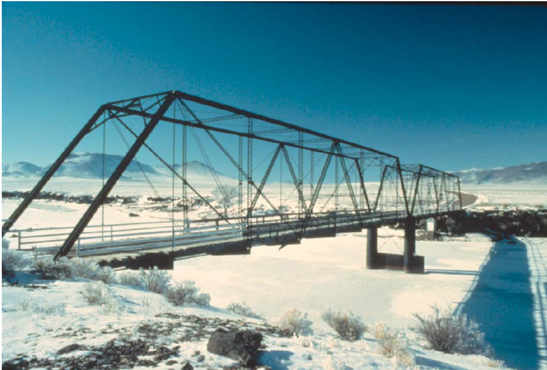
Costilla Crossing Bridge 5CN628-3(C)
