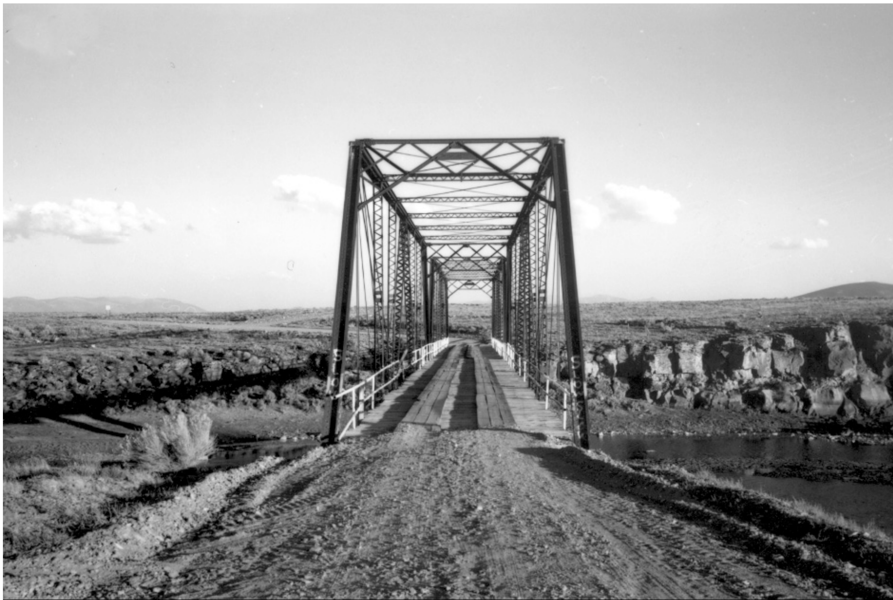
Costilla Crossing Bridge 5CN628-2
