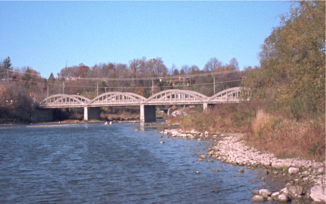
North West View
