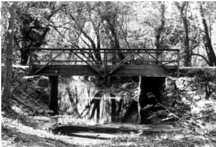
ABOVE: The Evanson Road bridge is one of three nearly identical extant late-19th-century Warren truss bridges in Delaware. Metal truss bridges were once common in New Castle County, with over 90 documented examples.
