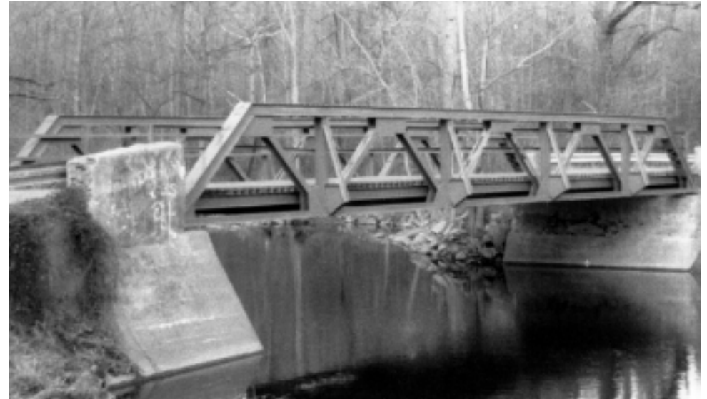
Warren pony truss bridges, such as the Thompson's Station Bridge erected in 1928, were a common highway bridge type from the first three decades of the 20th century.
