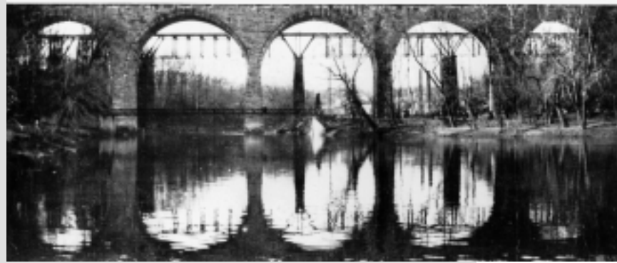
The B&O Railroad's Brandywine Viaduct, photographed shortly after it opened in 1910. In the background is the 1888 iron truss bridge it bypassed. In the foreground is a pedestrian suspension bridge that was used by workers walking to and from the mills that then lined the Brandywine Creek.
