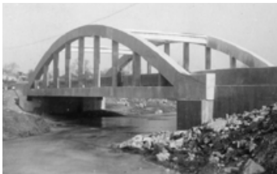
Construction photos for State Bridge NC-246.
