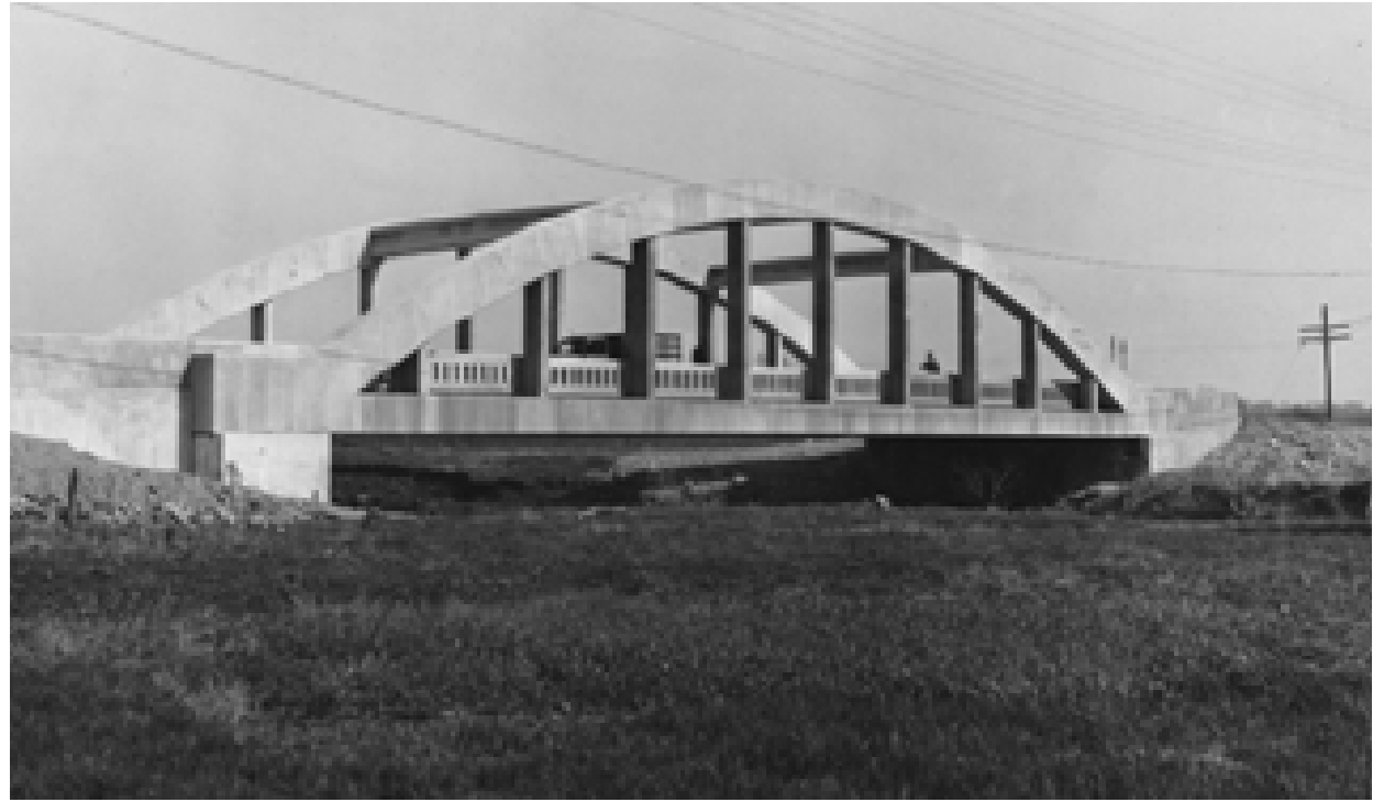
State Bridge NC-246, a reinforced concrete thru arch over White Clay and Mill creeks near Stanton, New Castle County, erected in 1940-1942.
