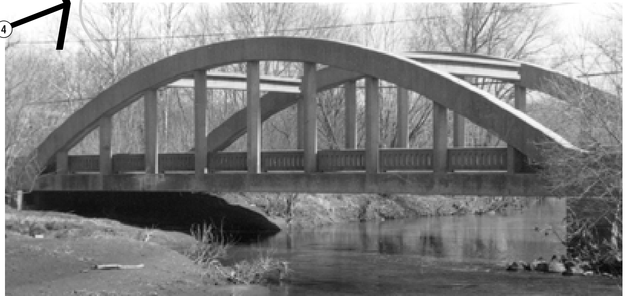
State Bridge NC-246 (1940-42) is Delaware's only reinforced concrete thru arch bridge.
