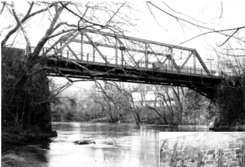
ABOVR: The main span of the Rising Sun Lane bridge, (above) erected in 1928, is a riveted steel Pratt thru truss, resting on massive granite abutments.
