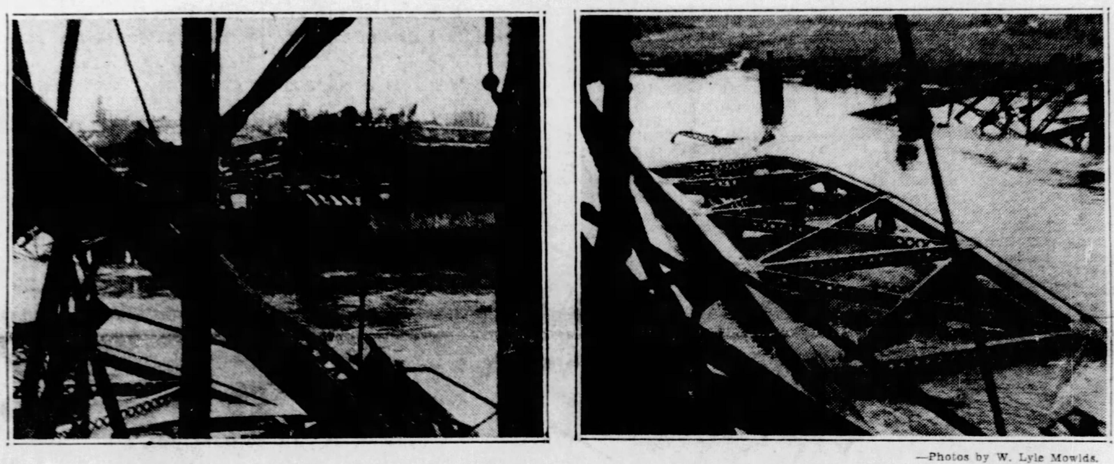
Engineers say it will take two or more weeks to remove the twisted structure of the bridge from the canal. The picture at the right shows the center span in the water. At the left is the Waukegan aground behind the bridge pilings.
