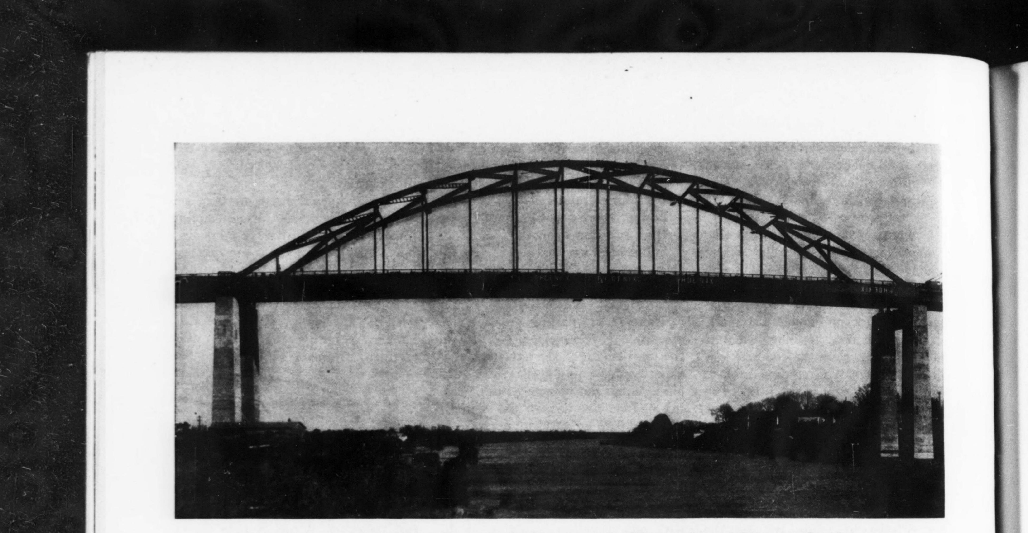
Fig. 1. A type of tied arch new to America spans the Chesapeake and Delaware Canal.
