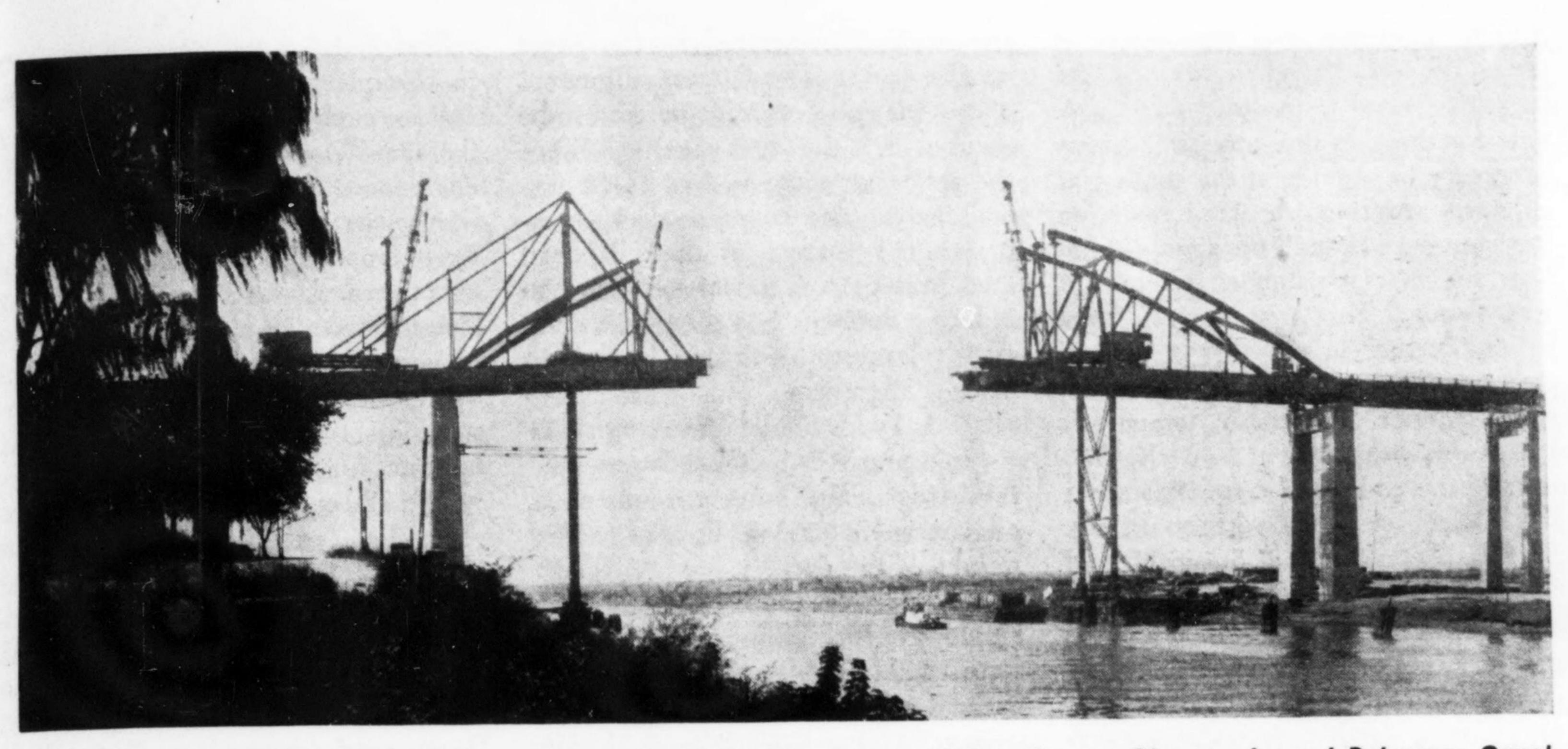
Fig. 1. Two variations of cantilever erection methods being used on tied arch over Chesapeake and Delaware Canal.
