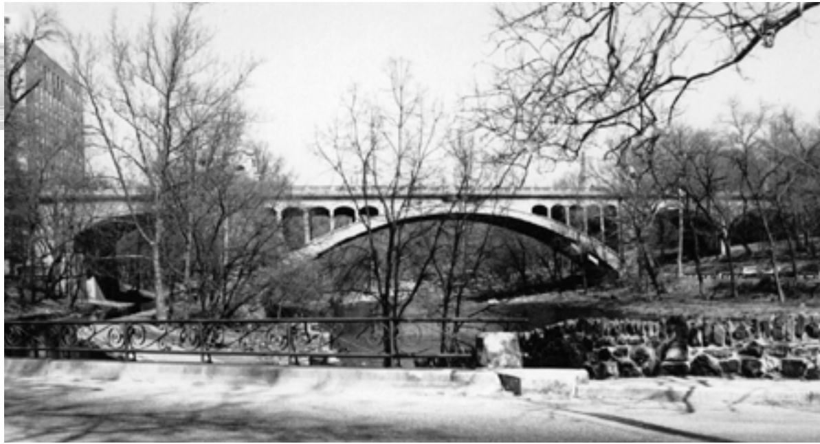
The Washington Street bridge (1920-21) is the only open spandrel arch bridge in Delaware. The high-level crossing of Brandywine Creek provided an ideal location to show the handsome open spandrel arch design.
