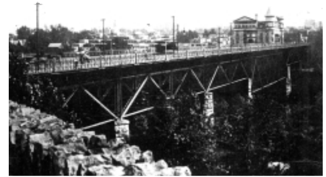
The Washington Street Bridge over Brandywine Creek in Wilmington was a deck truss bridge fabricated by the Edge Moor Bridge Works in 1893. The bridge served until 1921 when it was replaced by the present reinforced concrete open spandrel arch (State Bridge NC-576). Local residents and land developers objected to the truss bridge's narrow roadway.
