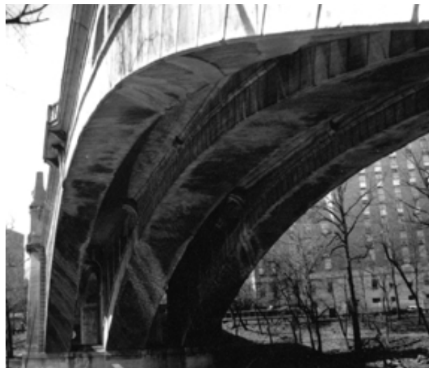
The view from below the Washington Street bridge.
