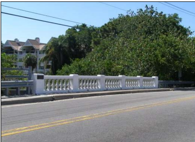
Photo 5-6. Osprey Avenue Bridge, Sarasota County (No. 175950)
