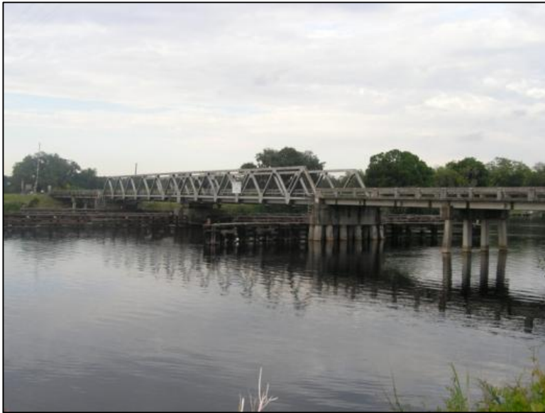
Photo 5-55. Ft. Denaud Swing Bridge, Hendry County (No. 070013)
