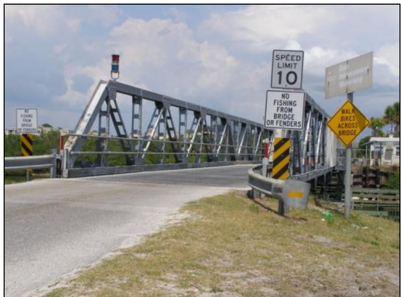
Photo 5-56. Blackburn Point Swing Bridge, Sarasota County (No. 170064)
