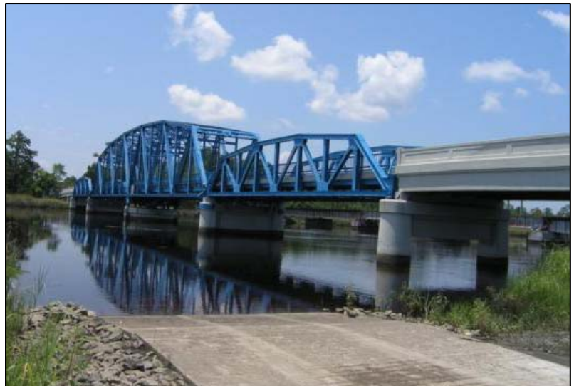
Photo 5-57. St. Mary's River Swing Bridge, Nassau County (No. 740008)
