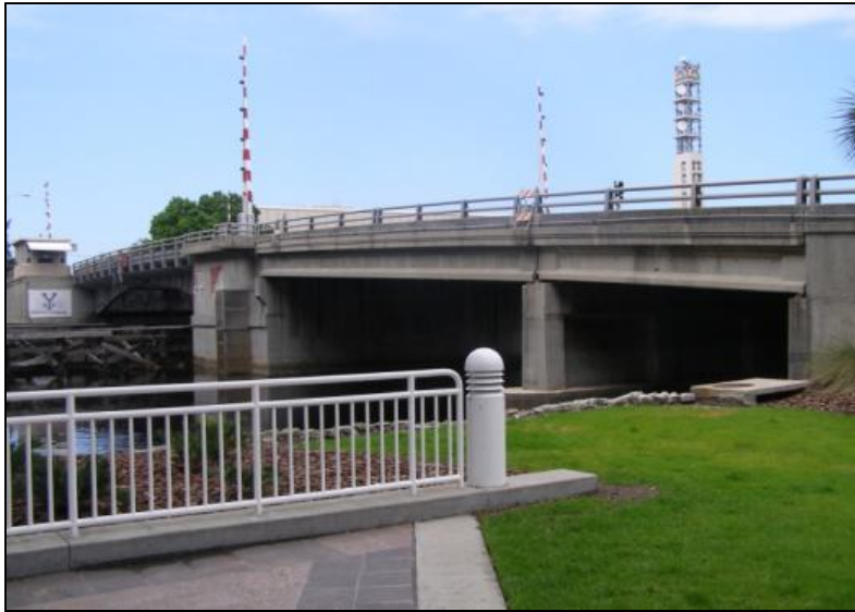
Photo 5-82. Brorein Street Bridge, Hillsborough County (No. 105501)
