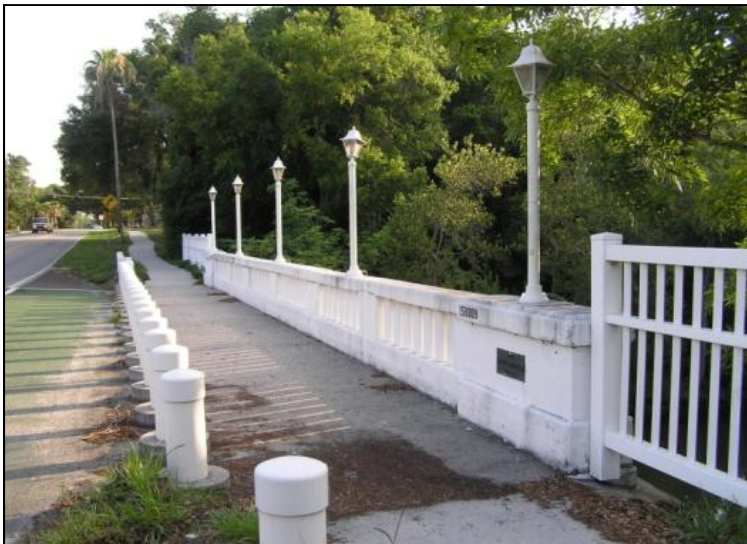
Photo 5-18. Philippe Parkway Bridge, Pinellas County (No. 150009)
