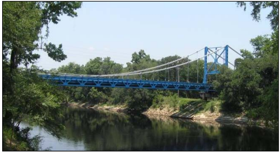
Photo 5-45. Hal Adams Bridge, Lafayette County (No. 330009)
