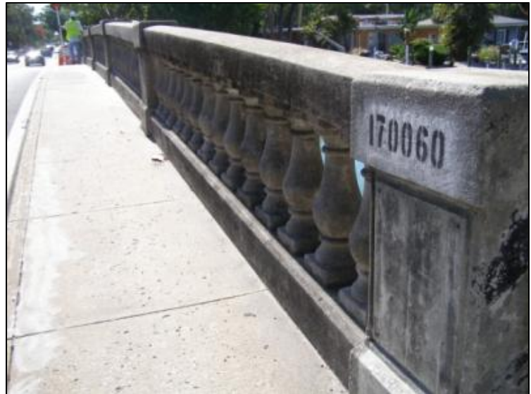
Photo 5-26. Hanson Bayou Bridge, Sarasota County (No. 170060)
