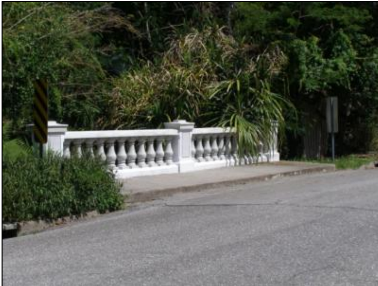
Photo 5-25. Whitaker Bayou Bridge, Sarasota County (No. 175660)
