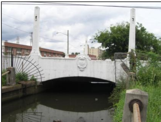
Photo 6-13. Market Street Bridge (No. 724172)
